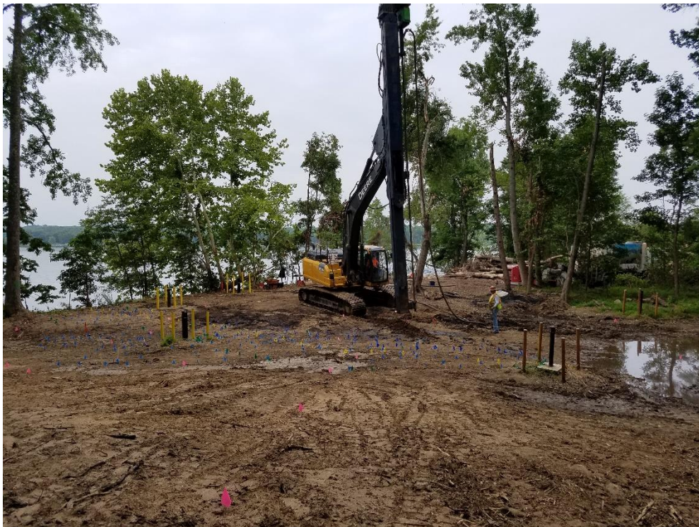
Field Demonstration: Grout Bomber column installation
