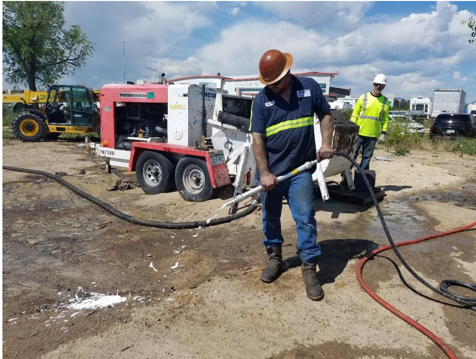
Amendment Pilot Test (Denver, CO): Organic Foam Additive
