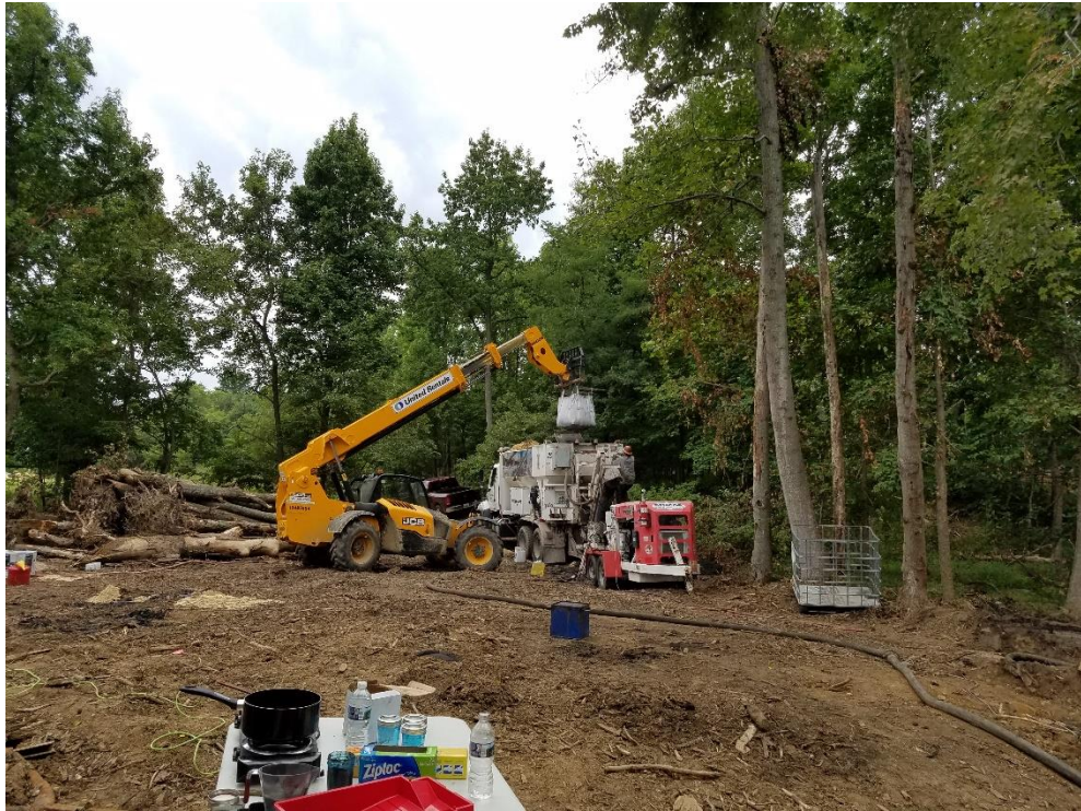
Field Demonstration, ZVI mixing in Elkin Mixer
