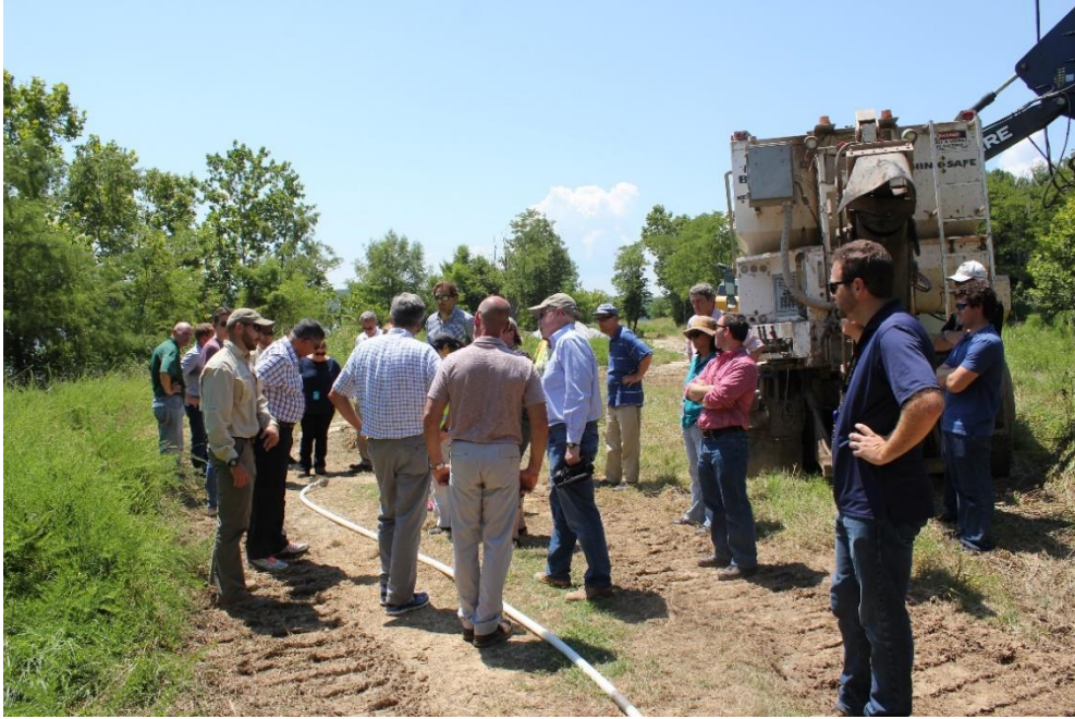
Field Demonstration of CMT construction using Grout Bomber (September 2017)
