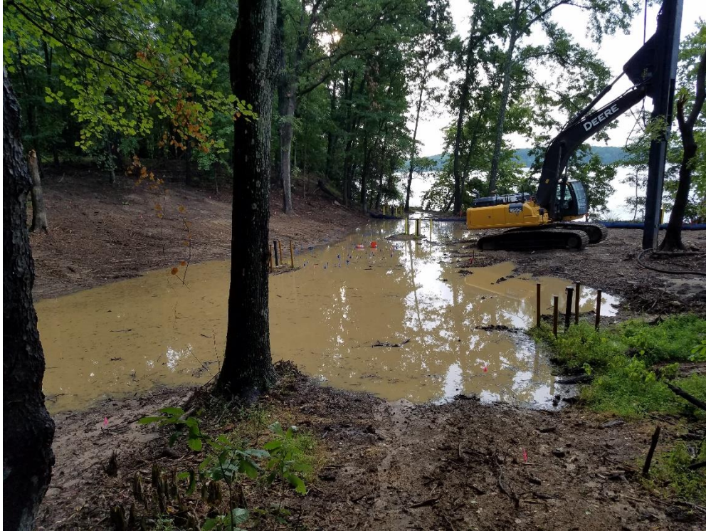
August 2017 Field Demonstration: After rain delay
