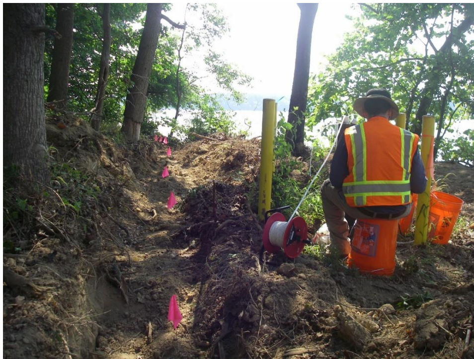
July 2017 GeoTrax LTM Electrode Installation (Facing North)
