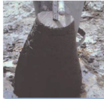
The grout mix must have specific characteristics: a very low mobility (low slump) mixture that is 'pumpable' but, upon installation, exhibits an internal friction enabling it to remain intact and displace the surrounding soil without fracturing it.
