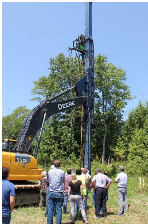
Grout Bomber Field Demonstration: South Plume Storage and Preparation Area
