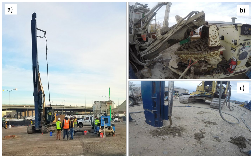
Figure 2.1. a) Grout Bomber Equipment Set Up; b) Hopper for Mixing and Delivery of Grout to the Stitcher; and c) Grout Exiting the Mandrel.
