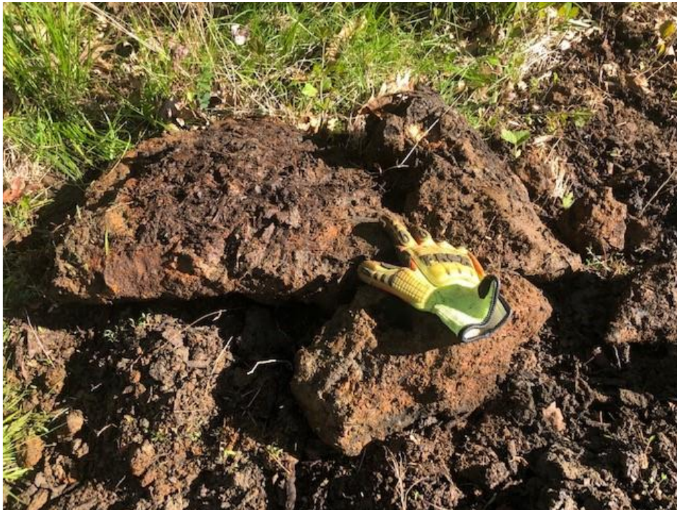
Chunks of ZVI material from “dogpiles” excavated during April 2019 SVP installation
