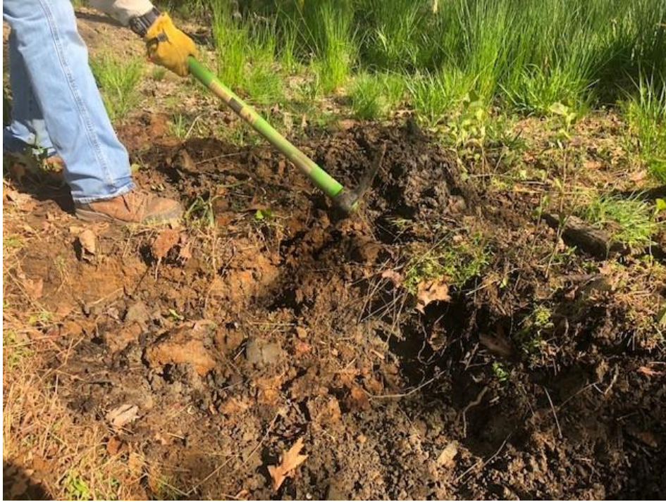
April 2019 Performance Monitoring and SVP Installation
