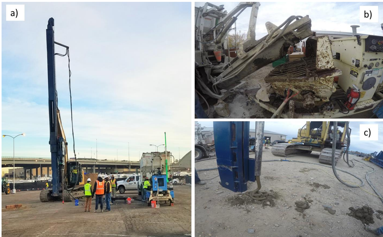
Figure C.1. a) Grout Bomber arrangement, includes excavator with grout delivery implements and onsite cement mixer, pumps, and power supply; b) example of concrete mixing truck unloading into hopper for mixing and delivery to rig; and c) exit end of grout bomber, shows concrete grout used in geotechnical applications being pumped through mandrel.
