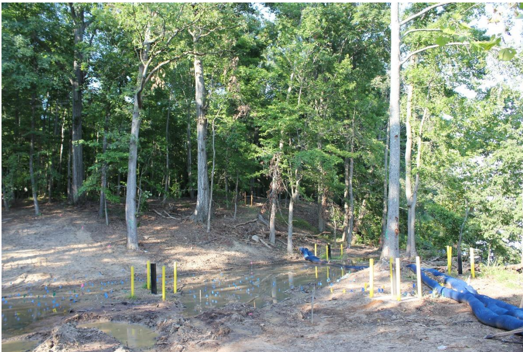
August 2017 Field Demonstration (Facing North)
