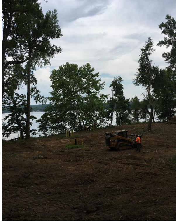
Field Demonstration: After Site Clearance (Facing South)
