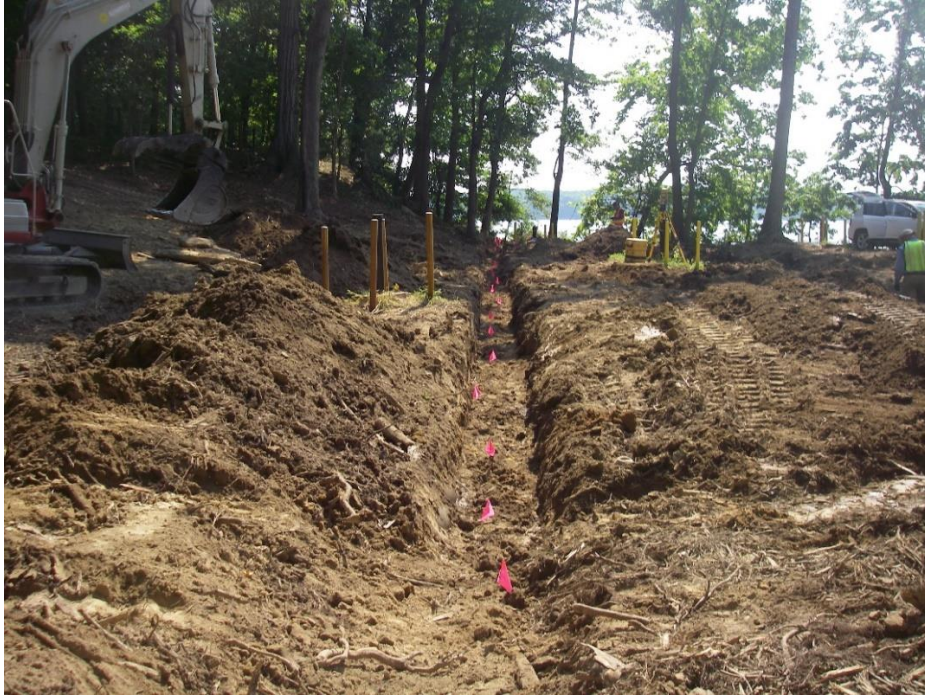
July 2017 GeoTrax LTM Electrode Installation (Facing South)
