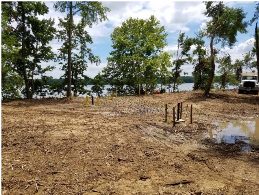
Field Demonstration: After Site Clearance (Facing South); Column Locations Marked in Preparation for Installation (blue flags)
