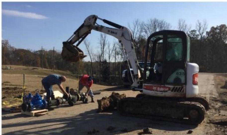
Figure B-2. Singer Valve Installation
