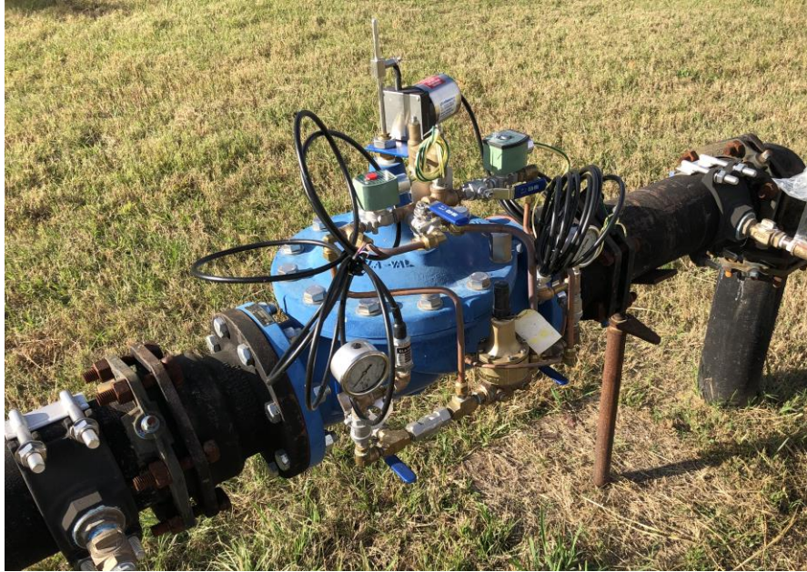
Figure 4-1. Conversion Kit Installed on Cla-Val 131
