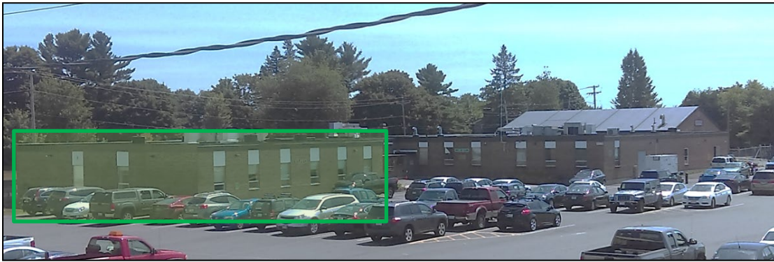
Figure 1. Building 39 at MEARNG Camp Keyes which Was the Primary Demonstration Site.
