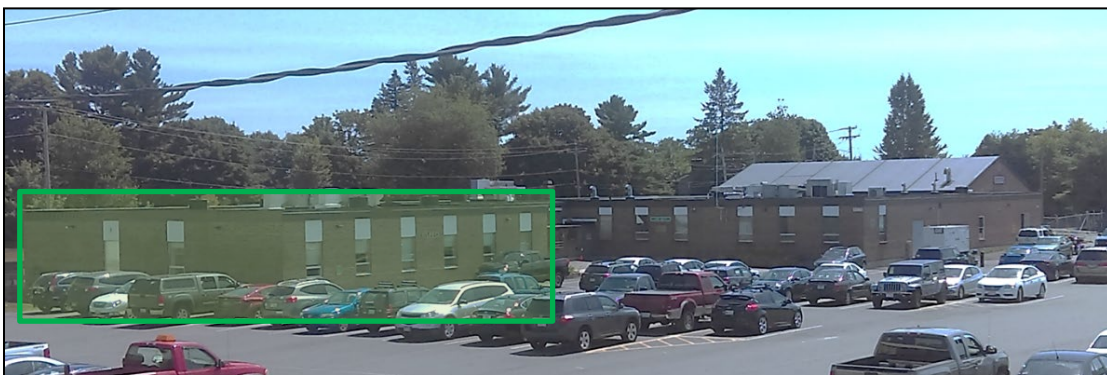
Figure 12. Building 39 at MEARNG Camp Keyes Which Was the Primary Demonstration Site.
