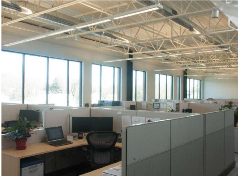
Figure 41. Highly Daylit Space with Photocontrolled Lighting System.
