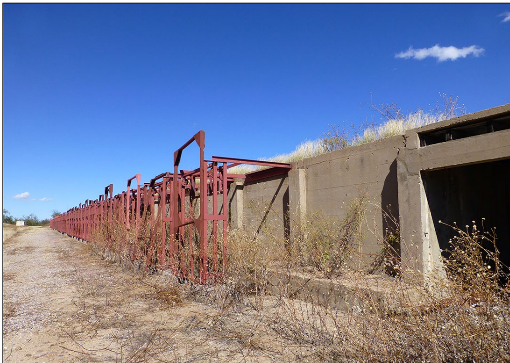
Figure 190. View north along target butt of Range 6 with metal target frames (ID #28) (ERDC-CERL 2016).
