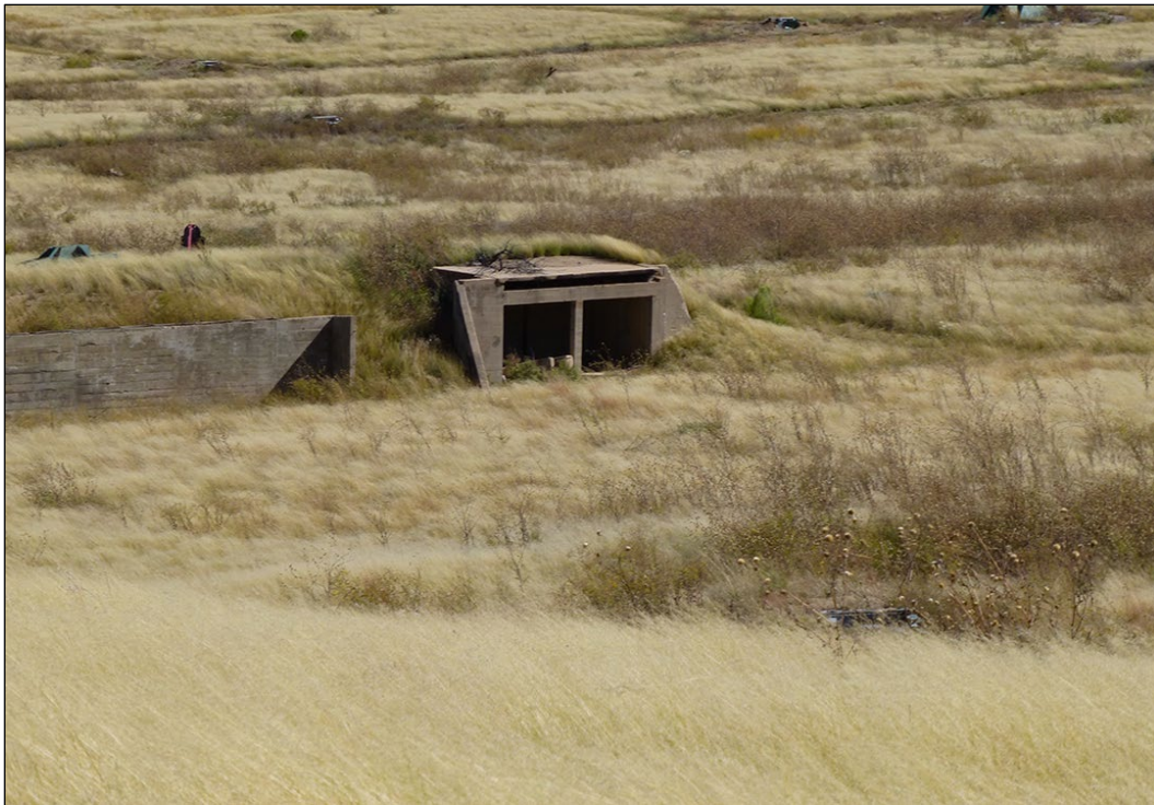
Figure 195. View to the southeast of storage area ( left ) and target storage ( right ) at Range 9 (ID #28) (ERDC-CERL 2016).
