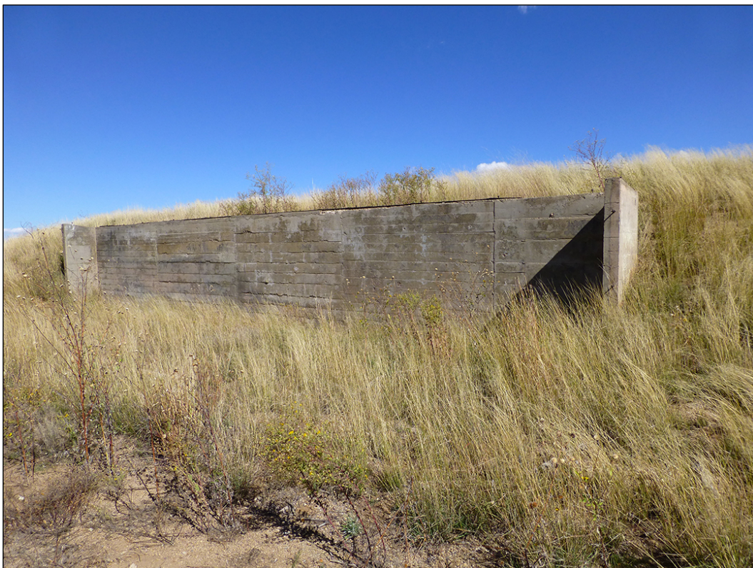
Figure 196. View to the east of storage area at Range 9 (ID #28) (1983) (ERDC-CERL 2016).
