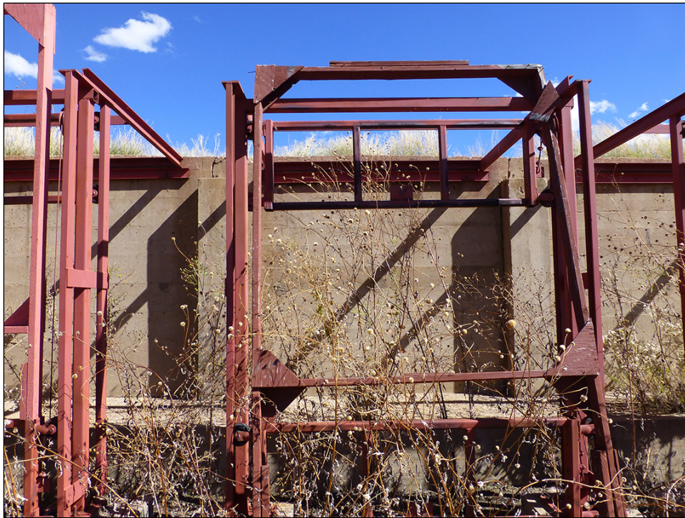
Figure 191. View to the east of a detail of target holders on target butt on Range 6 (ID #28) (ERDC-CERL 2016).
