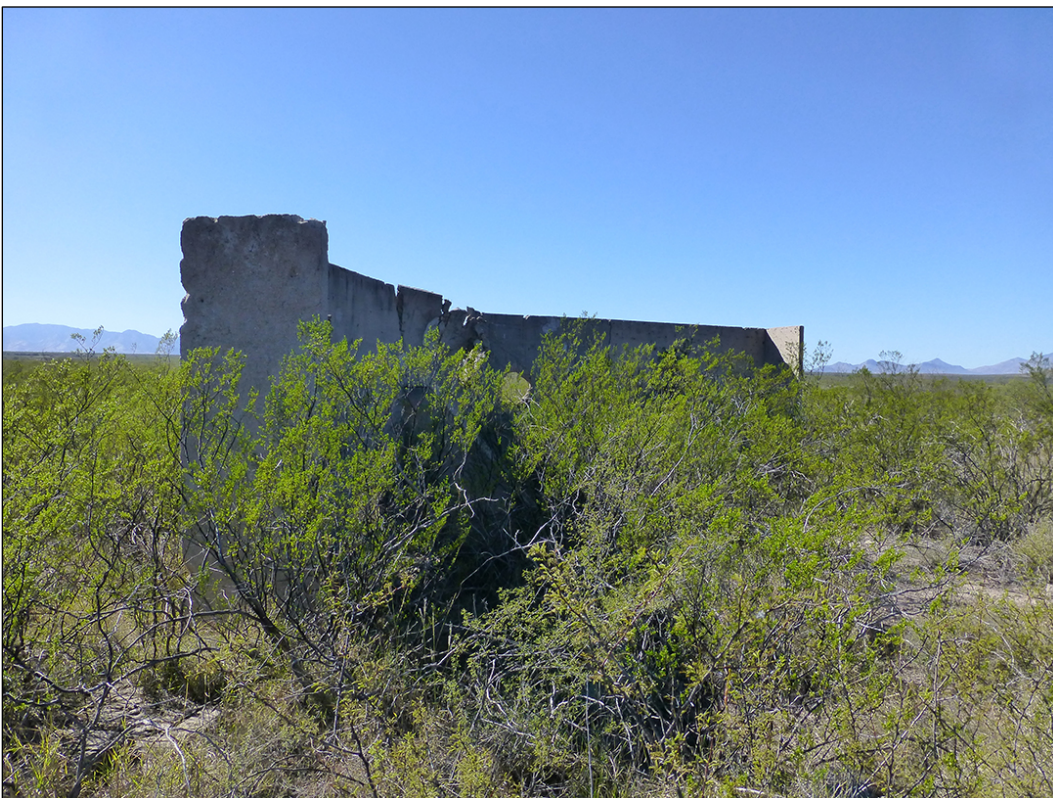
Figure 229. Remnants of concrete range targets looking west (ID #19) (ERDC-CERL 2016).
