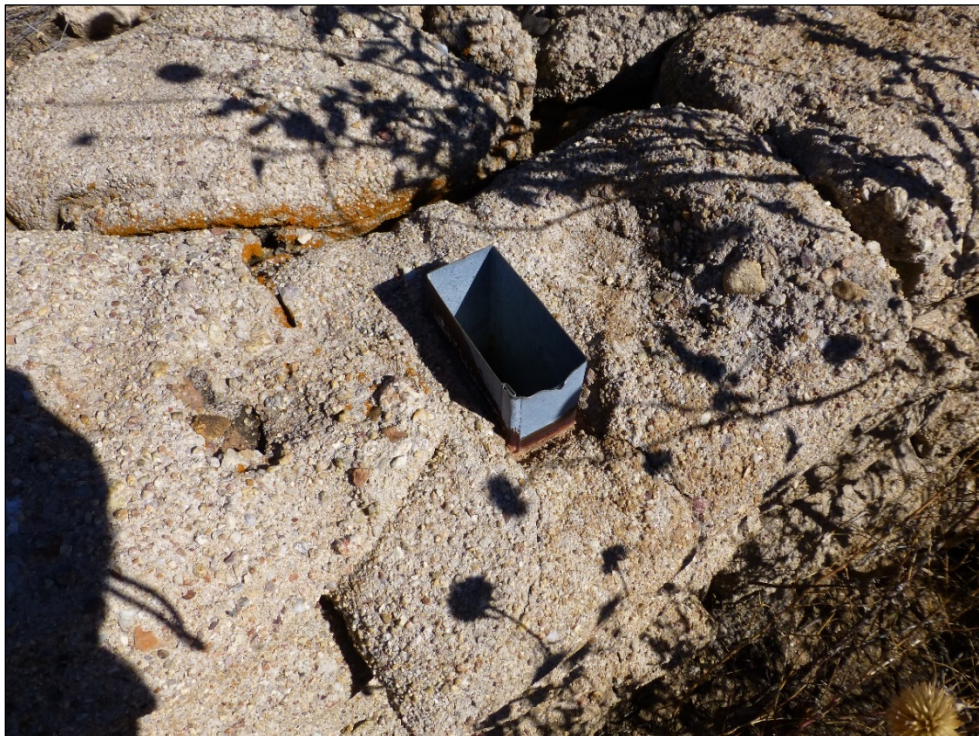
Figure 159. Looking down at remnants of concrete sandbag target bunker and target stand (ID #1) (ERDC-CERL 2016).
