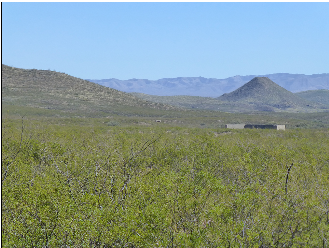
Figure 227. Remnants of concrete range targets looking east (ID #19) (ERDC-CERL 2016).
