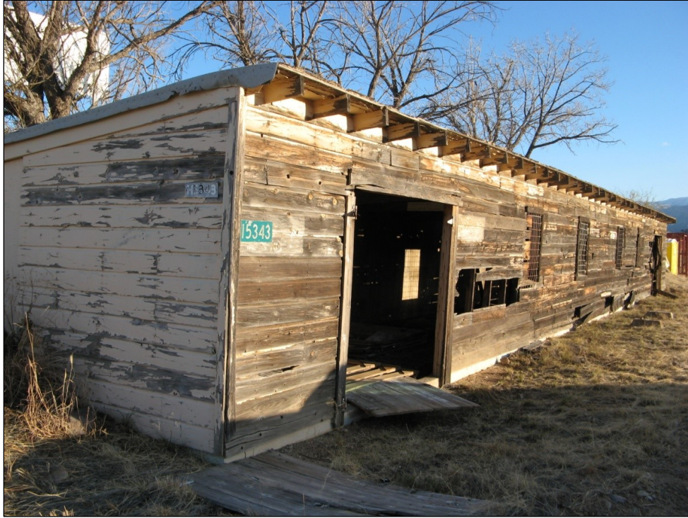
Figure 181. View to the southeast of last remaining wooden storage building at the north end of the target butt at Range 6 (Facility #15343) (ID #28) before it burned down in 2013 (Chattey and Abraham 1998. Public Domain).
