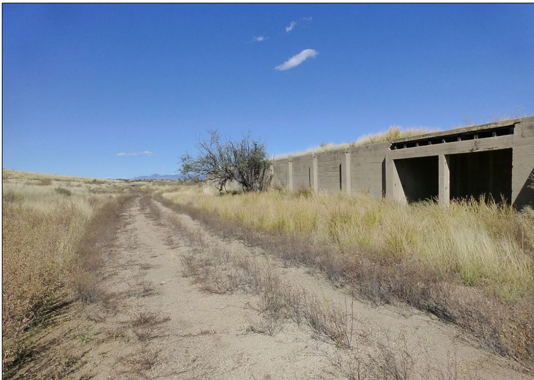
Figure 186. View north along target butt of Range 8 (ID #28) (ERDC-CERL 2016).
