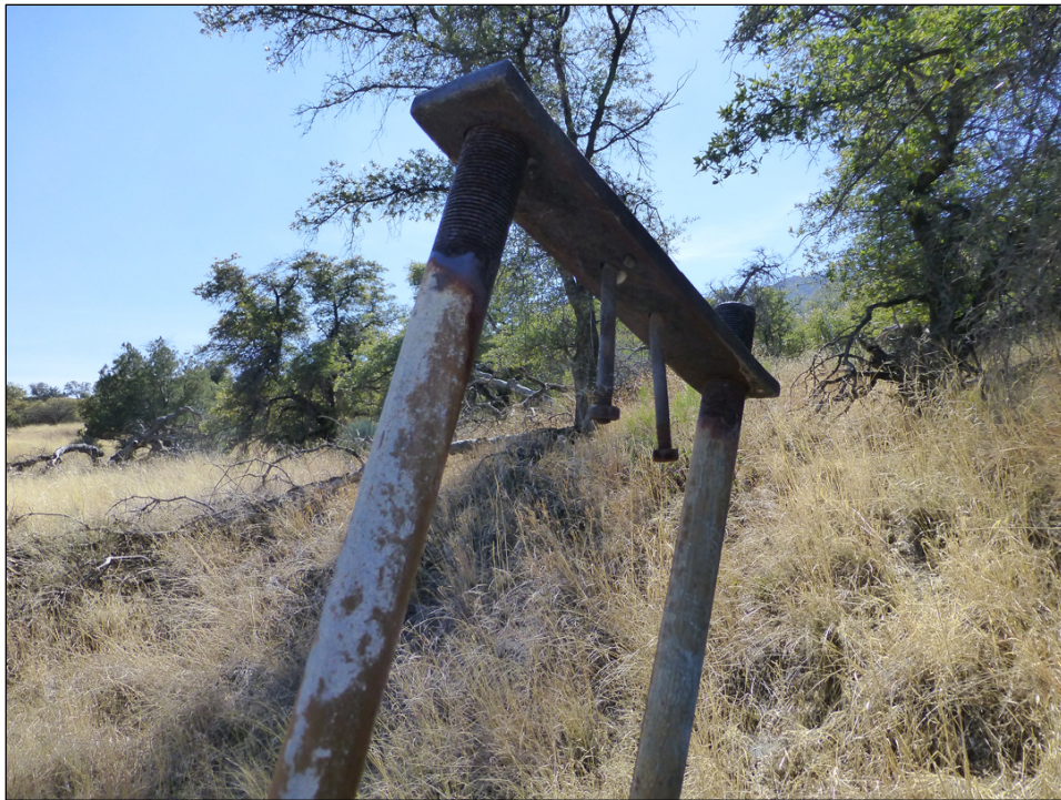
Figure 165. View looking south at old target stand at WWI firing range (ID #24) (ERDC-CERL 2016).
