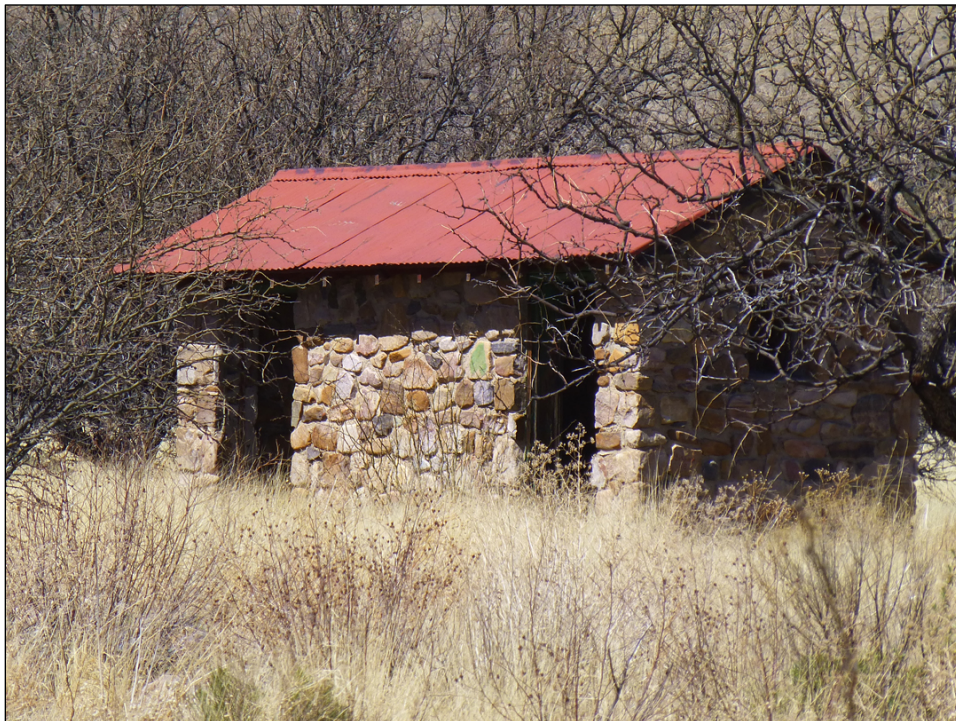
Figure 176. View looking northwest at stone latrine building (Facility #15331) north of the Known Distance Range (ID #25) (ERDC-CERL 2016).
