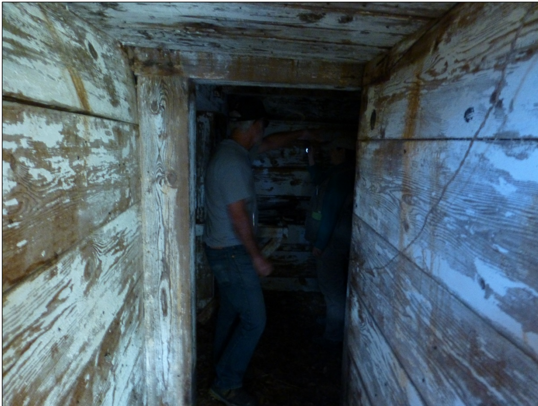
Figure 204. Looking northeast at the interior through entryway of wood-walled communication bunker (ID #6) (ERDC-CERL 2016).
