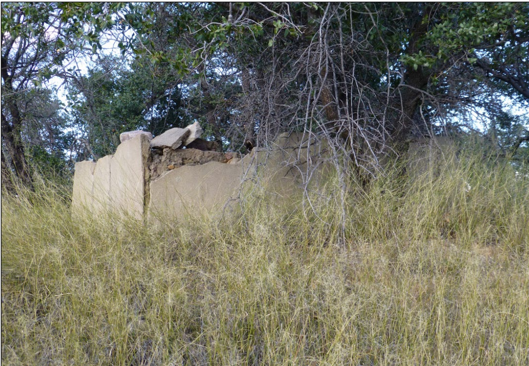
Figure 147. Looking southeast at WWII concrete structures (ID #15) (ERDC-CERL 2016).
