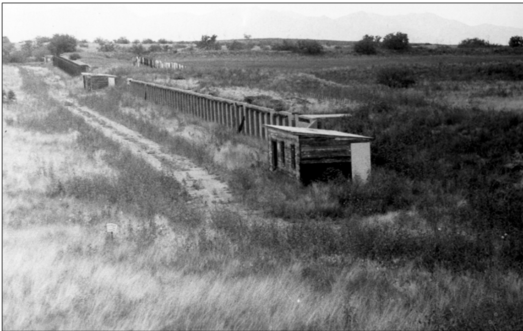
Figure 93. Building #15339 ( foreground ), target butt, Building #15335 ( middle ), and Building #15343 ( background ), 1998 (AZ- -1, Box 15, Fort Huachuca DPW. Public Domain).
