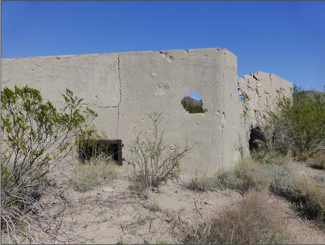
Figure 230. Remnants of concrete range targets looking east (ID #19) (ERDC-CERL 2016).
