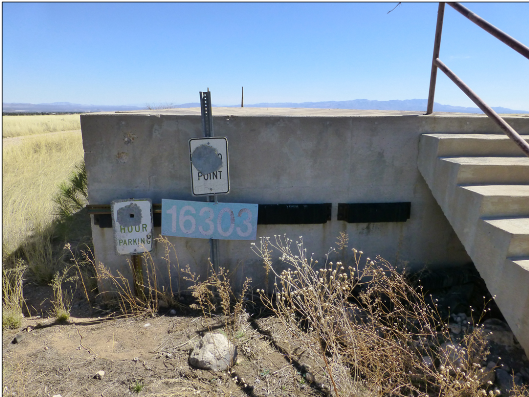
Figure 213. Concrete stairs and platform facility sign (Facility #16303) (ID #29) (ERDC-CERL 2016).
