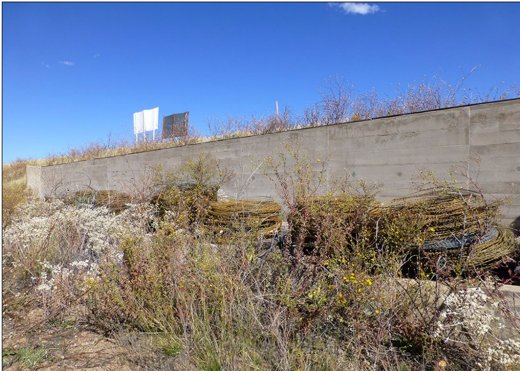
Figure 188. View to the northeast of storage area at Range 8 (ID #28) (ERDC-CERL 2016).
