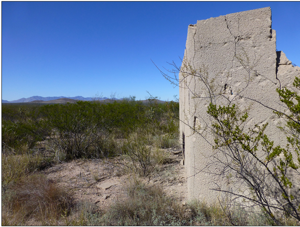
Figure 232. Remnants of concrete range targets looking northwest (ID #19) (ERDC-CERL 2016).
