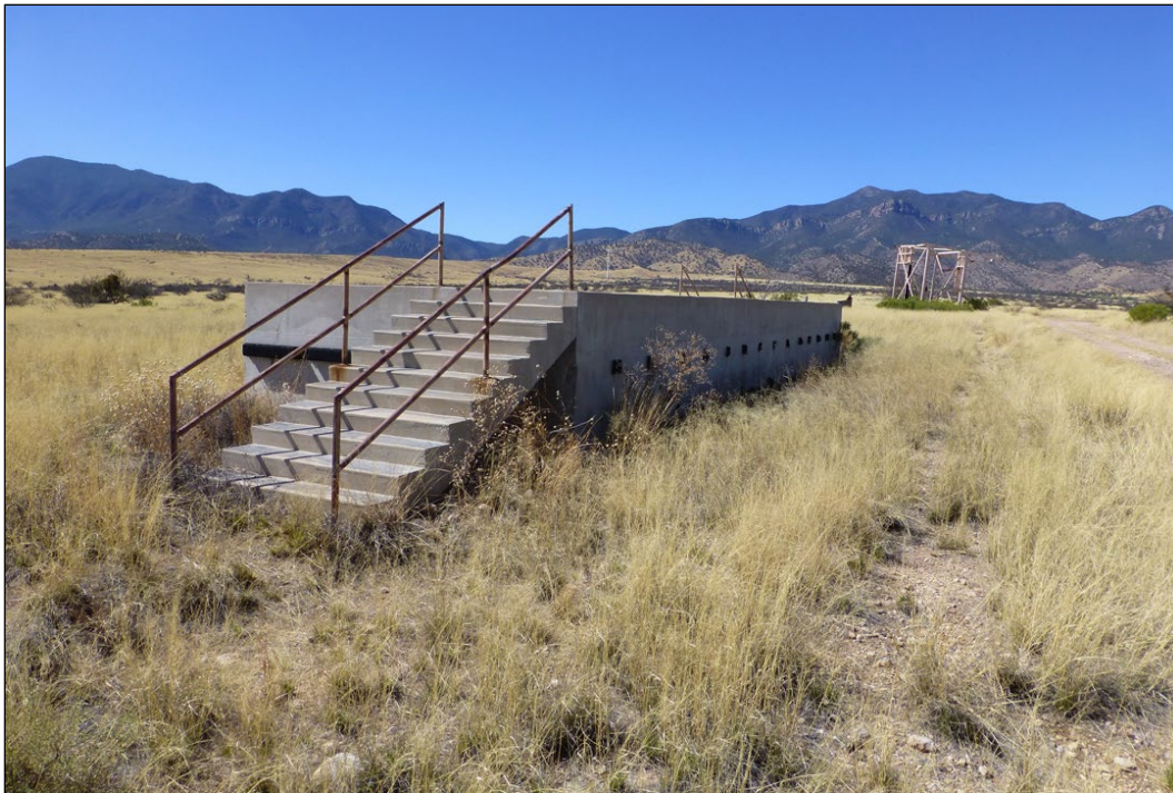
Figure 212. View to the west of concrete stairs and platform (Facility #16303) (ID #29) (ERDC-CERL 2016).
