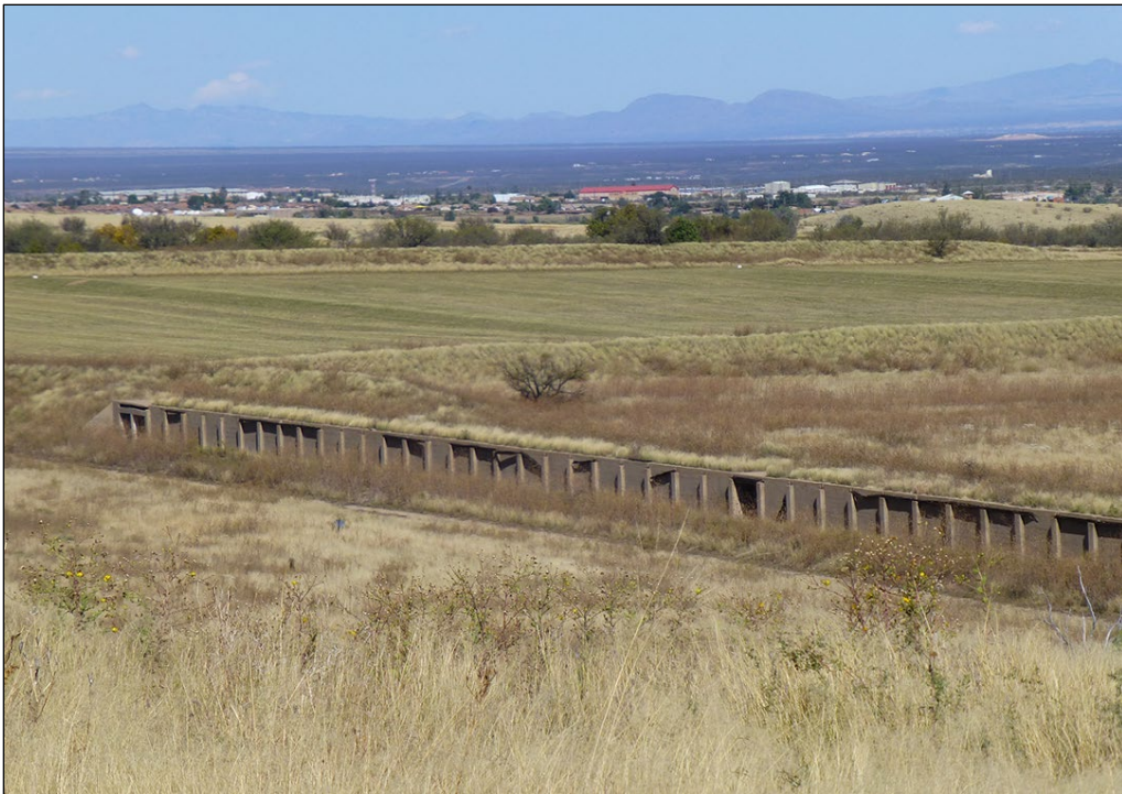
Figure 183. Looking to the northeast over the concrete target butt of Range 8 (ID #28) (ERDC-CERL 2016).
