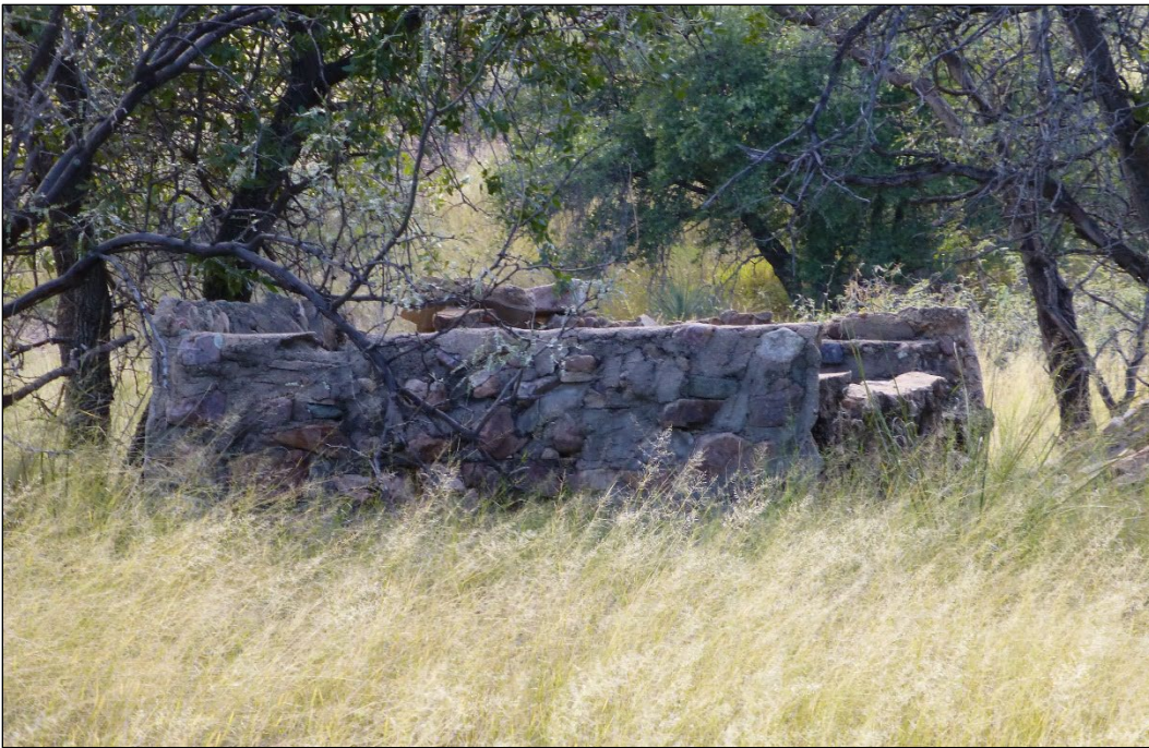
Figure 148. View to the south-southeast of stone structures (ID #15) north of Demonstration Hill (ERDC-CERL 2016).
