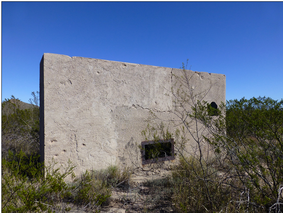
Figure 233. Remnants of concrete range targets looking east (ID #19) (ERDC-CERL 2016).
