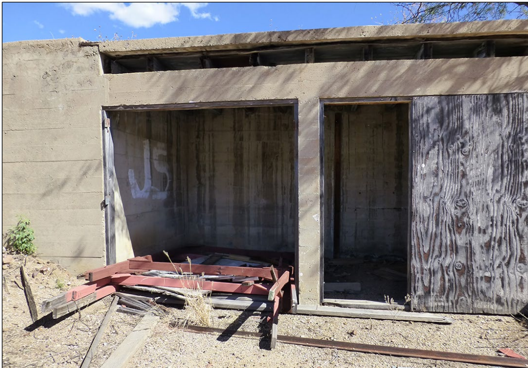
Figure 193. View of target storage area at north end of target on Range 6 (ID #28) (ERDC-CERL 2016).
