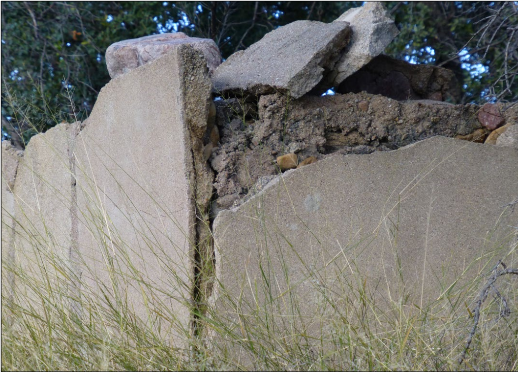
Figure 146. Looking southeast at corner detail of WWII concrete structures (ID #15) (ERDC-CERL 2016. Public Domain).
