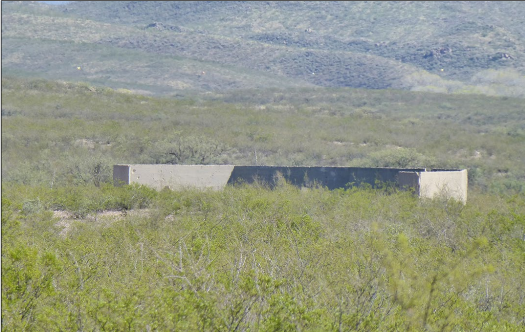
Figure 228. Remnants of concrete range targets looking east (ID #19) (ERDC-CERL 2016).
