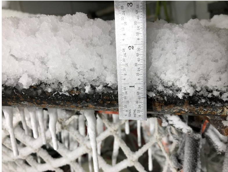
Figure 14. Small engineer scale measurement.
