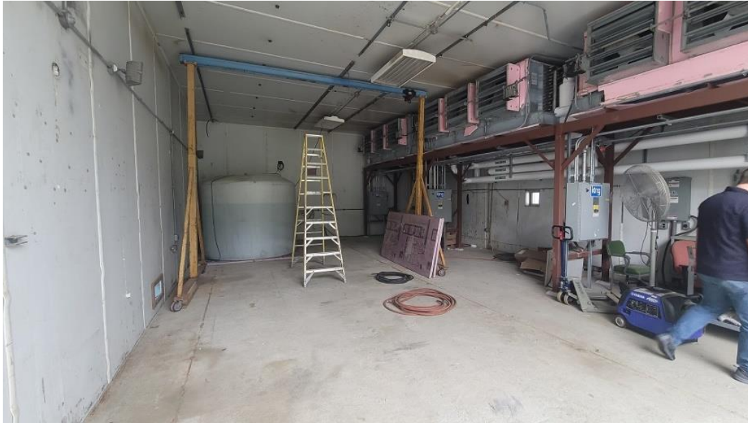
Figure 5. Interior view, CRREL Materiel Evaluation Facility.
