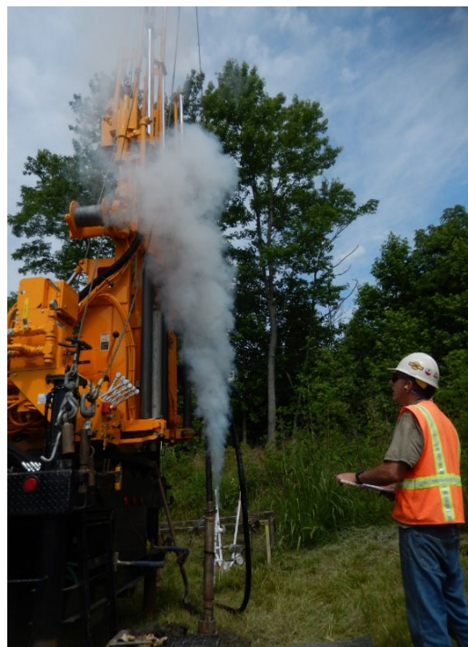
Figure 2.2. Liquid nitrogen injection and vending during the freezing process.
