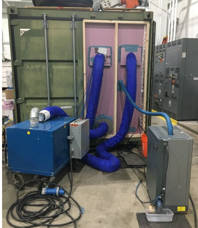
Figure C-7. 250K heater (left) and steam generator (right) used for Trial 3
