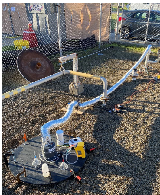
Figure 51. Flexible duct connected from Hatch C (upper right corner) to air recirculation blower to GDU
