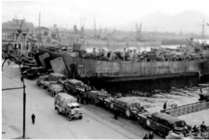
Figure 4. Preloaded Supply Trucks and DUKWs at Naples. Center of Military History Publication 72-19, Anzio , (Center of Military History), 11.
