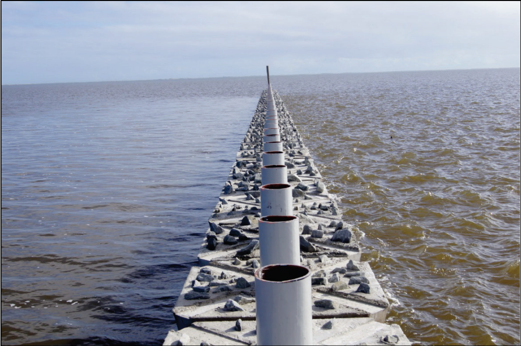
Figure 1. Section of Ecosystem Wave Attenuator installed on sound side of the Outer Banks.
