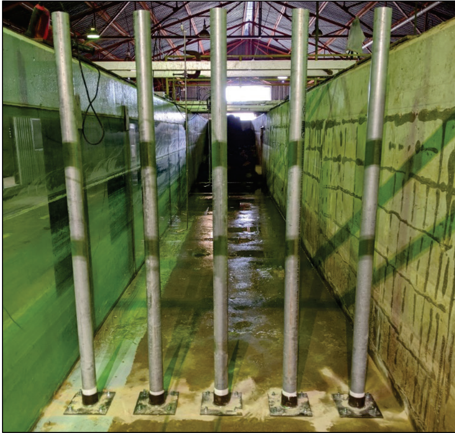
Figure 6. Mounting plates and pipe installation in flume.
