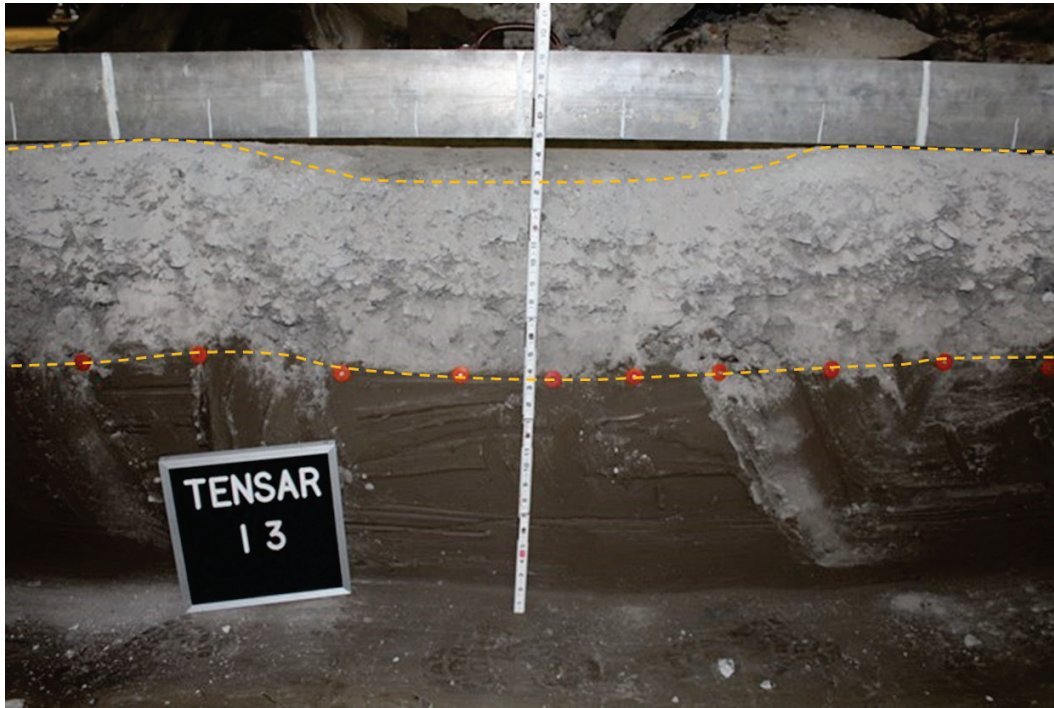
Figure 43. Item 3 (unstabilized) posttest excavation.
