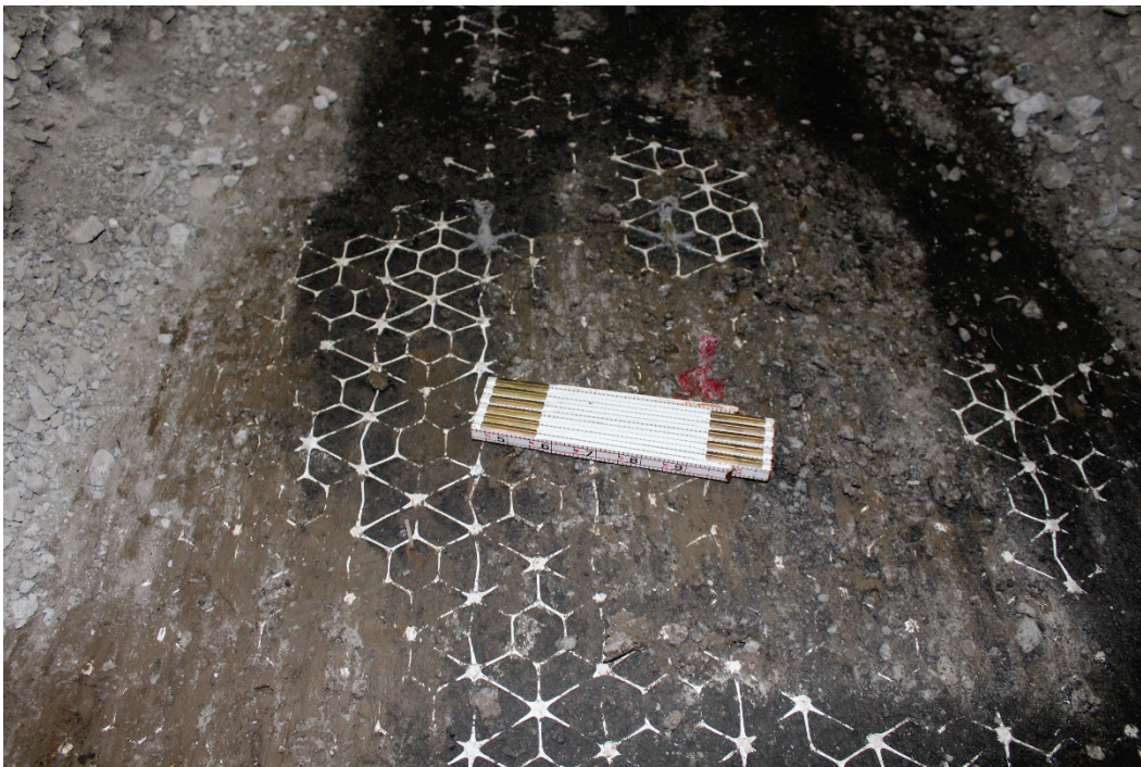
Figure 39. Item 2 (NX750) excavated geogrid.
