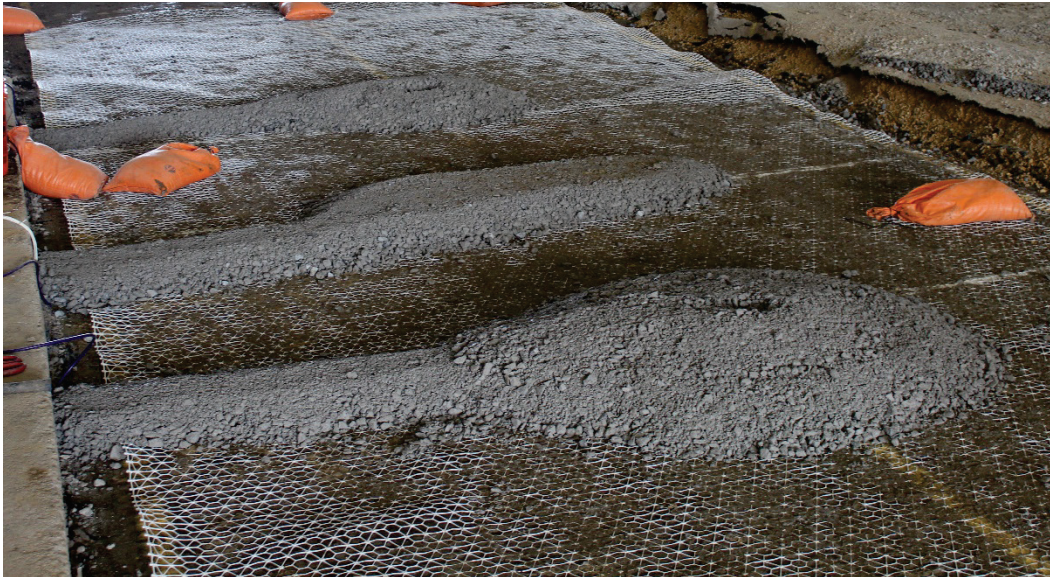
Figure 11. Base EPC installation prior to base aggregate placement.
