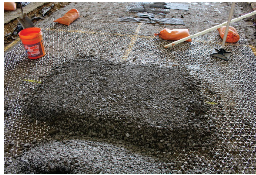
(c) Completed installation.
