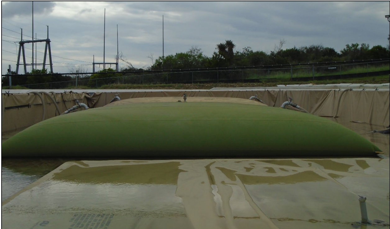
Figure H-4. SEI JK #8 CFT Filled with Fuel (Puddles are from Recent Rains, not Fuel)
