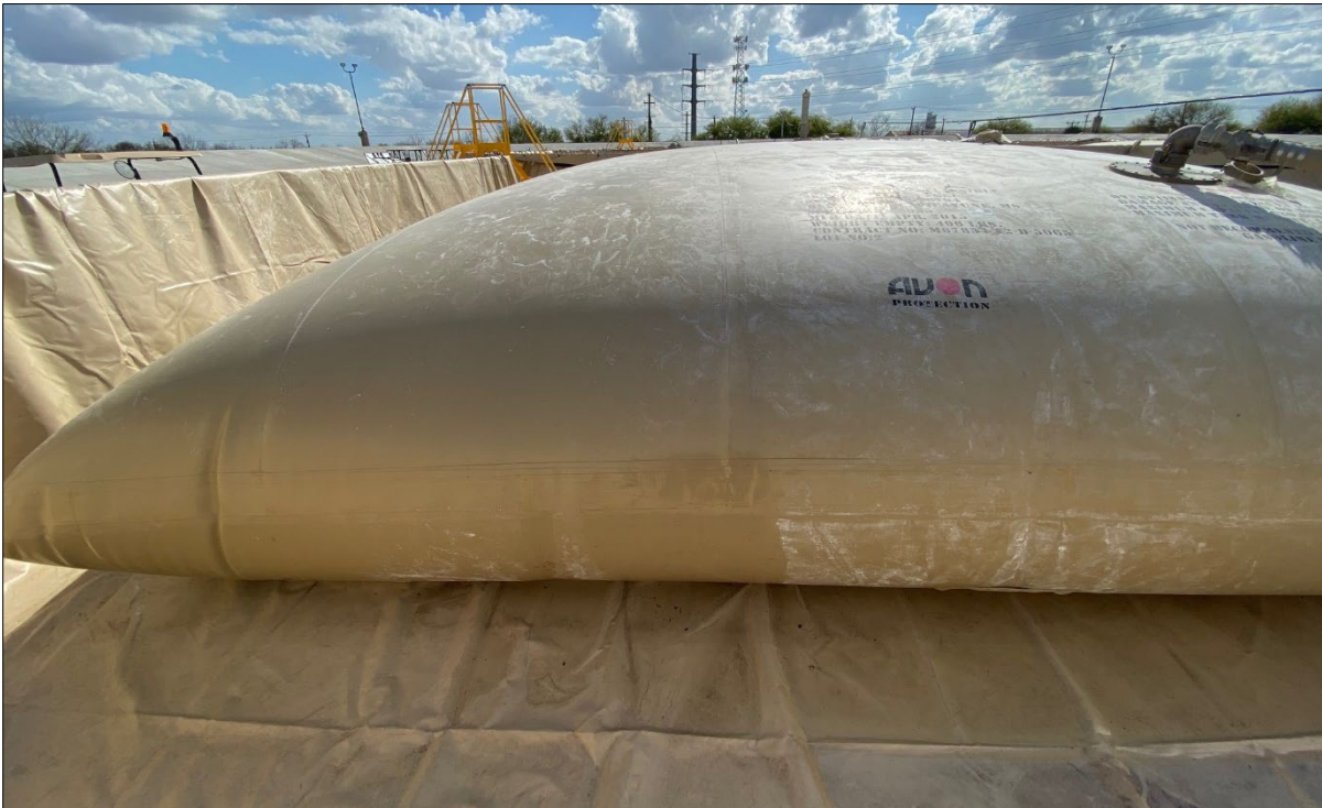
Figure D-4. MILPAWS #4 CFT Fuel Seeping from Seam
