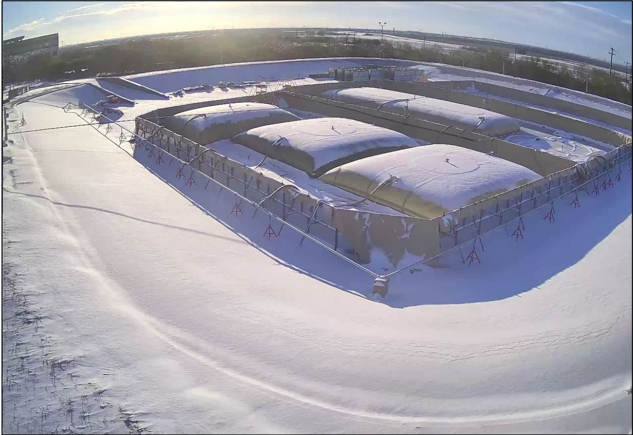
Figure 1. SwRI CFT Facility on February 15, 2021 During Winter Storm Uri
