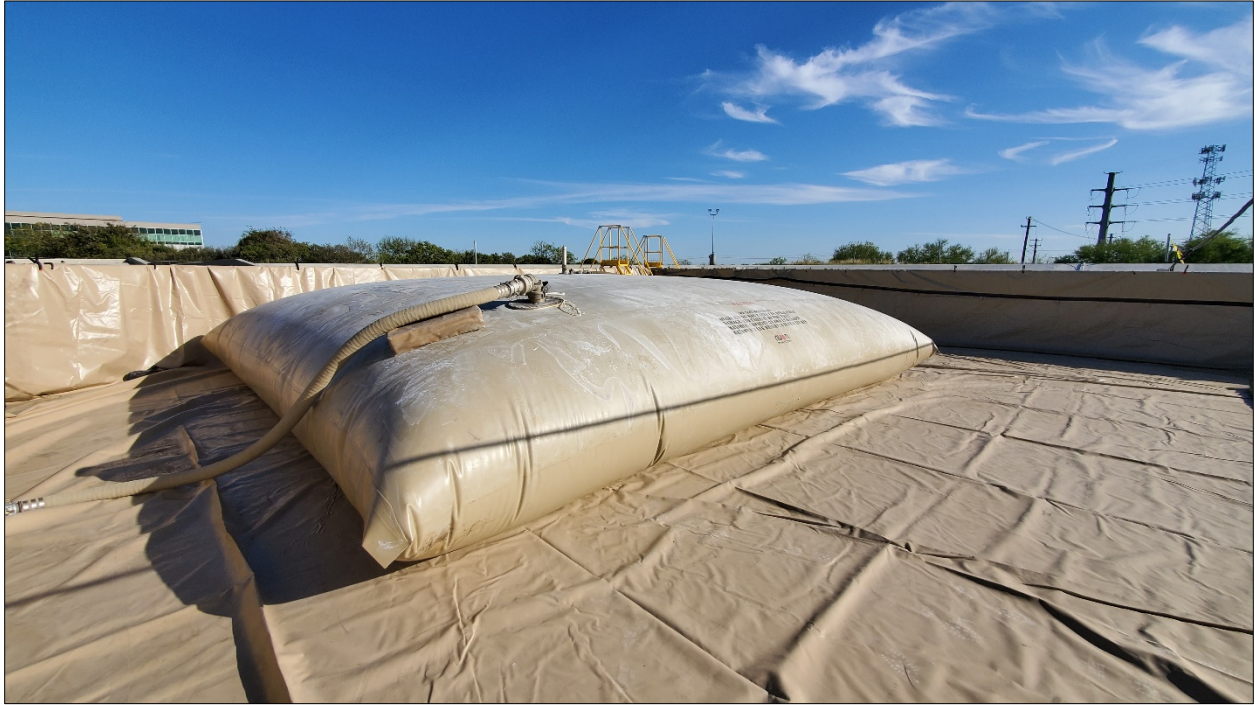
Figure C-4. AEF #3 CFT Filled with Fuel
