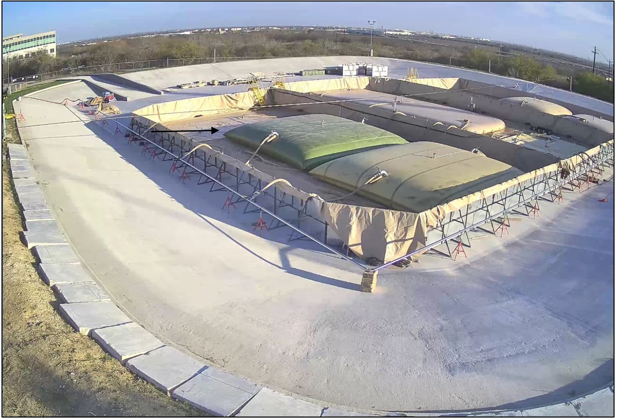
Figure H-5. Location of SEI JK #8 CFT at SwRI CFT Facility
