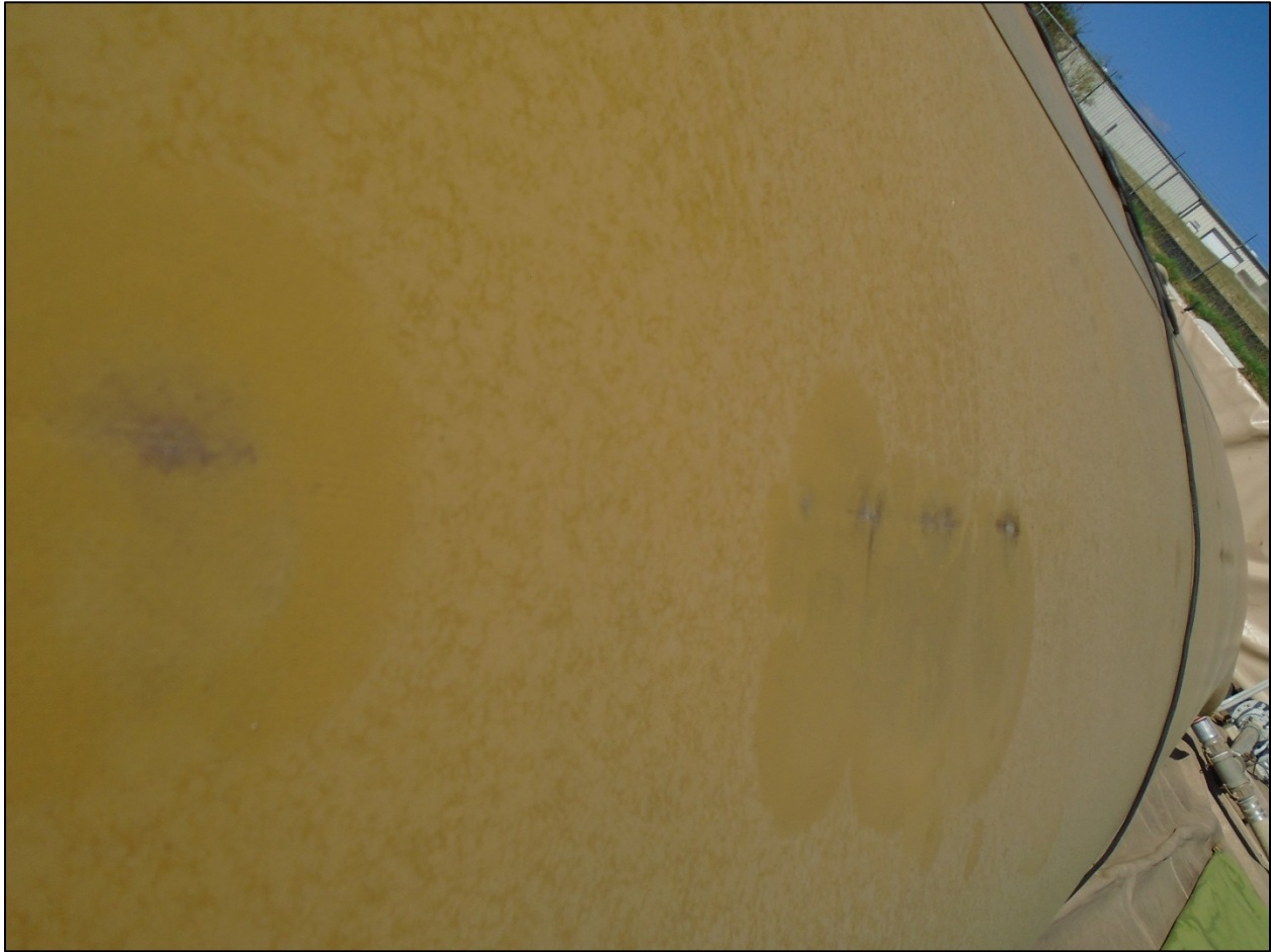
Figure I-6. SEI DK #9 CFT Showing Fuel Staining Through Fabric, October 2021
