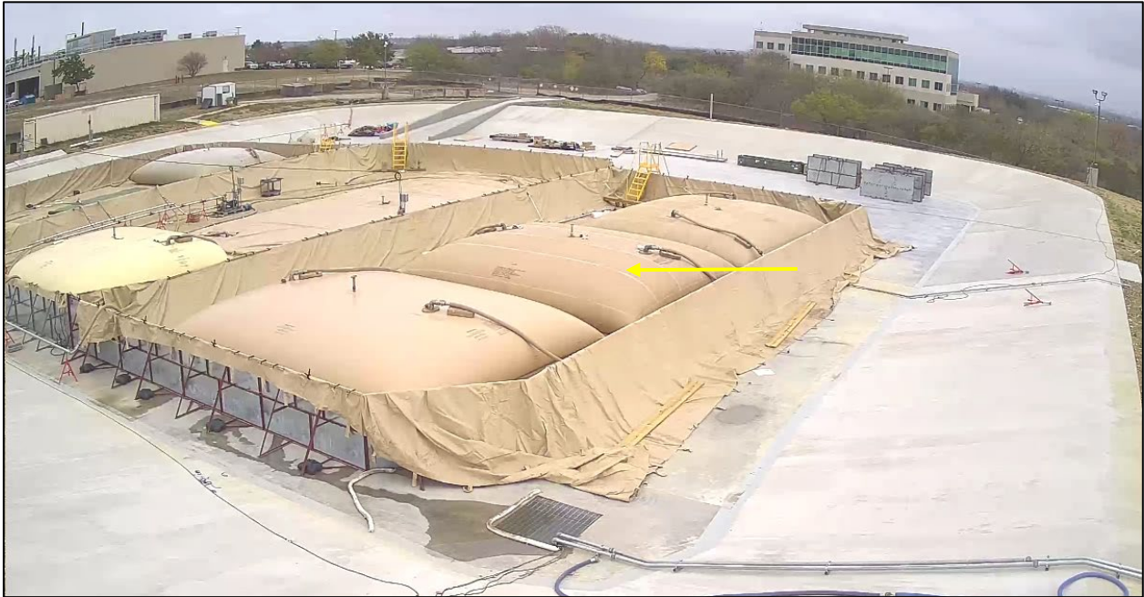
Figure B-5. Location of JGB #2 NITRILE CFT at SwRI CFT Facility
