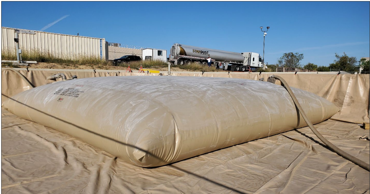
Figure C-3. AEF #3 CFT Filled with Fuel
