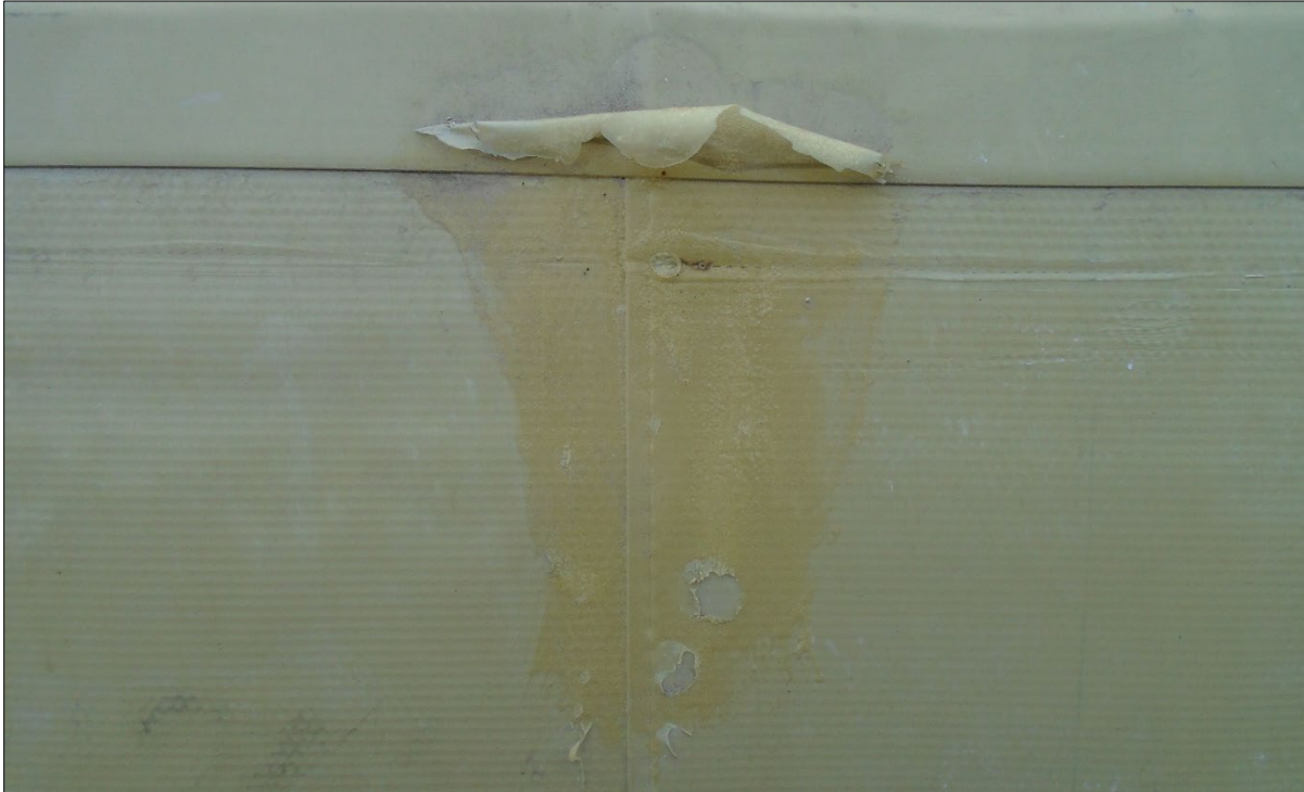
Figure D-5. MILPAWS #4 CFT Surface Blistering
