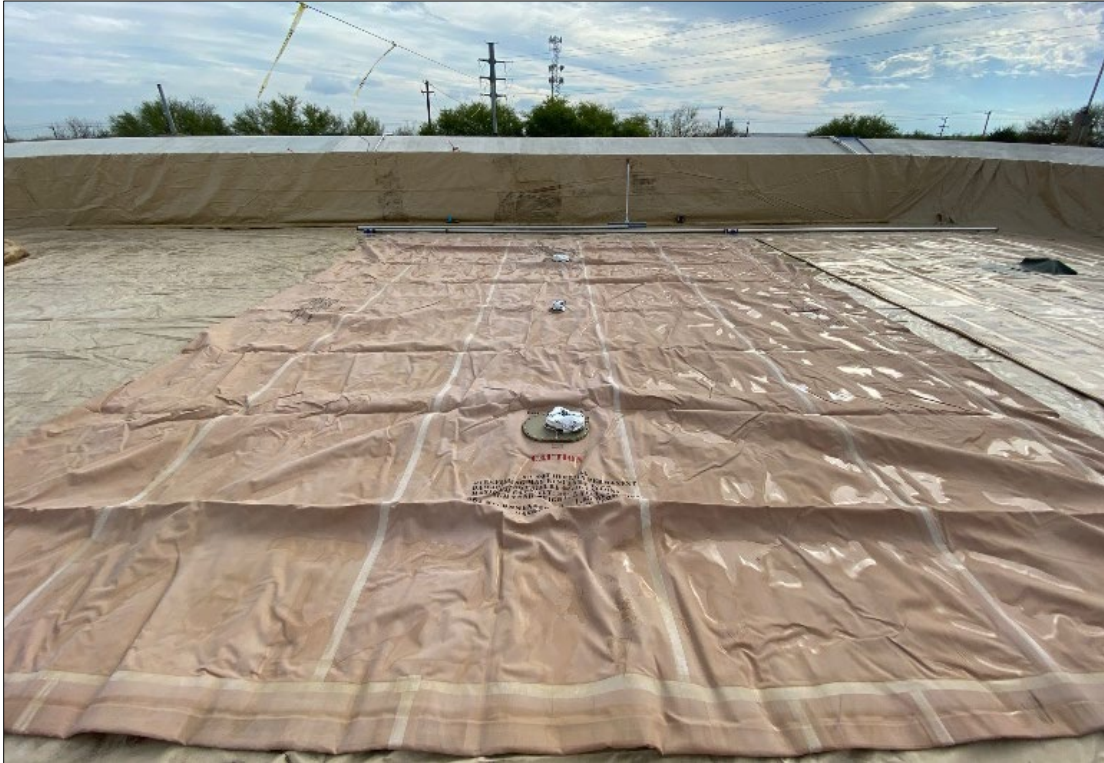
Figure B-1. JGB #2 NITRILE CFT Unfolded and Deployed (Looking South)
