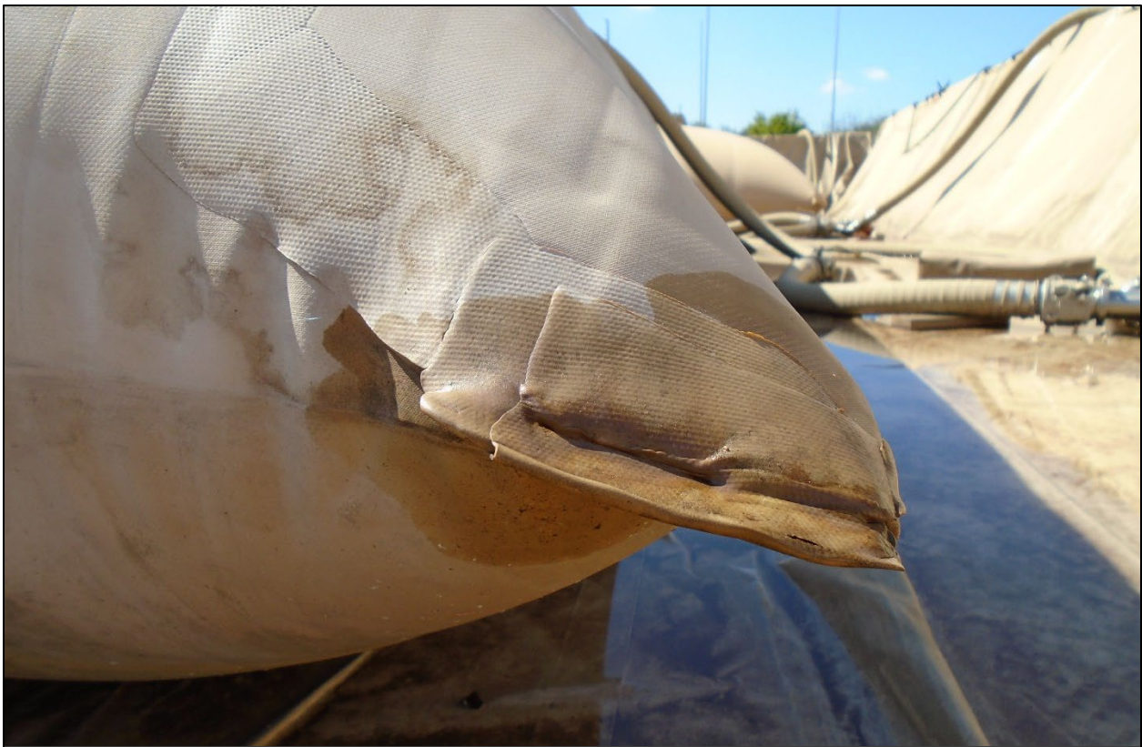
Figure B-6. JGB #2 NITRILE CFT Corner Fuel Wetting (Puddles are from Recent Rains, not Fuel)
