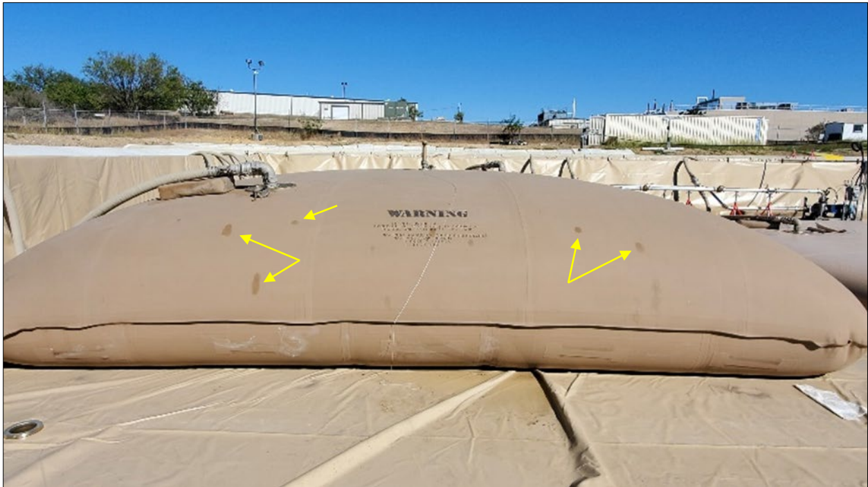
Figure A-2. BLSS #1 (NAFT #1) Filled with Fuel; Evidence of Leaks Through Fabric
