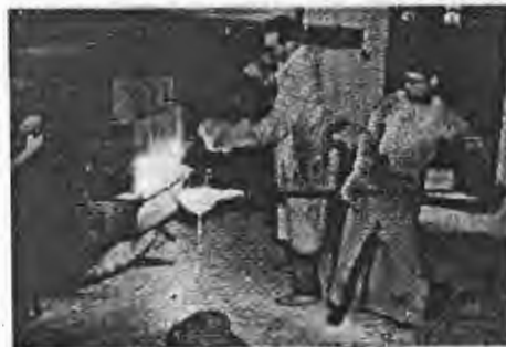
FIG. 2-STIRRING THE ALUMINUM INTO THE SPOON SAMPLE.
