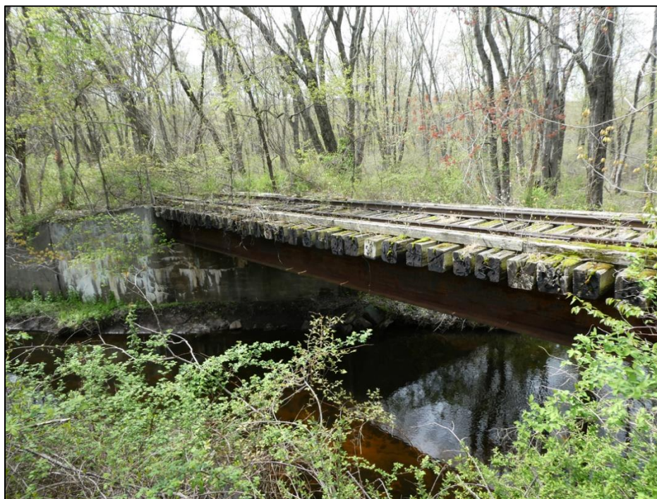
Figure 59. Bridge over Green Pond Creek.
