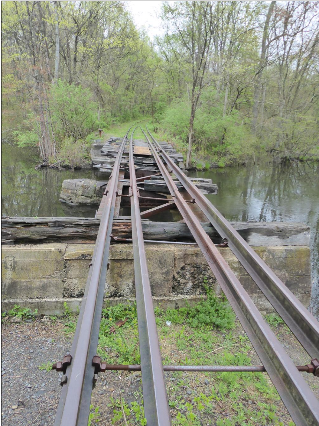
Figure 50. Looking east across the Rockaway River bridge.
