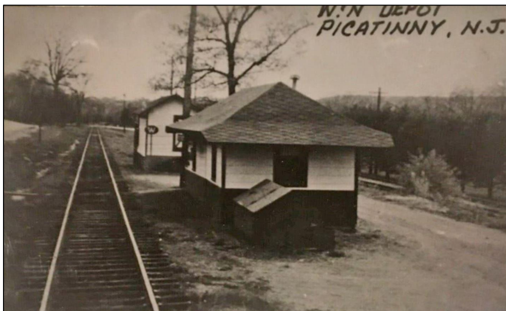
Figure 27. Wharton & Northern Depot at Picatinny Arsenal, no date.
