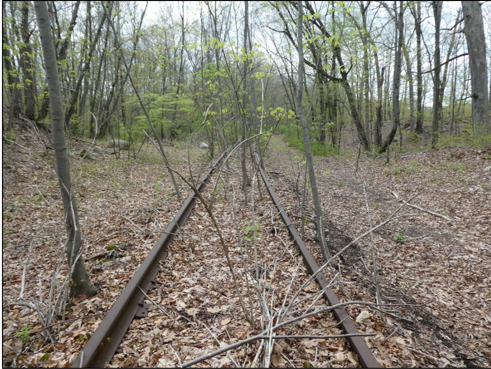
Figure 52. Looking west on the Wharton & Northern ROW.
