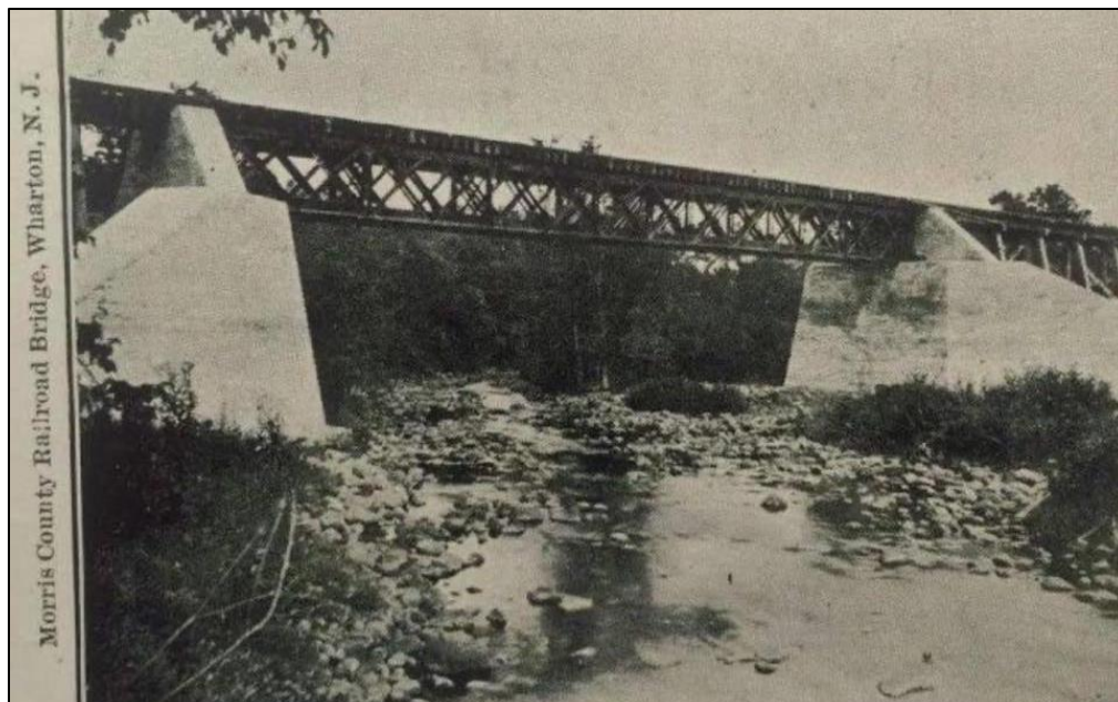
Figure 20. Photo of the trestle (far left and right) and the bridge (center) of the Wharton & Northern over the Rockaway River, No date.
