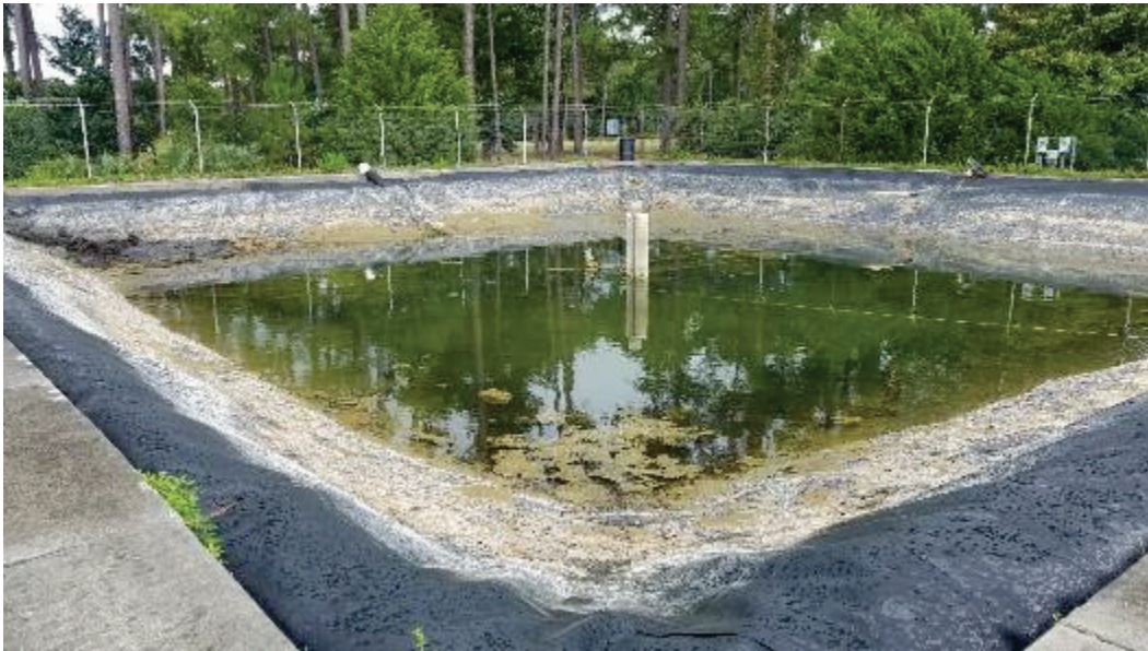
Figure 39. Pond at end of demonstration—Hurlburt Field, demonstration 2.
