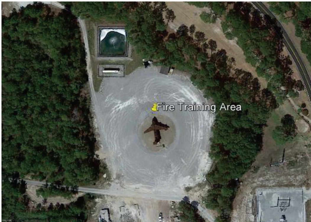
Figure 26. Aerial View of Fire training facility at Hurlburt Field.
