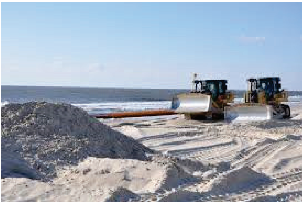
Figure 2-4. Bulldozers moving sand creating the new beach profile. Photo credit: USACE: New York District.
