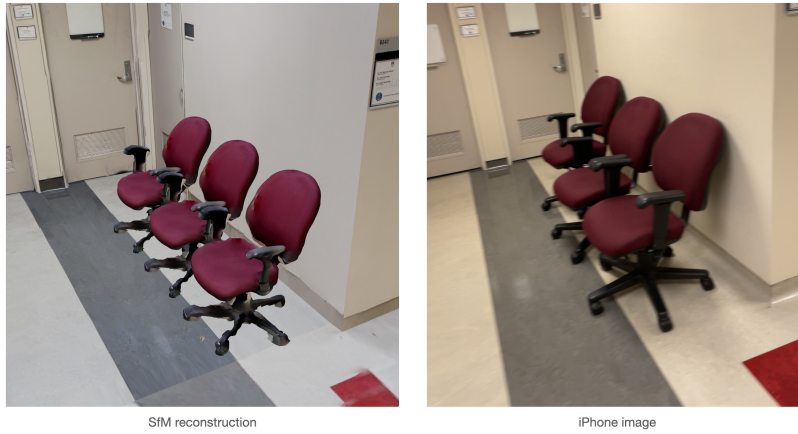
Figure 14: More intractable blemishes. Note the seam in the floor, legs of the chairs and warping around door frames.
