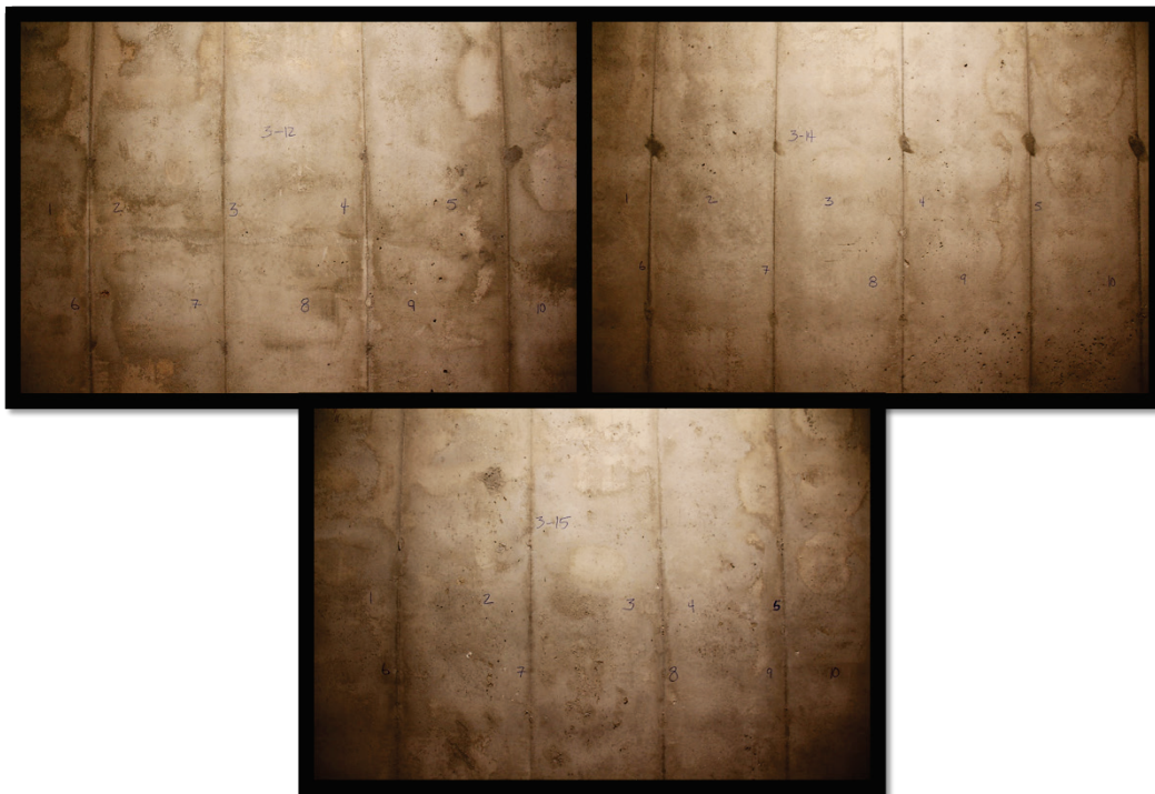
Figure B37. Rebound hammer test locations in Tower 3—Floors 12, 14, and 15.
