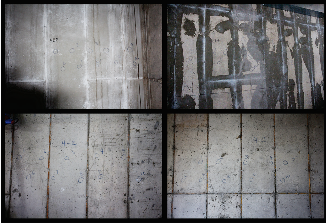
Figure B45. Rebound hammer test locations in Tower 4—Basement through Floor 3.
