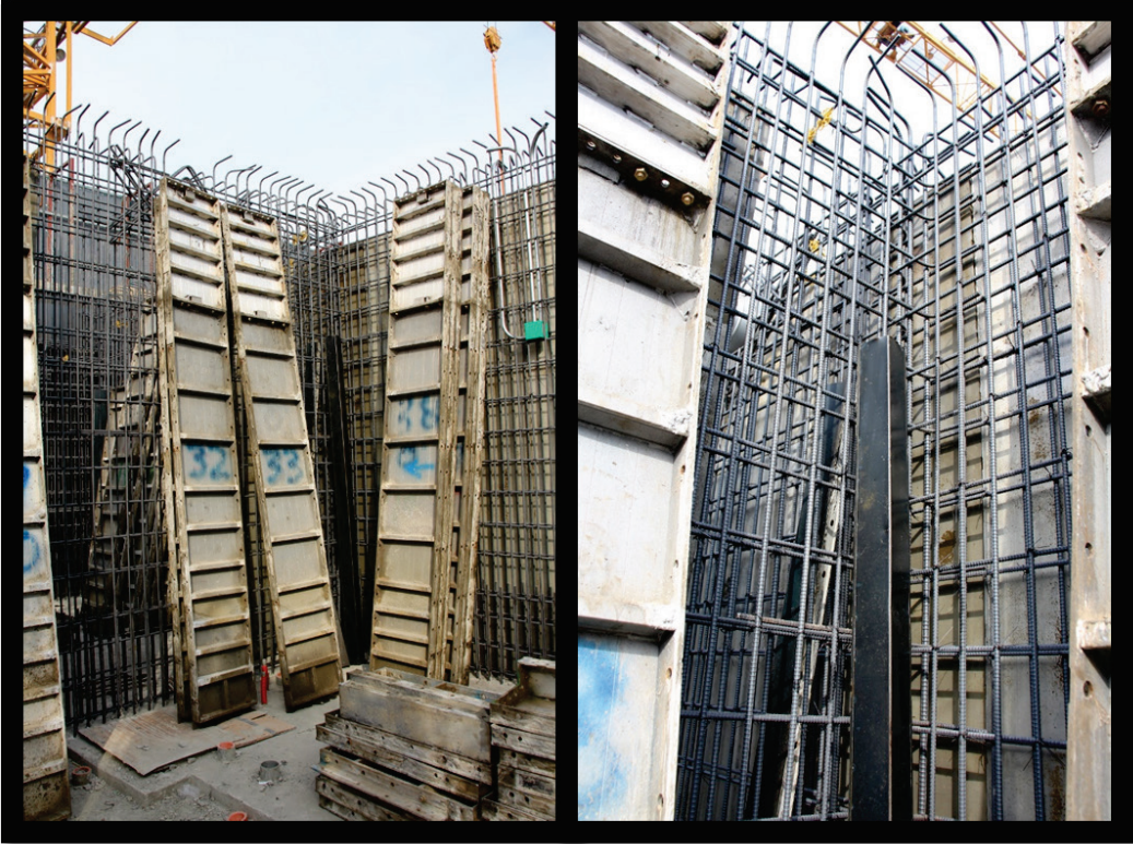
Figure B49. Wall reinforcement of Floor 15 in Tower 4.
