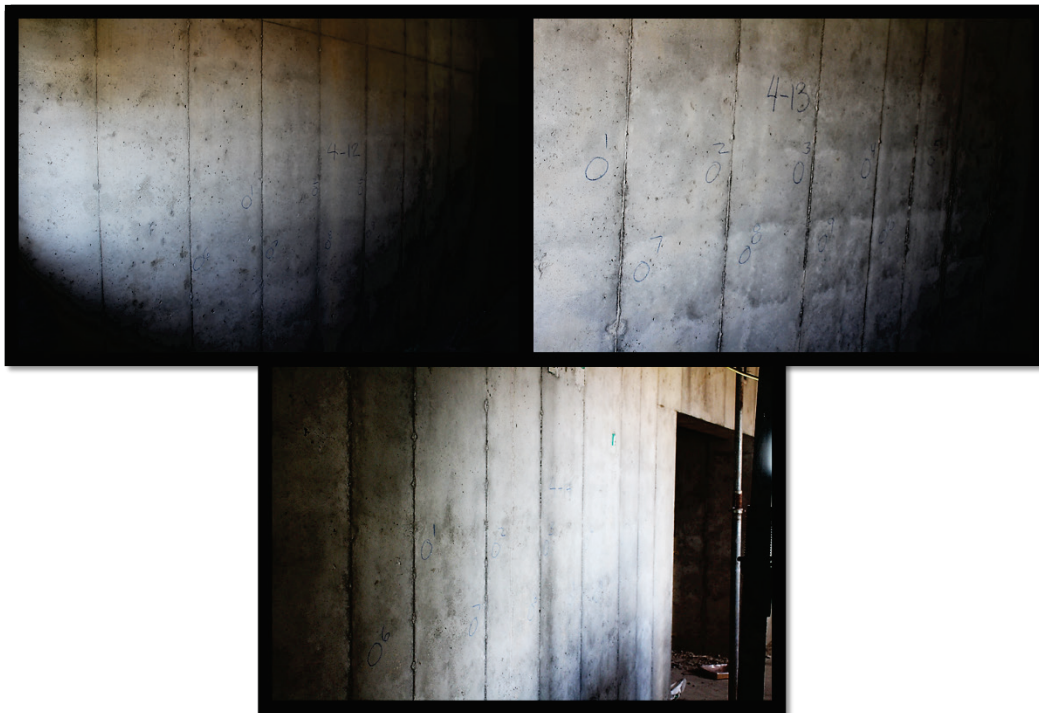
Figure B48. Rebound hammer test locations in Tower 4—Floors 12 through 14.
