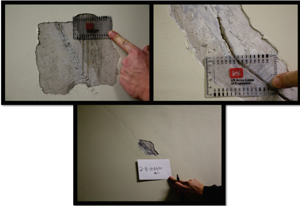
Figure B18. Sealed cracks in Tower 2 basement.
