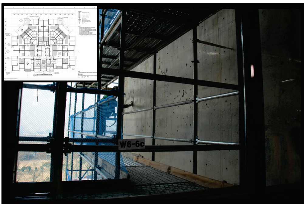
Figure 33. Patching of voids in exterior concrete of Tower 4 (floorplan insert).
