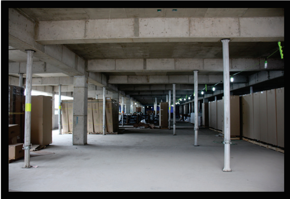
Figure B67. Shoring for girders and beams throughout Parking Garage 4.
