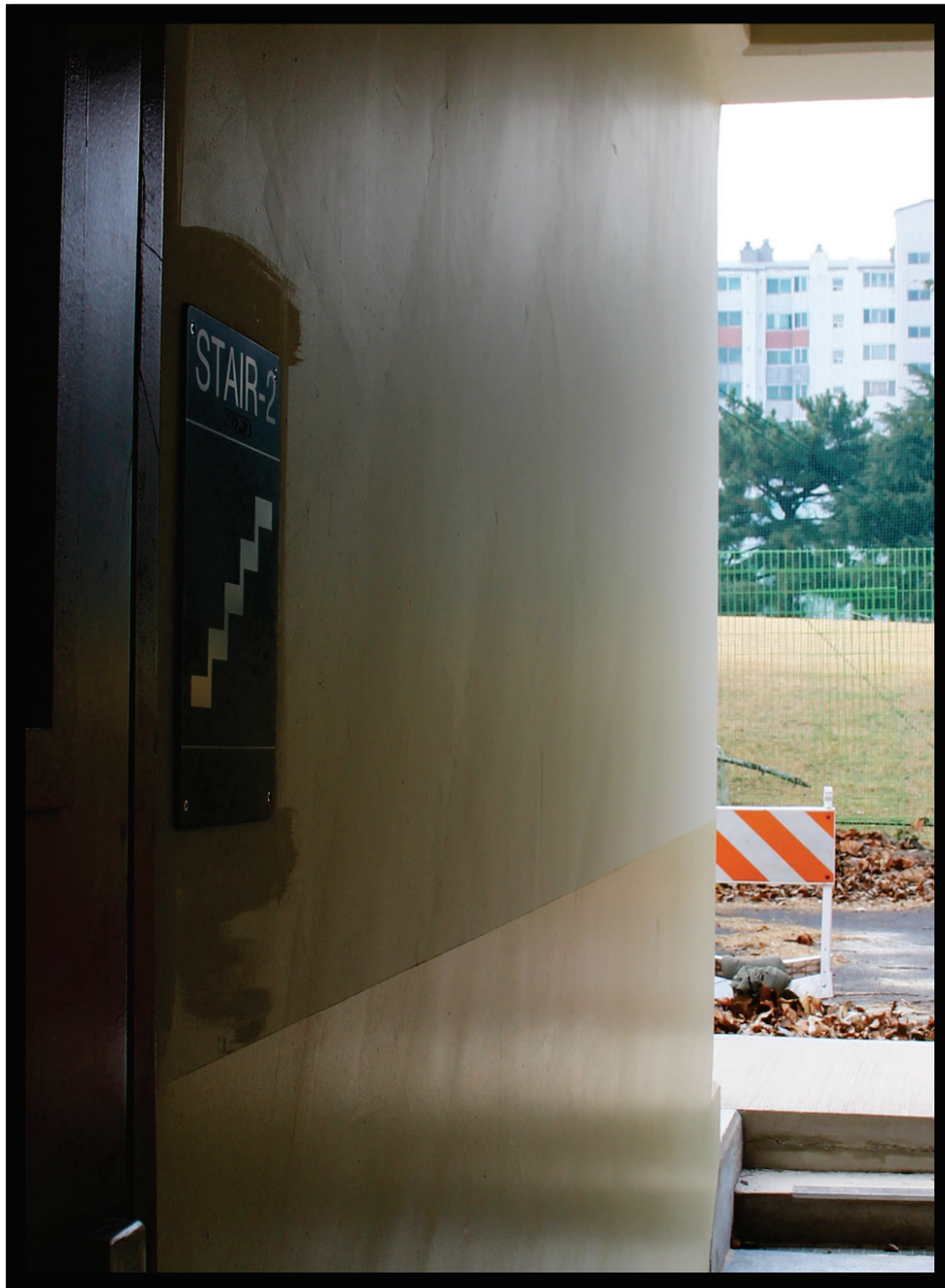
Figure 52. Repaired wall of cracked stairwell in Parking Garage 3.
