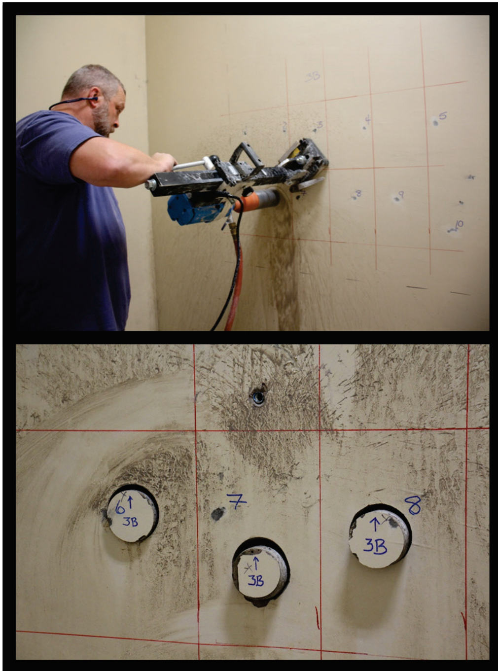
Figure B38. Coring activities in basement of Tower 3.
