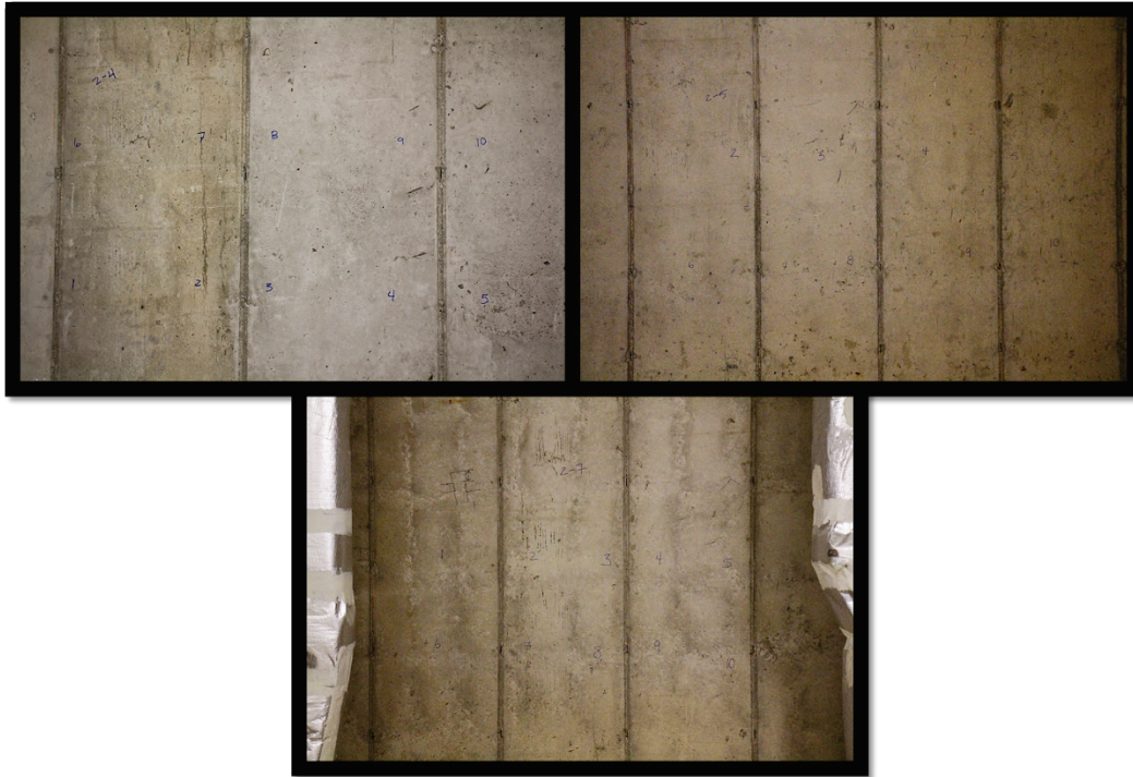
Figure B28. Rebound hammer test locations in Tower 2—Floors 4, 5, and 7.
