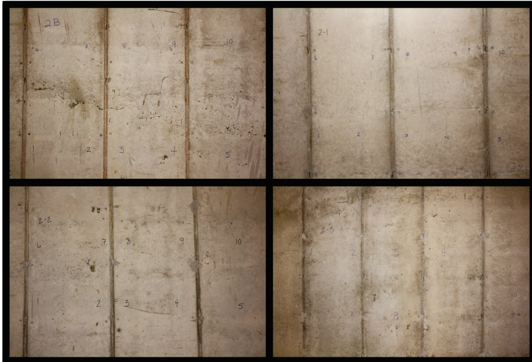
Figure B27. Rebound hammer test locations in Tower 2—Basement through Floor 3.
