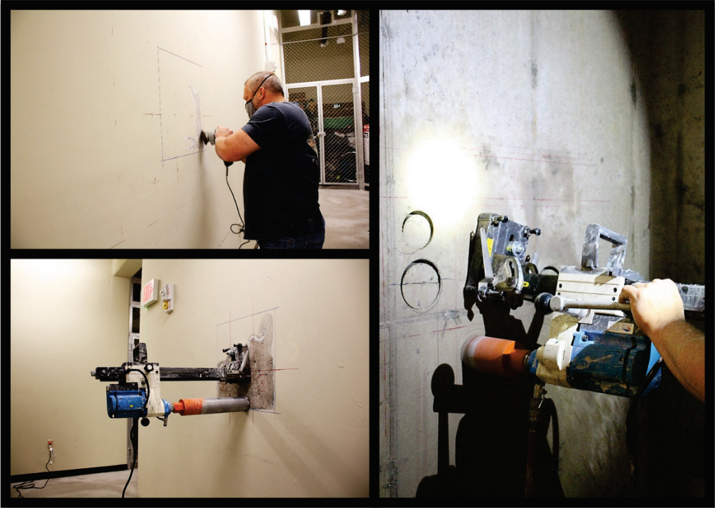
Figure B11. Coring activities in Tower 1.
