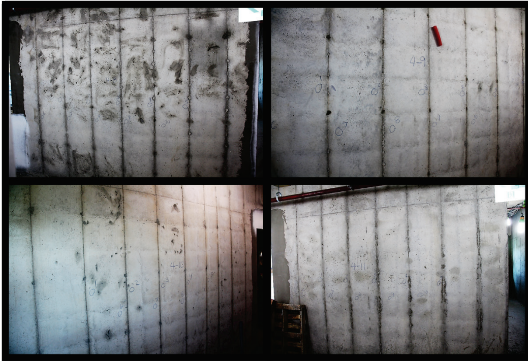
Figure B47. Rebound hammer test locations in Tower 4—Floors 8 through 11.
