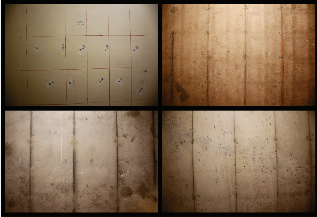
Figure B34. Rebound hammer test locations in Tower 3—Basement through Floor 3.
