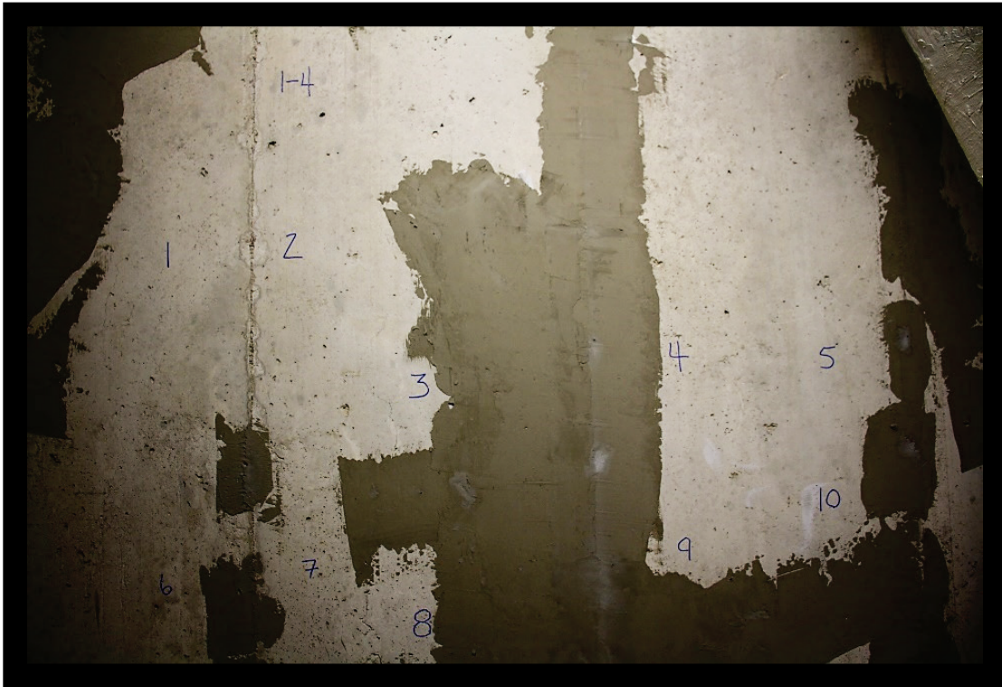
Figure B6. Rebound hammer test locations in Tower 1—Floor 4.
