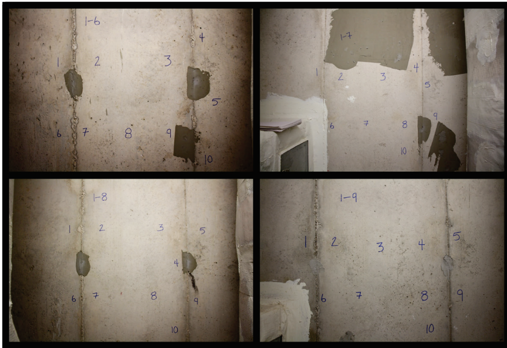
Figure B8. Rebound hammer test locations in Tower 1—Floors 6 through 9.
