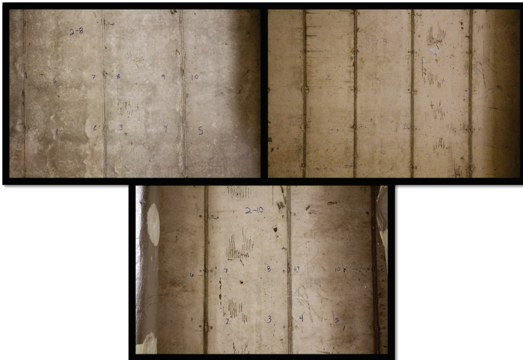
Figure B29. Rebound hammer test locations in Tower 2—Floors 8, 9, and 10.
