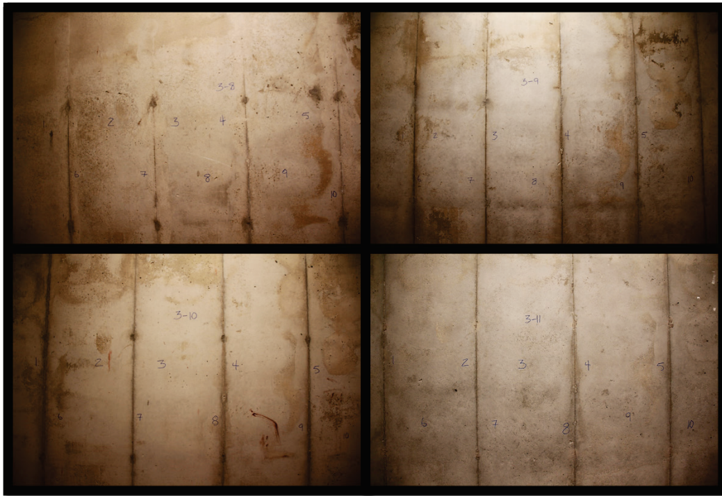
Figure B36. Rebound hammer test locations in Tower 3—Floors 8 through 11.
