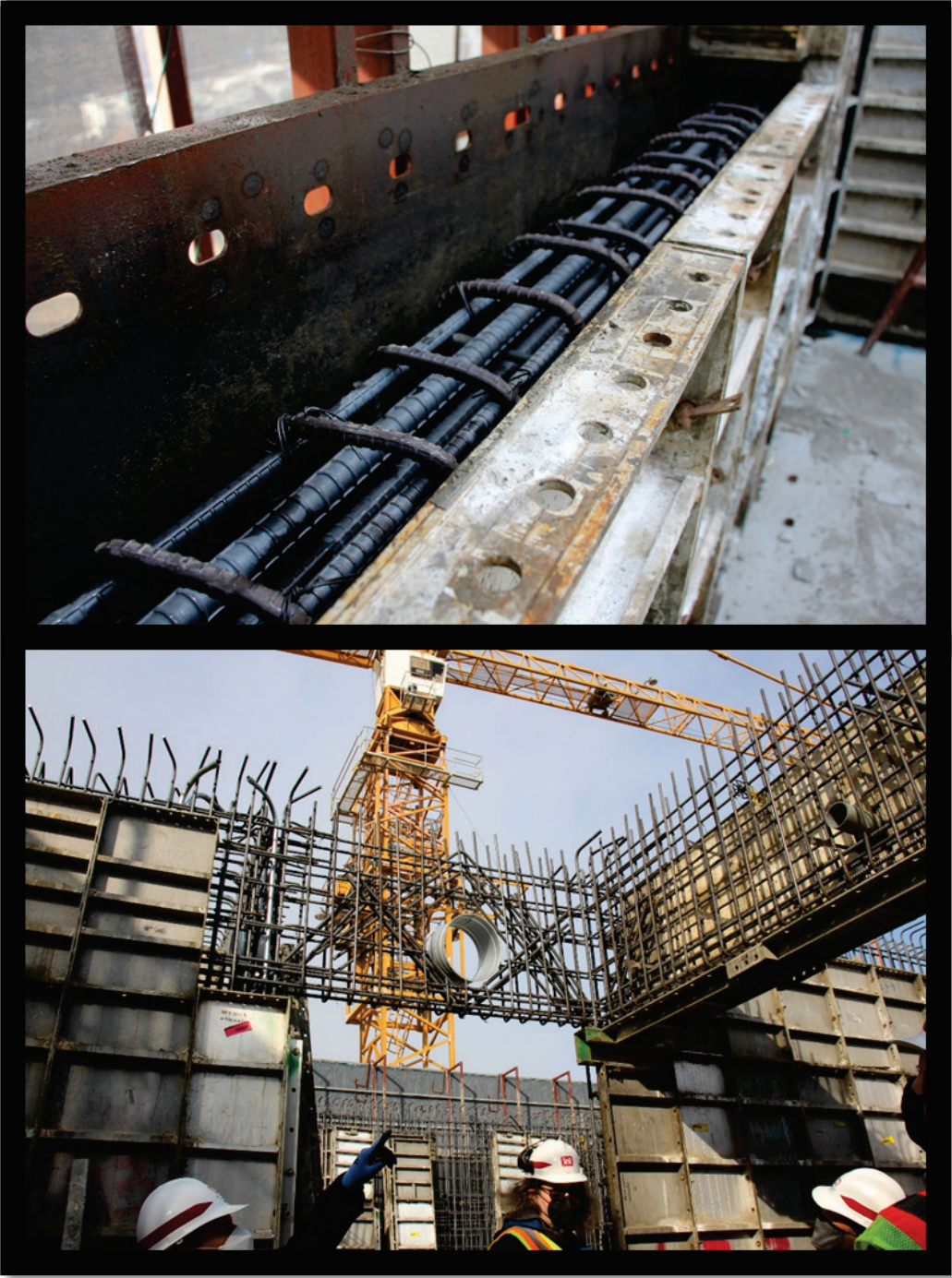
Figure B50. Reinforcement on Floor 15 of Tower 4.
