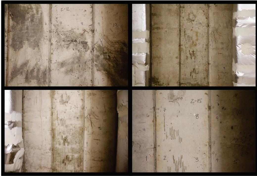
Figure B30. Rebound hammer test locations in Tower 2—Floors 12 through 15.
