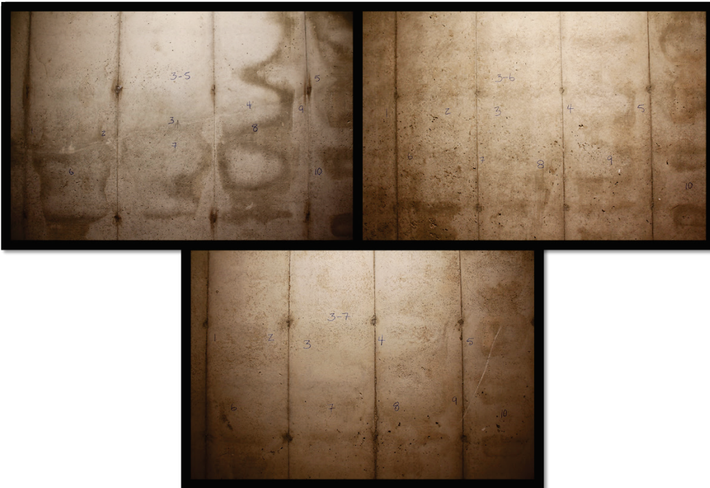
Figure B35. Rebound hammer test locations in Tower 3—Floors 5, 6, and 7.
