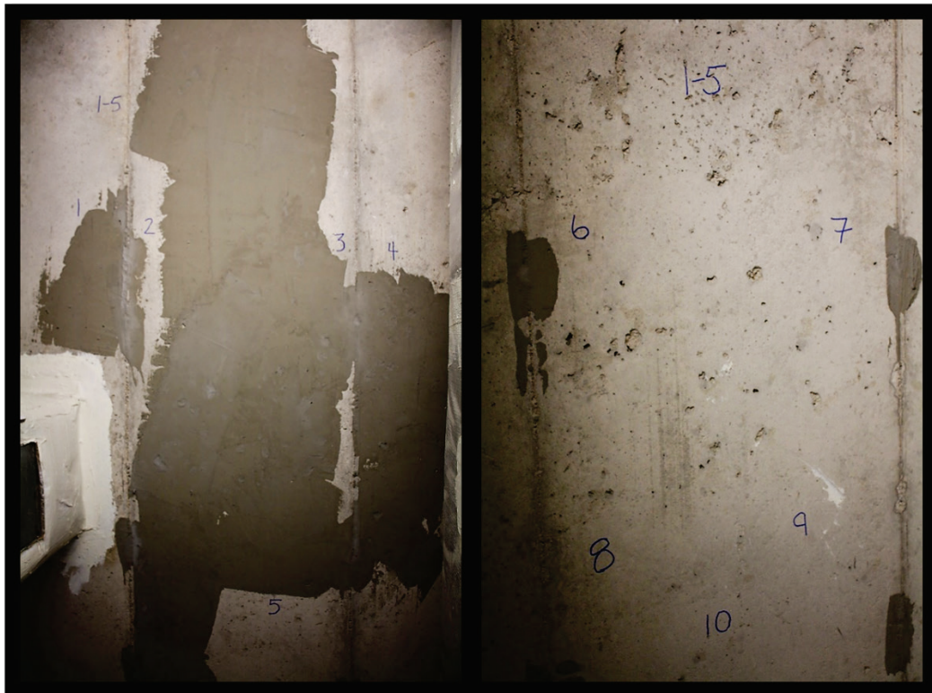
Figure B7. Rebound hammer test locations in Tower 1—Floor 5.
