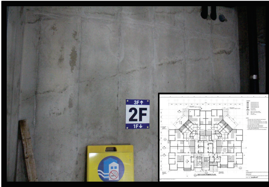
Figure 31. Observed cold joint in Tower 4 stairwell (floorplan insert).
