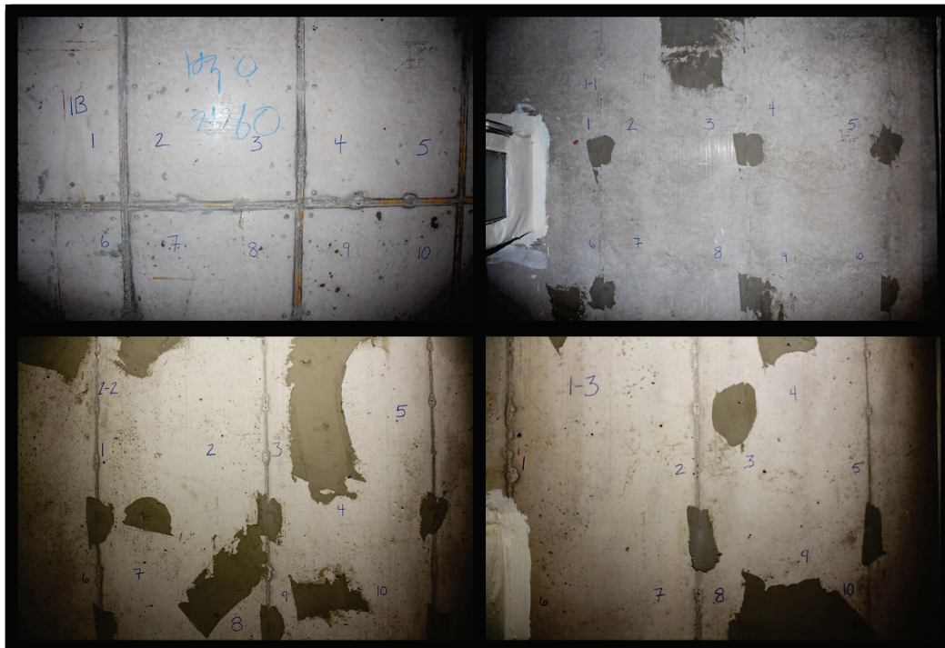
Figure B5. Rebound hammer test locations in Tower 1—Basement through Floor 3.
