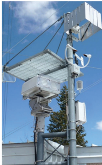
Figure 61. WTLE Transmitter, Weather Station, and Disdrometer
