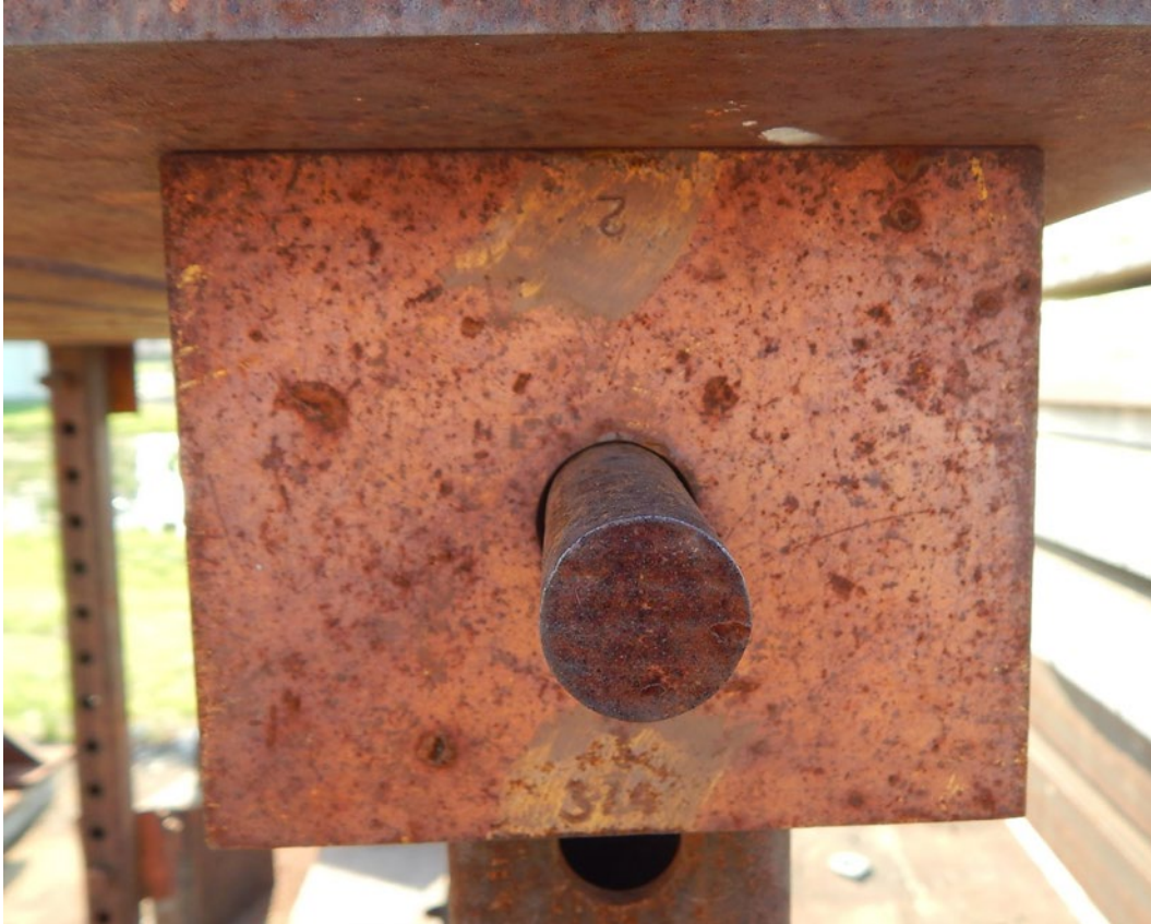
Fig. 2 Shim placement for target alignment
