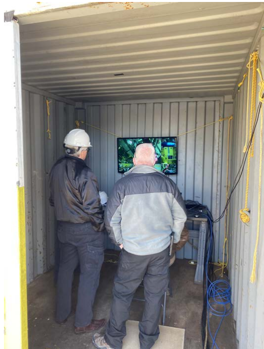
(d) Operational container used to control the tool package and view cameras during operation.
