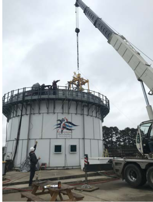
(b) Tool package being hoisted into the large test tank.
