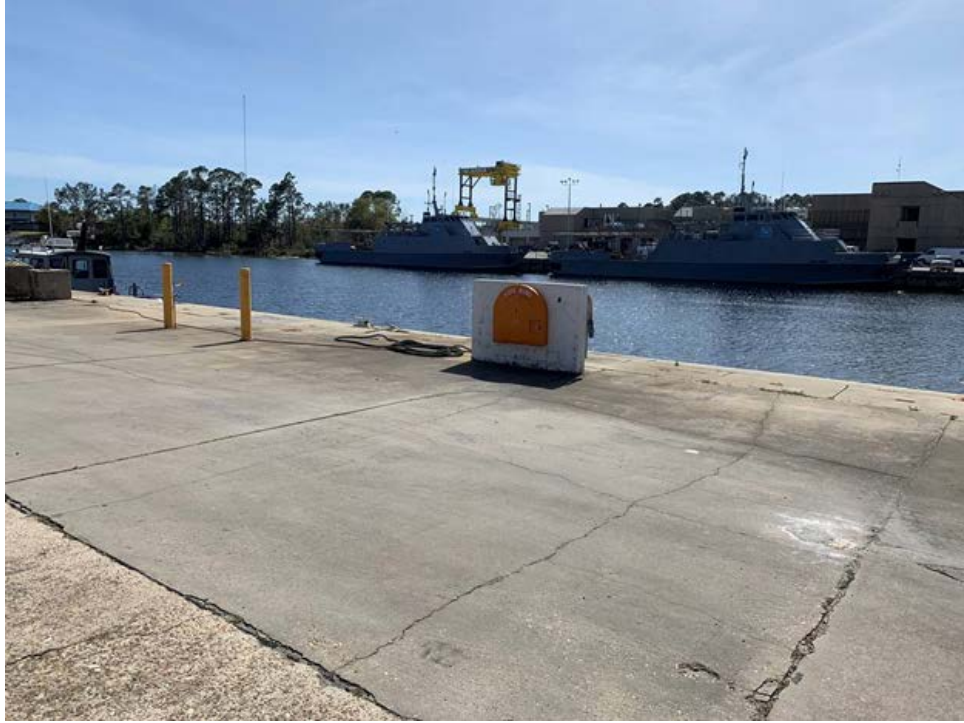
Figure 15. Area for locating the utility equipment.
