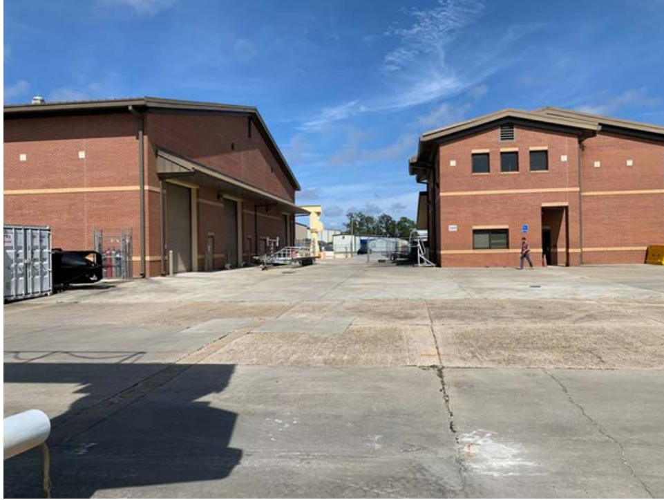
Figure 13. Bayou is directly behind photographer and the crane is to the left; Building 582 is on the right and is where the generator and high-pressure pump will be located.
