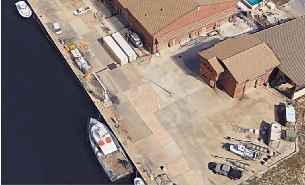
Figure 8. Overhead view of pier and gantry crane where the open water demonstration will occur.
