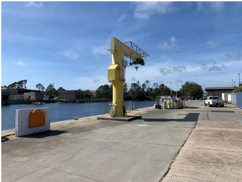
Figure 14. Gantry crane that will be used to deploy the tool package.
