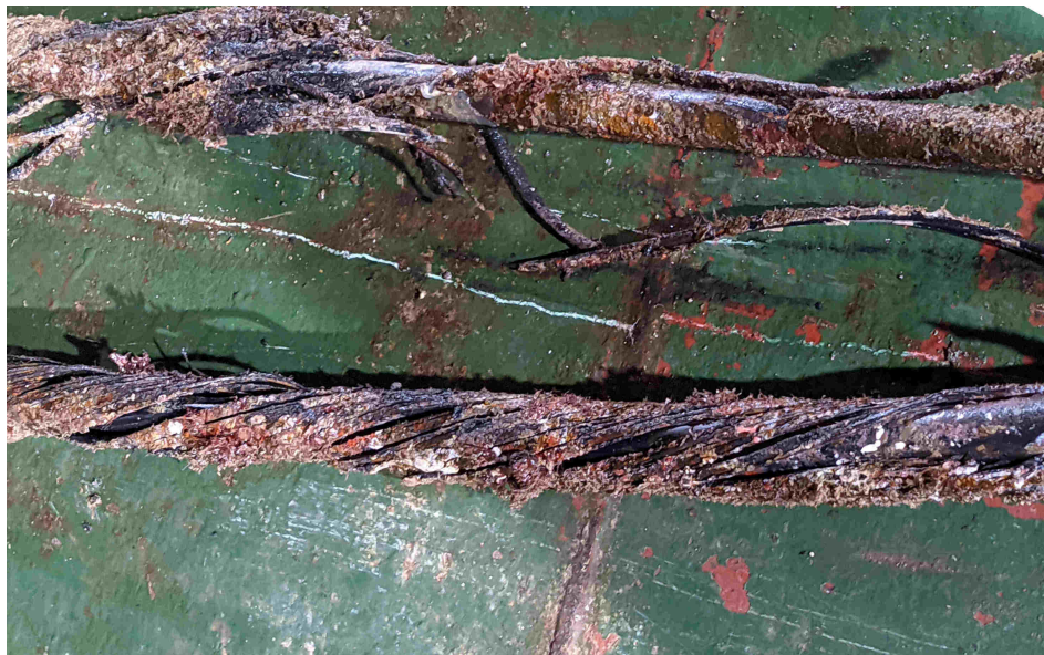
Figure 17: Abrasion damage in the shoreward end of the SDL3 cable. The armor on the top example is completely gone in the middle.
