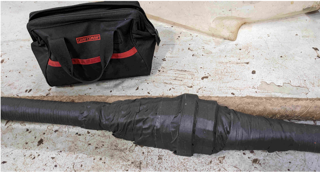
Figure 13: The SDL3 to SDL3 splice (armored to armored), after completion.
