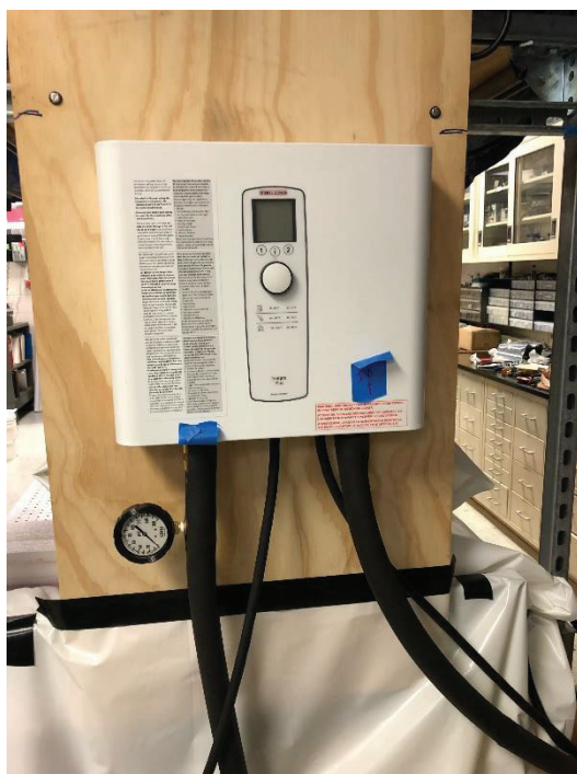
Figure 10.4: Cold water chiller for cool RB plate
