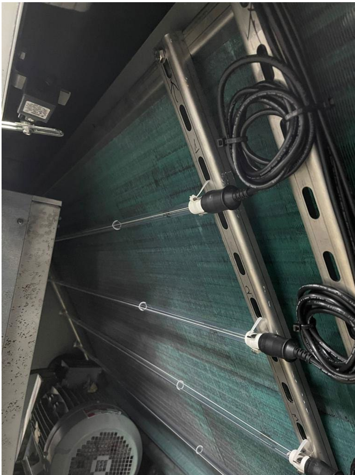
Figure 25. Deck-mounted public-area fan coil unit with 100% recirculation and UV off. Source: Carnival Corporation HVAC Working Group (2021).
