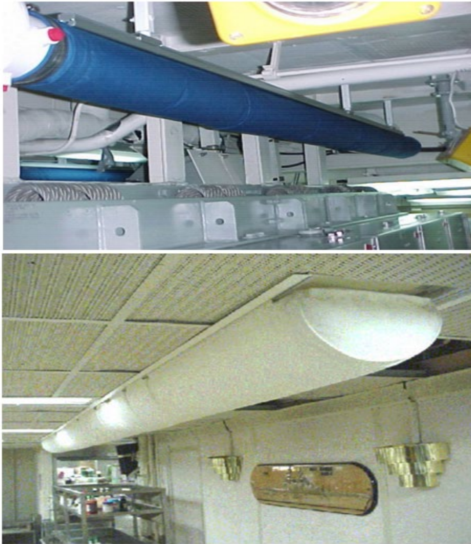
Figure 2. The purpose of the textile ducting is to distribute air used in HVAC systems aboard U.S. Navy Ships. The ductwork can be either from fire-resistant textile material or galvanized steel or aluminum. Galvanized steel and aluminum may provide higher reflective values for the installation of UVGI lamps. Adapted from Naval Sea Systems Command (2006).
