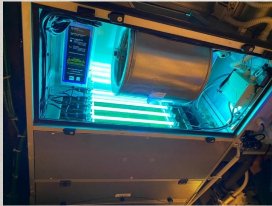
Inspection of a public-area fan coil unit. 100% recirculation suction is at the bottom, with exhaust flow at the top.
