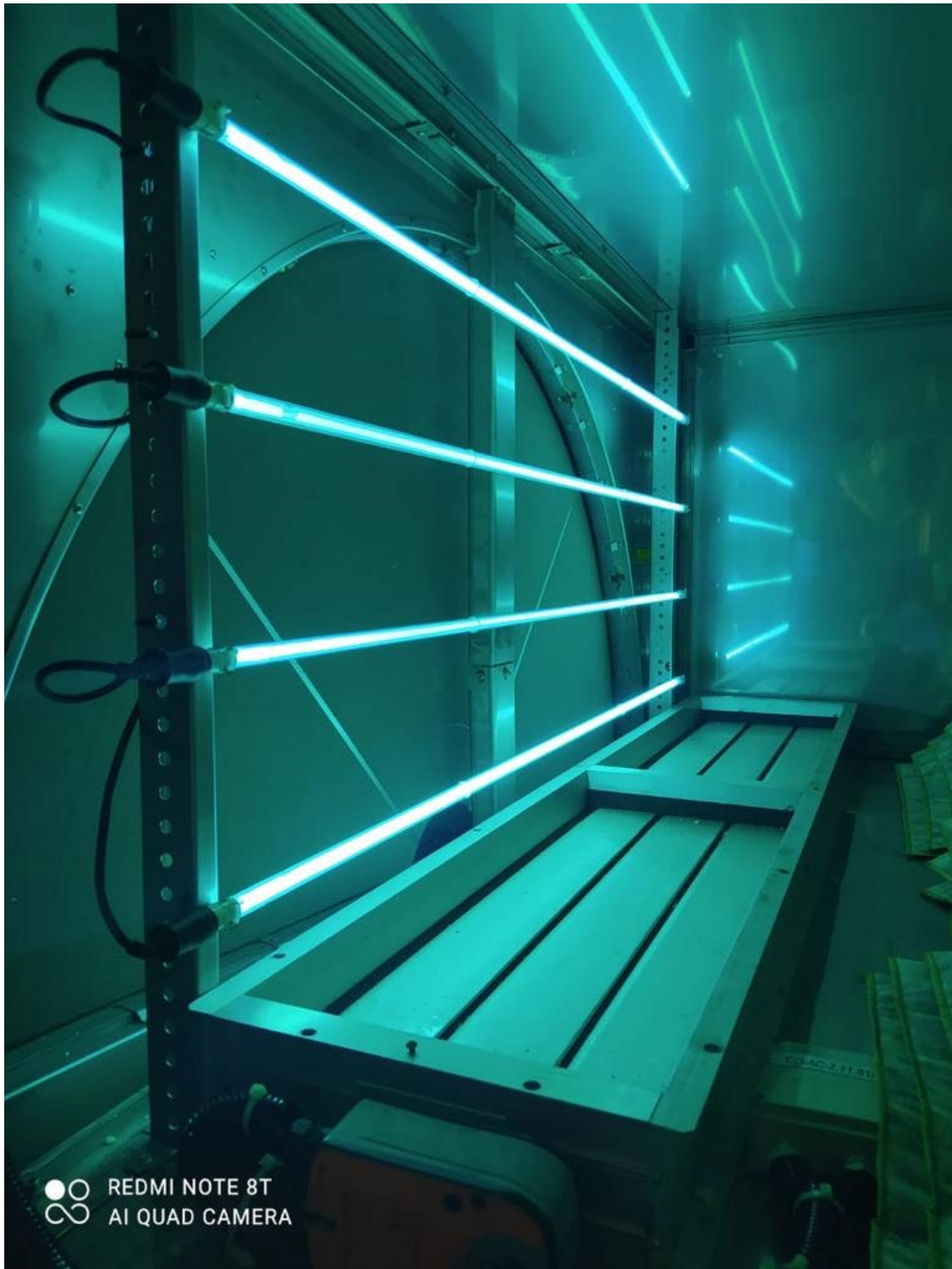
Figure 26. Main air handling unit (AHU) with Sorption wheels (for energy recovery) and modulating recirculation damper, as seen from exhaust side. Source: Carnival Corporation HVAC Working Group (2021).
