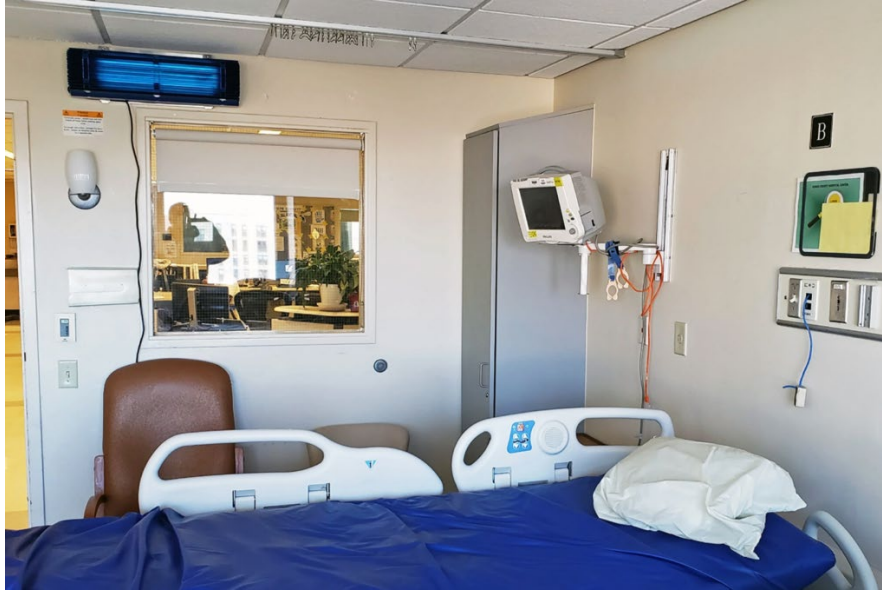
Figure 11. Photo of an upper-room UVGI device used in a hospital room. UVGI systems have been used to disinfect the air inside rooms where tuberculosis patients have resided. Louvers on the UVC device unit reflect the UVC light up and away from any pathogens present in the room. It is important to follow device safety instructions by placing these units 7 or 8 feet above the deck. Source: Chang (2020).
