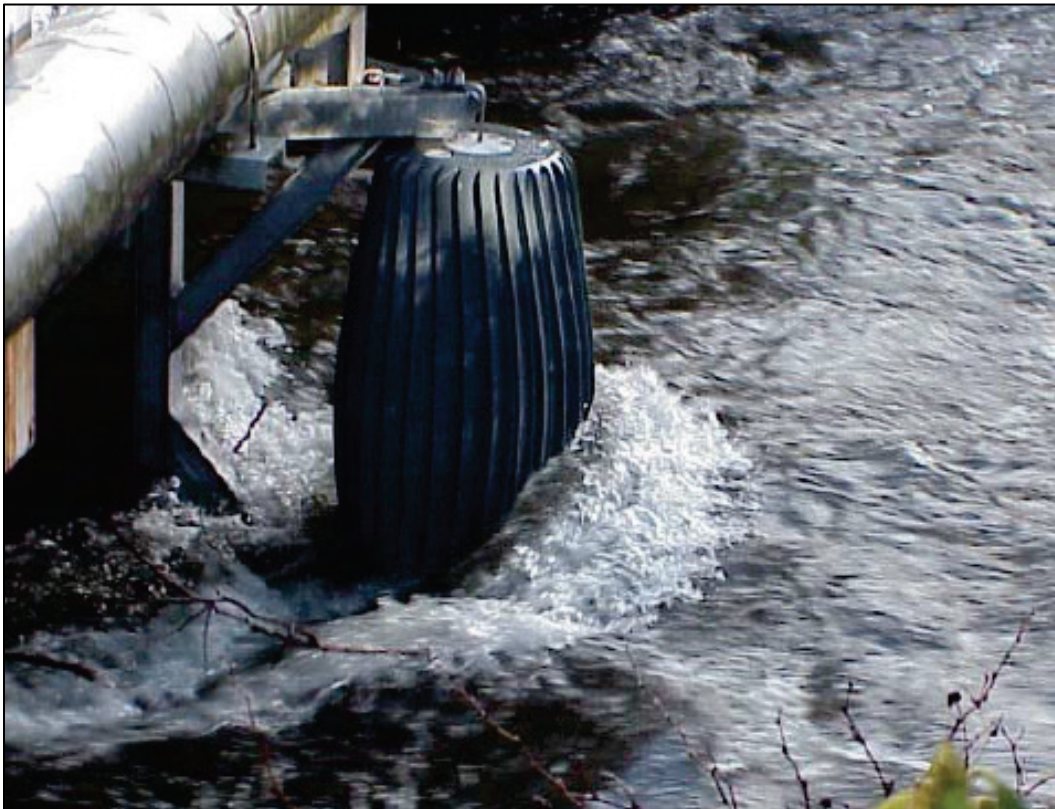
Figure 8. Debris sweeper installed on the Cedar Creek in Washington, USA (Bradley et al. 2005).
