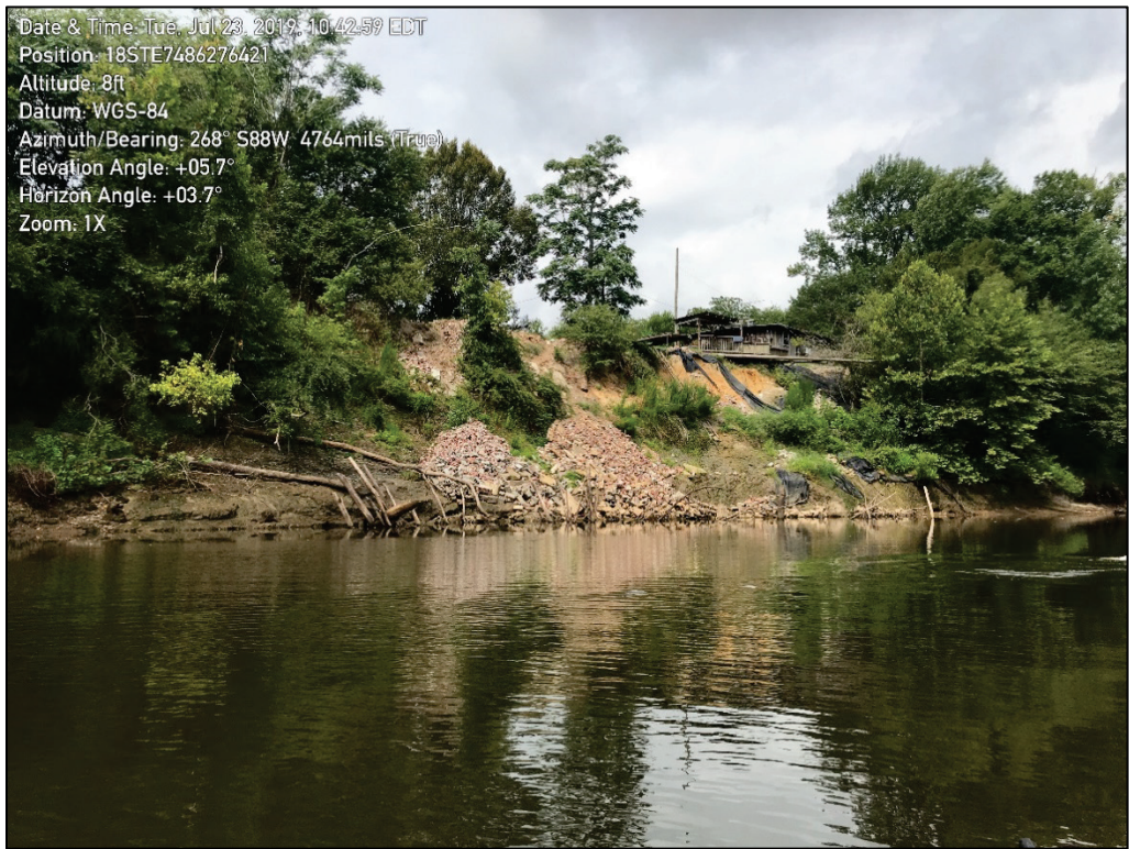
Figure A-8. Possible past stabilization efforts on the Tar River near Tarboro, NC.
