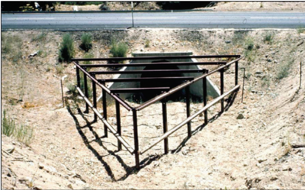
Figure 10. Debris deflector protecting a culvert from debris accumulation (Bradley et al. 2005).
