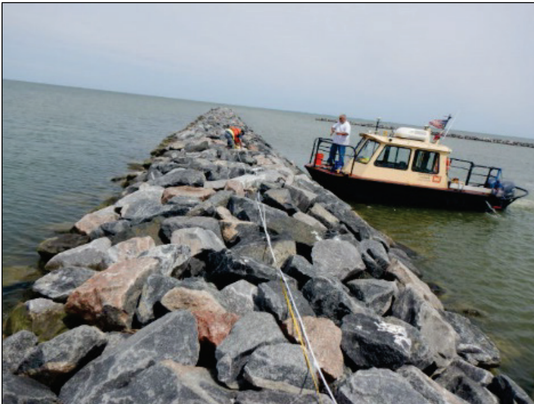
Figure 4. Crew setting up transects for analysis of structural stability.
