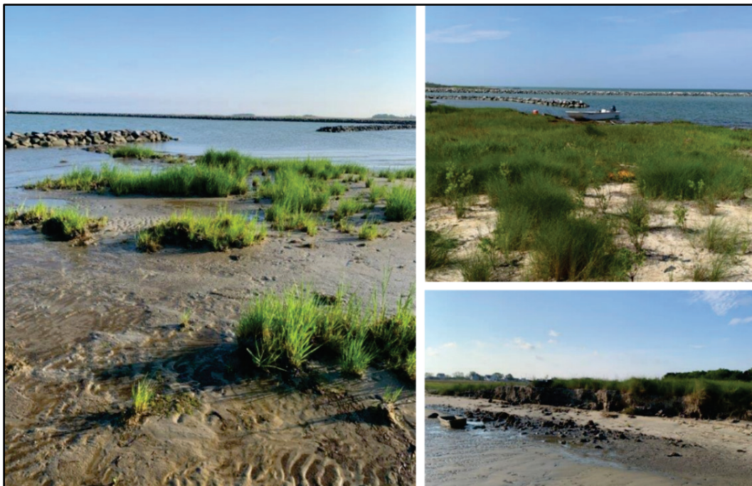
Figure 15. Left: Plantings along the shoreline behind the sill (June 2020). Right, top: Plantings at the north placement site. Right, bottom: Formation of scarp behind gap in segmented sill.
