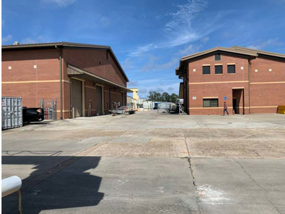
Figure 22. Bayou Is Directly Behind Photographer and the Crane Is to the Left; Building 582 is on the Right and Was Where the Generator and High-pressure Pump Were Located.
