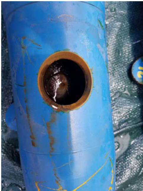
(c) Item #21 after cutting, plug removal, and washout.
