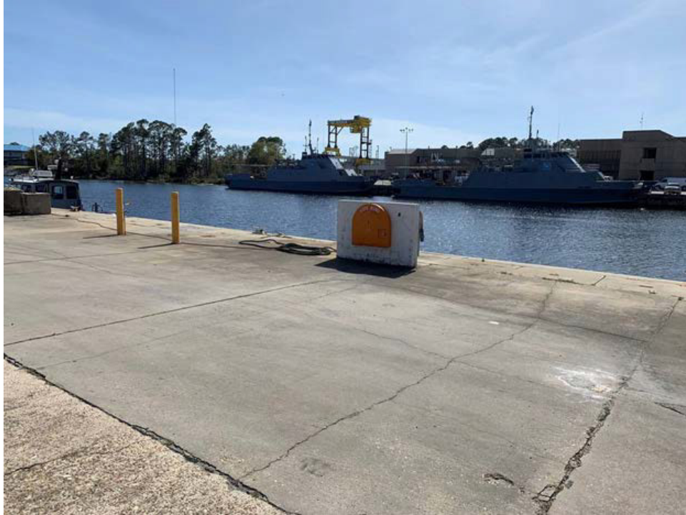
Figure 24. Area Where Utility Equipment Was Located.
