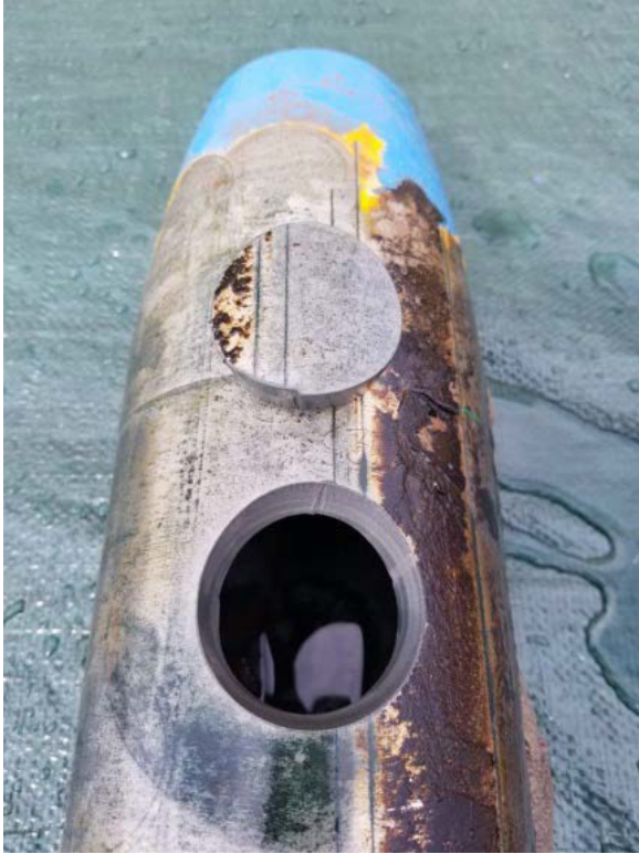
(a) Item #15 after concrete removal, cutting, and plug removal.
