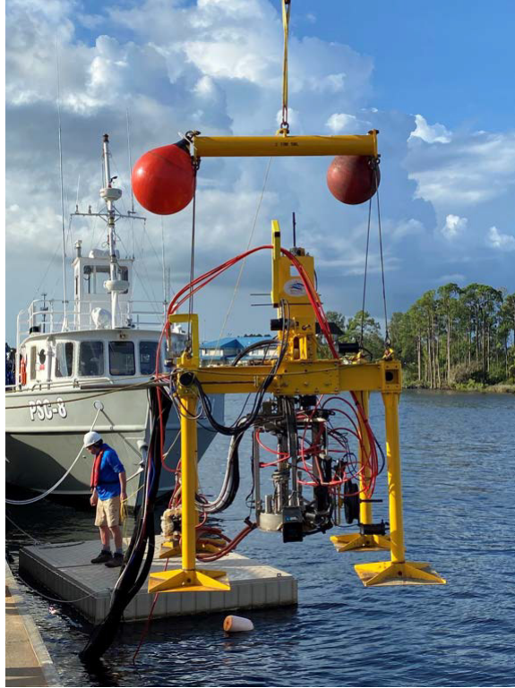
(a) Tool package being lowered into the water
