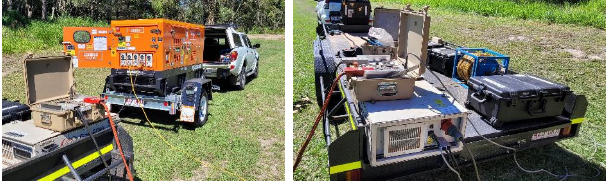
Figure 16. Proof-of-Concept testing of transmitter loop configurations. (left) 20 kVA three phase generator, (right) power supply and transmitter (Model EODTx200).
