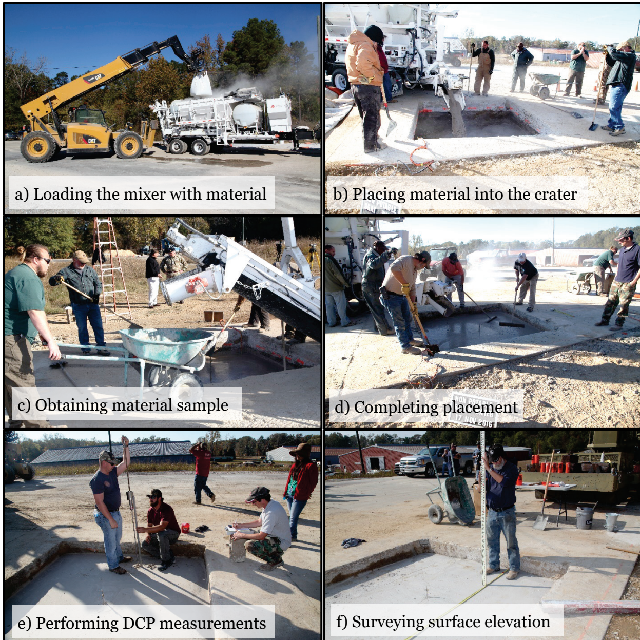
Figure 15. CSA flowable fill placement process.
