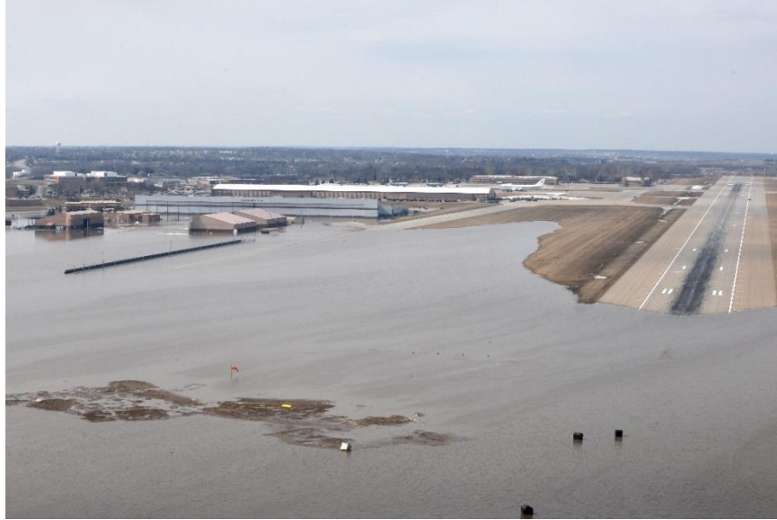
Figure 1: Airfield Flooding at Offutt AFB (55th Wing Public Affairs 2019)
