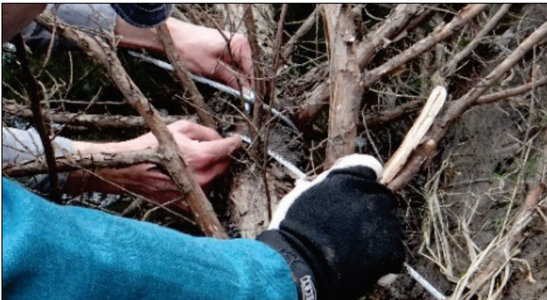
Figure 4. A cable is wrapped around the cedar trunk and secured with a cable clamp.
