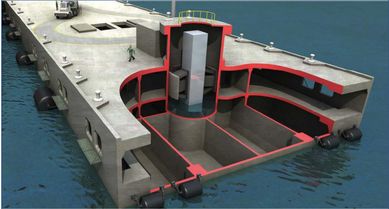
Figure 7B: Floating Double-Deck Pier. Source NAVFAC, https://www.navfac.navy.mil/content/dam/navfac/Specialty%20Centers/Engineering%20and%20Expeditionary%20Warfare%20Center/PDFs/ci_tech_data_sheets/TDS-NAVFAC-EXWC-CI-1410.pdf
