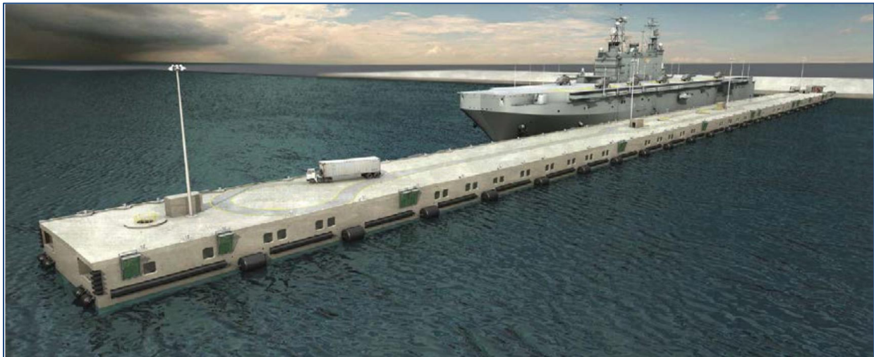
Figure 7A: Floating Double-Deck Pier. Source NAVFAC, https://www.navfac.navy.mil/content/dam/navfac/Specialty%20Centers/Engineering%20and%20Expeditionary%20Warfare%20Center/PDFs/ci_tech_data_sheets/TDS-NAVFAC-EXWC-CI-1410.pdf
