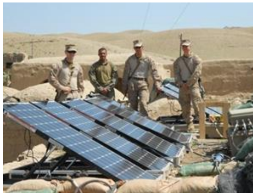
Fig 2: Infantry Battalion Uses GREENS to Power COC Communication Equipment (Source: https://www.hqmc.marines.mil/e2o/Fleet/ )
