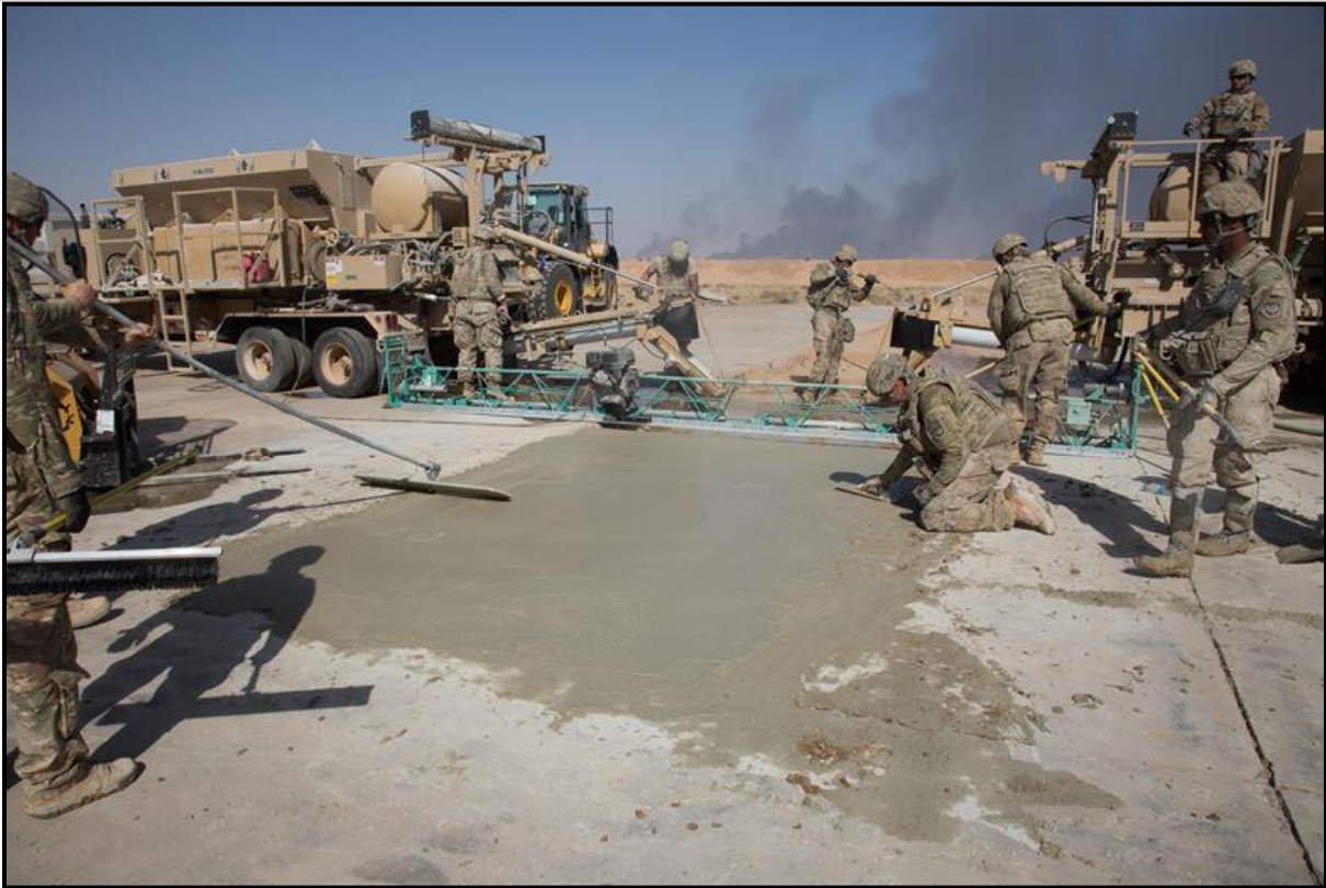
Figure 5: Civil engineers repair the Qayyarah West runway to enable the Mosul Offensive Source: SSgt Charles Rivezzo, “Q-West to Support Mosul Offensive,” Air Forces Central , 25 October 2016, https://www.afcent.af.mil/News/Article/985022/air-force-engineers-restore-q-west-to-support-mosul-offensive/
