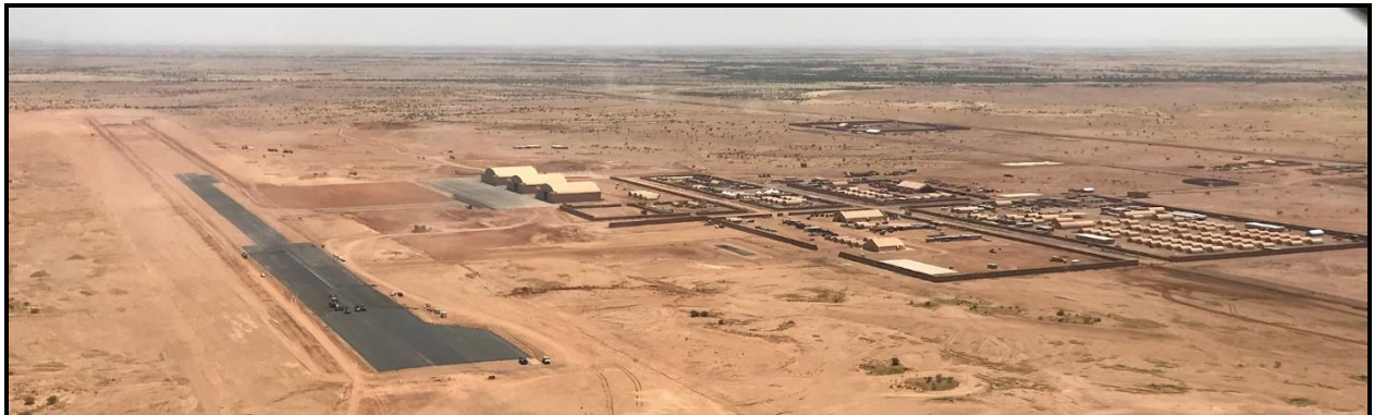
Figure 7: Engineers construct an airfield in the Saharan Desert
