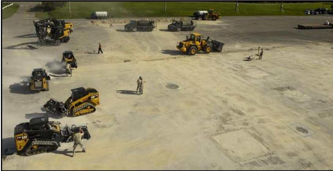
Figure 6: Engineers execute rapid airfield damage repair during Exercise Resilient Shogun
