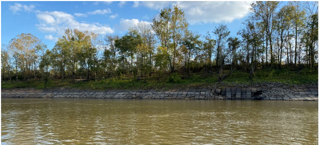
Figure 2: Revetment along the Atchafalya River
