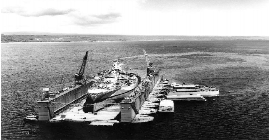
Figure 1. ABSD-1 with West Virginia docked off Espiritu Santo in the New Hebrides Islands. This dry dock is of the open-ended design where the ship sails into the dock when it is underwater and then is raised by pumping mechanisms. (Courtesy of the Naval Historical Center) 5
