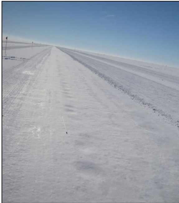
Figure 47. Refrozen road with a washboard surface.
