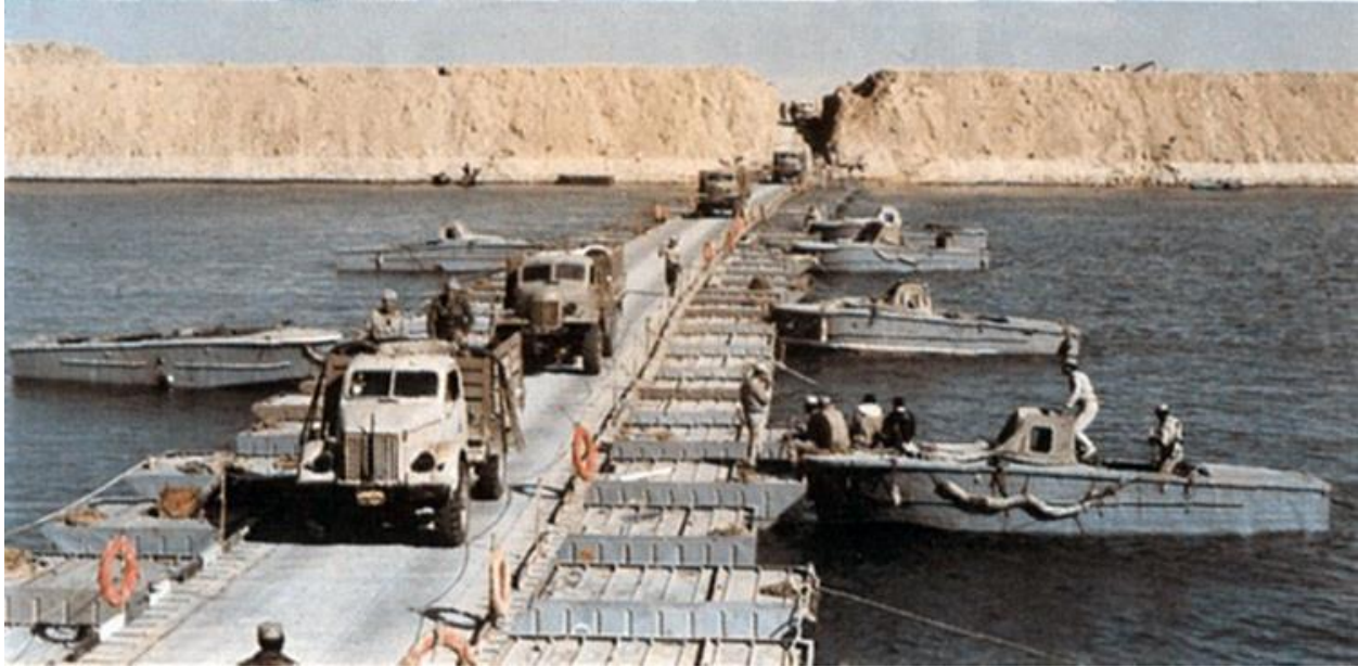
Photo 2: Shows one of several bridge crossings constructed by the Egyptians. It spanned the width of the Suez Canal, which varies between 590 to 720 feet. It was built in a matter of hours following the blasting of passages through the earthen defensive wall. 24
