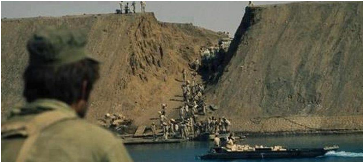
Photo 1: The 70' high earthen defensive wall is shown, along with a passage blasted through the sand by Egyptian combat engineers using high pressure water. Israeli defense plans assumed it would take a minimum of 12 hours to blast through the sand wall using explosives, giving Israel adequate time to mobilize reserve forces. High pressure water broke through in 3 hours. 23
