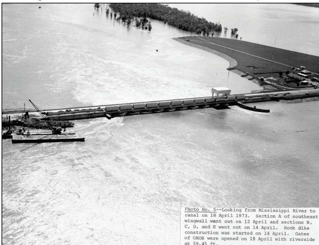
Figure 7. Construction of rock dike on left abutment on 18 April 1973.
