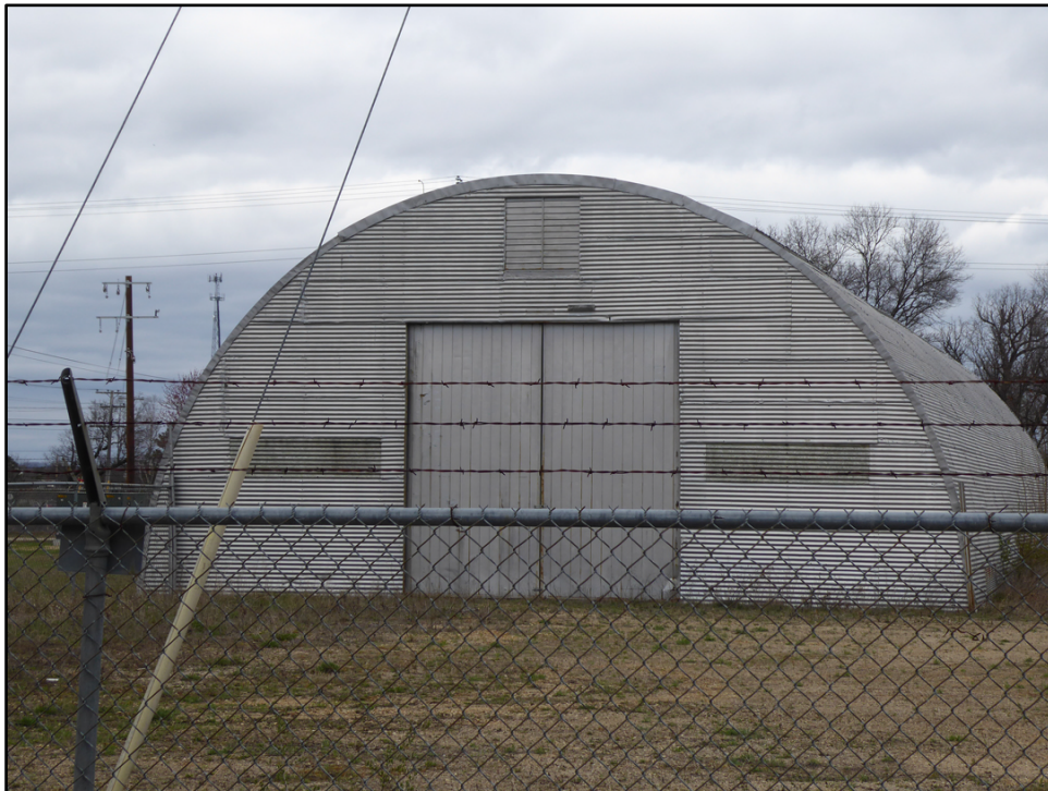
Figure 48. South side of Building 2176 (ERDC-CERL 2021).
