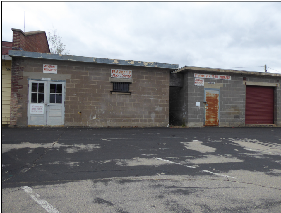
Figure 56. North side of Building 2199 ( left ) and Building 2198 ( right ) (ERDC-CERL 2021).
