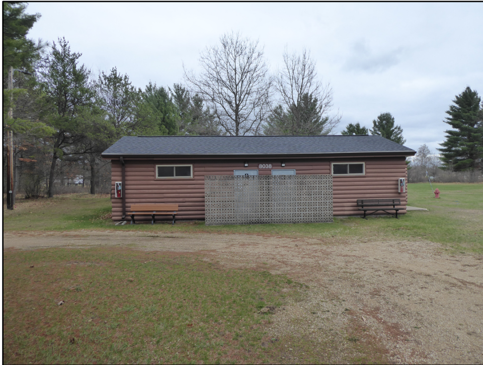
Figure 62. West side of Building 8038 (ERDC-CERL 2021).
