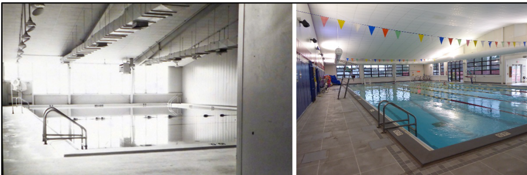
Figure 77. Comparison image of an interior view of the pool area looking southeast in Building 1122, Rumpel Fitness Center. Left is historic photograph (1978) with original vaulted ceiling, concrete flooring, wall of large multipane industrial-style windows on the east side and no window openings on the south wall versus the right image from 2021 showing newer concrete flooring, replacement windows on the east wall, newer windows and doors added to the south wall, and a solarium addition added off the south wall ( left image is RG111-SCA, Album 402A, SC675942, NARA, College Park, MD, and right image is from ERDC-CERL, 2021. Public Domain).
