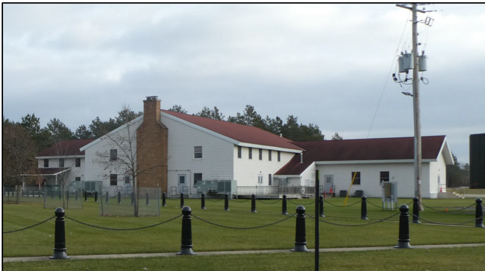
Figure 34. Northeast side of Building 905, Service Club No. 3 (ERDC-CERL 2020).
