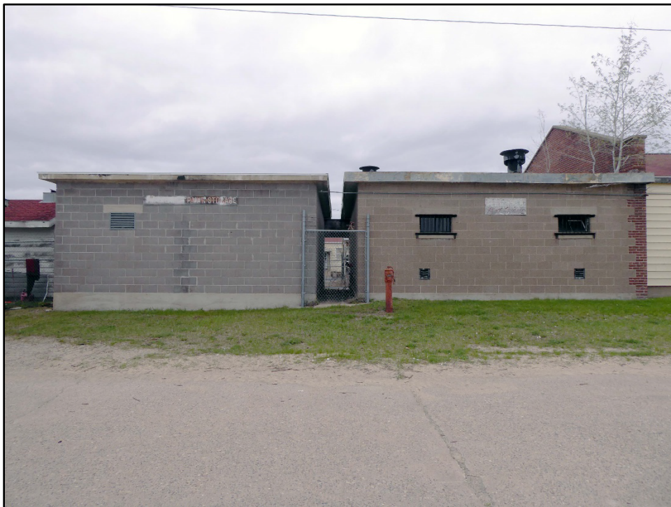
Figure 57. South side of Building 2199 ( right ) and Building 2198 ( left ) (ERDC-CERL 2021).
