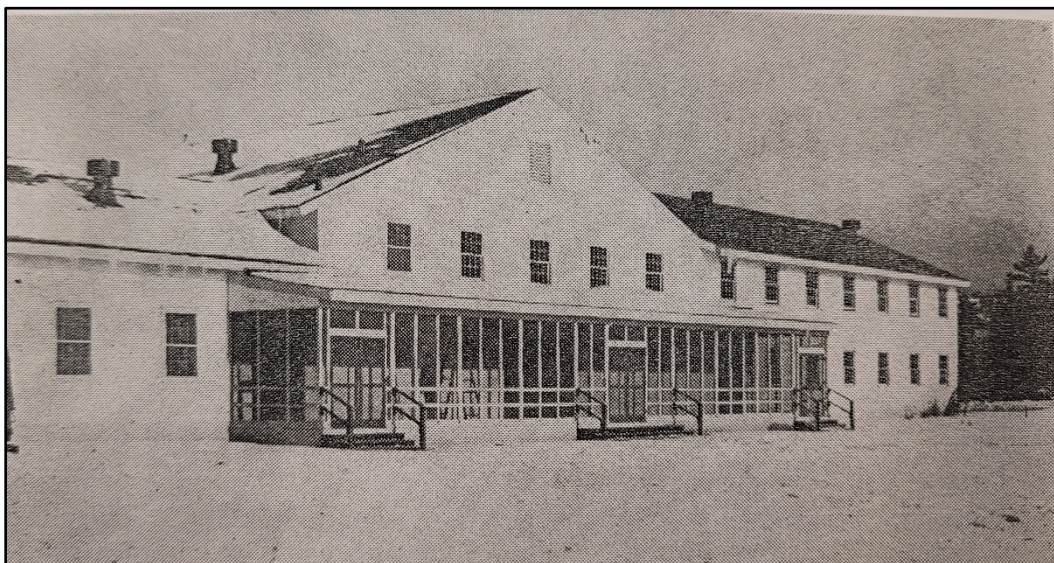
Figure 11. Building 905, Service Club No. 3, after reconstruction, January 1953 (La Crosse Sunday Tribune. Public Domain).
