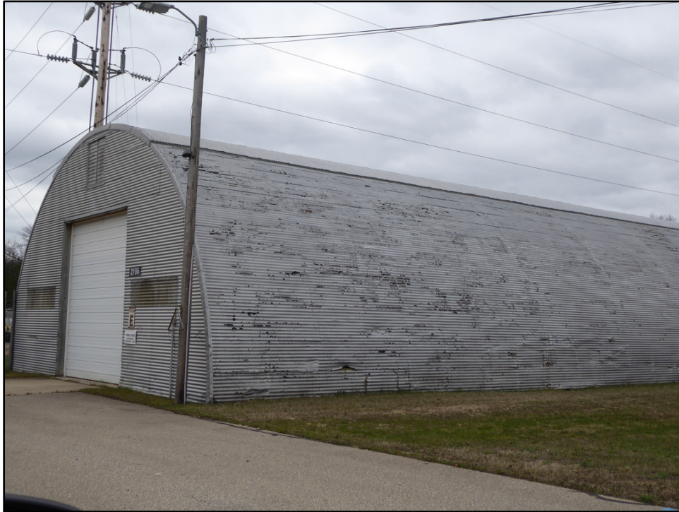
Figure 50. Northwest oblique of Building 2186 (ERDC-CERL 2021).
