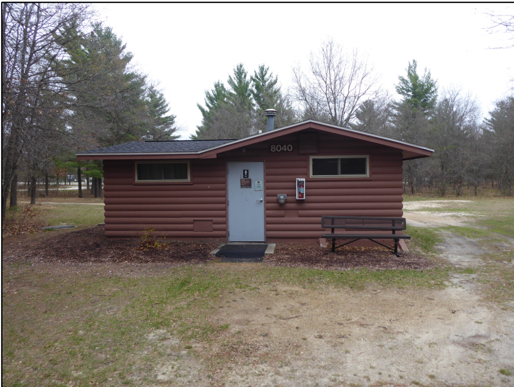
Figure 67. Southwest side of Building 8040 (ERDC-CERL 2021).
