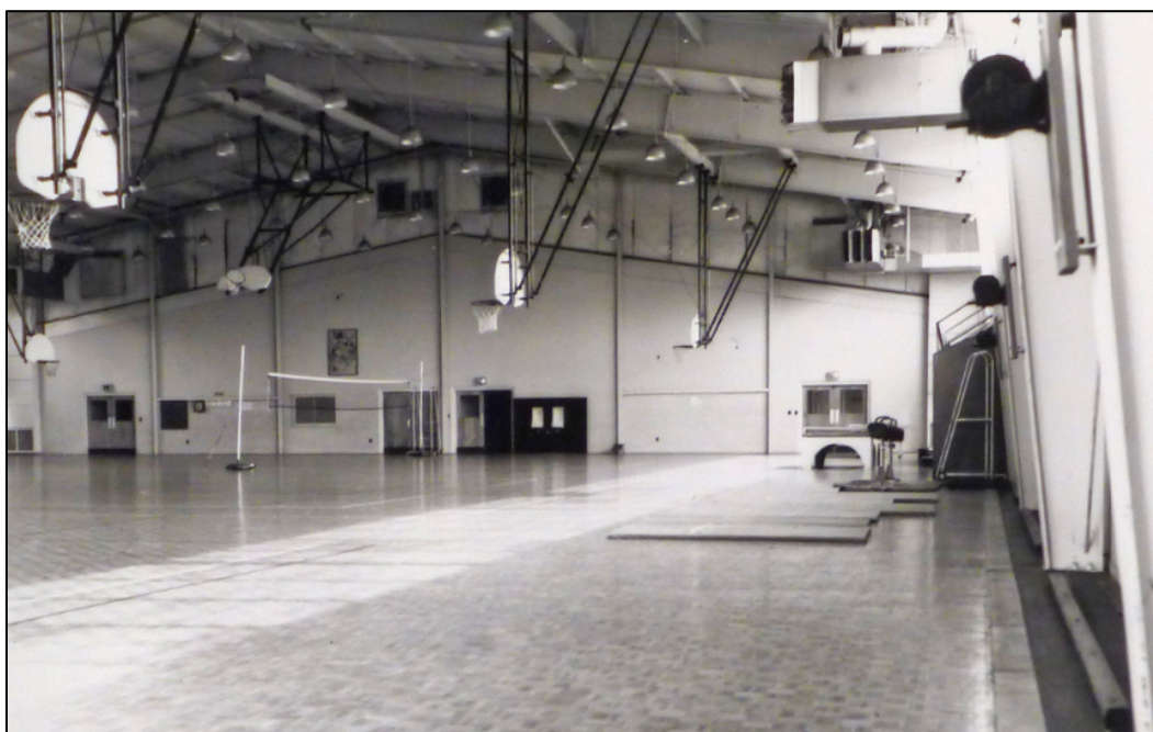
Figure 24. Special Services gym in Building 1122, July 1978 (Photo no. 675941, July 25, 1978, McCoy, CP. WIS. Book #5, Record Group 111-SCA 400, NARA, College Park, MD. Public Domain).
