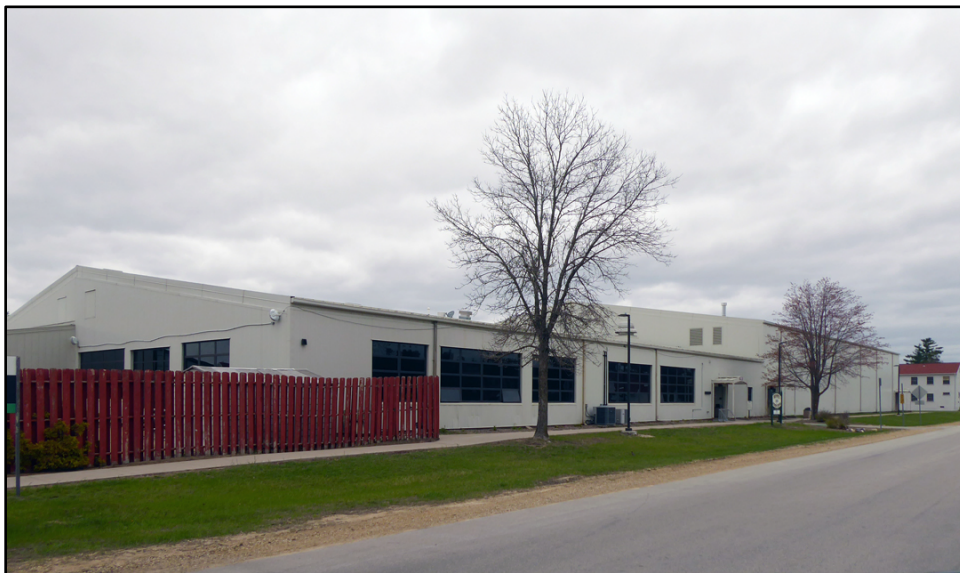
Figure 38. Southeast oblique of Building 1122, Rumpel Fitness Center (ERDC-CERL 2021).
