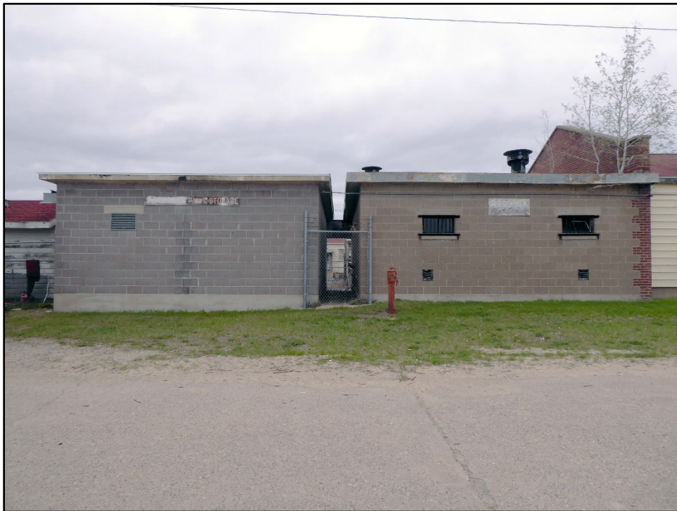
Figure 54. South side of Building 2198 ( left ) and Building 2199 ( right ) (ERDC-CERL 2021).
