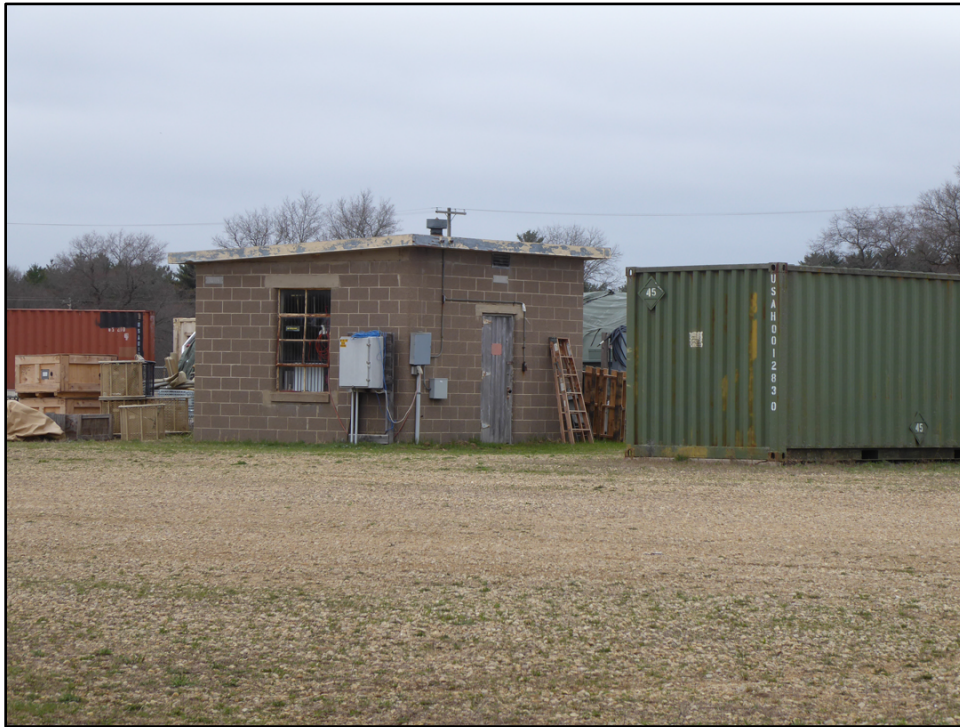
Figure 70. Southeast oblique of Building 10119 (ERDC-CERL 2021).
