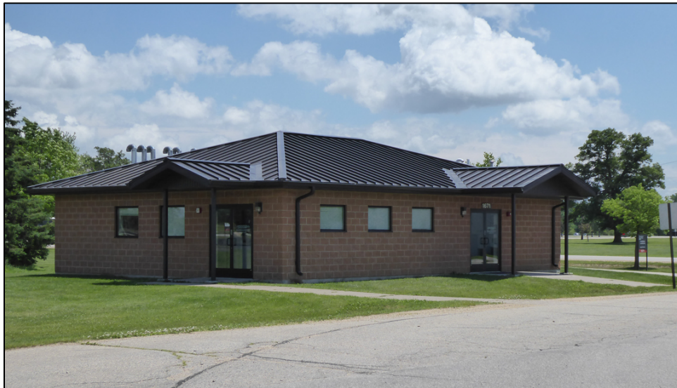
Figure 28. Looking southeast at Building 1671, a new laundry facility, 2020 (ERDC-CERL 2020).
