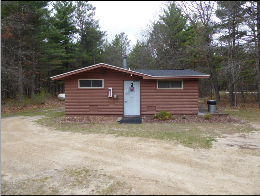
Figure 66. Northwest side of Building 8040 (ERDC-CERL 2021).
