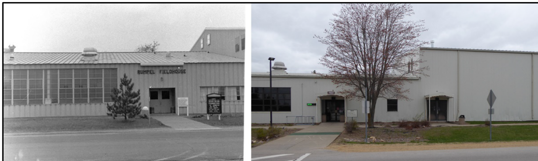
Figure 75. Comparison image of the east side of Building 1122, Rumpel Fitness Center. Left is historic photograph (no date) with original large multipane windows for the pool area, original recessed entry doors, original band of smaller metal windows, metal standing seam siding versus the right image from 2021 showing replacement windows for the pool, removal of the band of smaller windows, replacement entry doors with canopy, and replacement metal siding ( left image is from Fort McCoy DPW, and right image is from ERDC-CERL 2021. Public Domain).
