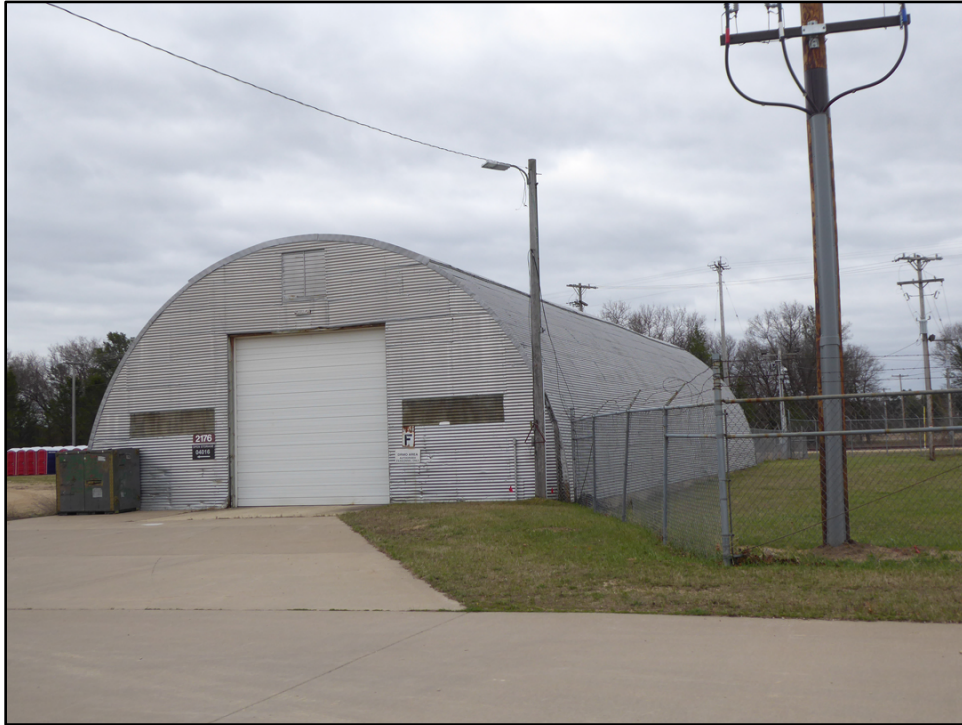
Figure 47. Northwest oblique of Building 2176 (ERDC-CERL 2021).
