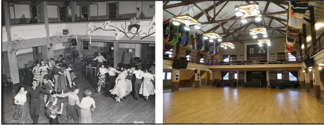
Figure 74. Comparison image of an Interior view looking northwest in the dancehall being used by soldiers dancing in Building 905, Service Club No. 3; left image from 1952, and right image from 2021 ( Left image is Photo no. 401476, April 29, 1952, McCoy, CP. WIS. Book #3, Record Group 111-SCA 401, NARA, College Park, MD, and right image is from ERDC-CERL, 2021. Public Domain).
