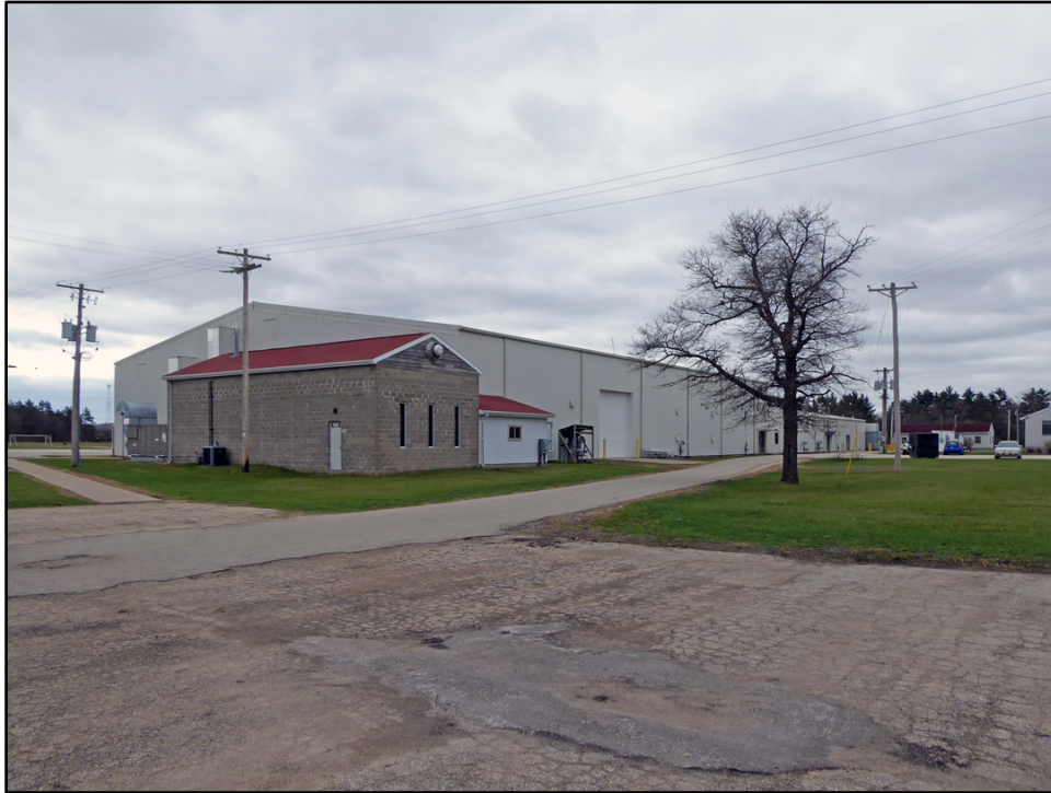
Figure 39. West side of Building 1122, Rumpel Fitness Center (ERDC-CERL 2021).
