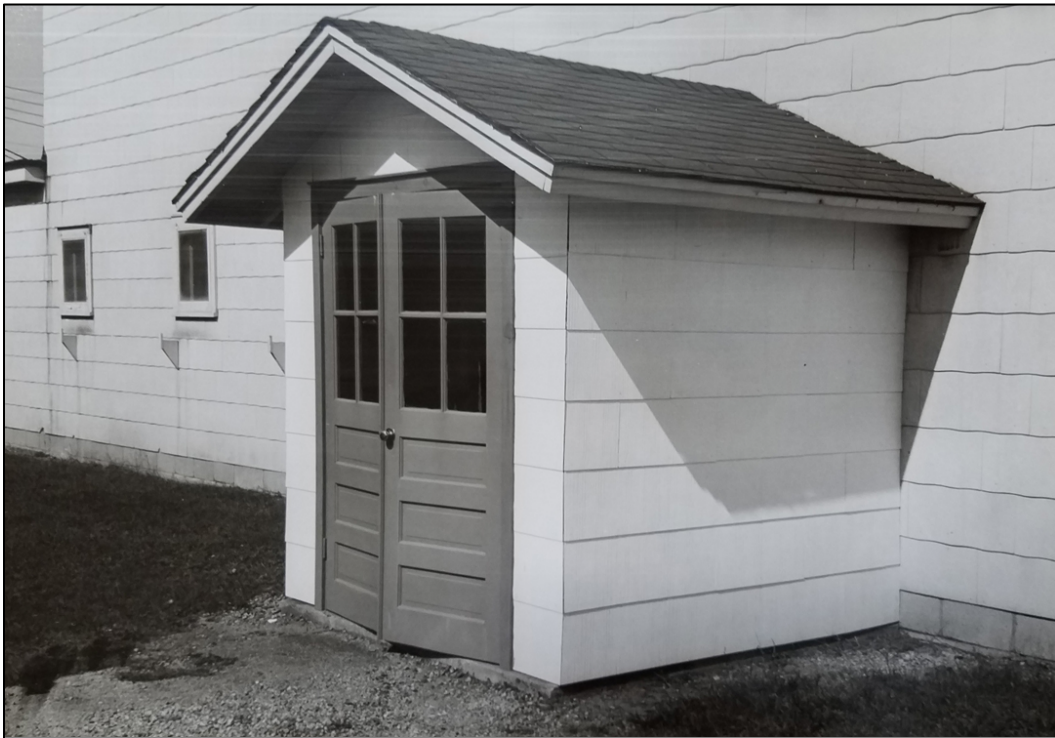
Figure 26. Enclosed side exit to Theater No. 5, Building 2017 (“Post Engineer Project Enclose Side Exits to Theater #5.” Public Domain).
