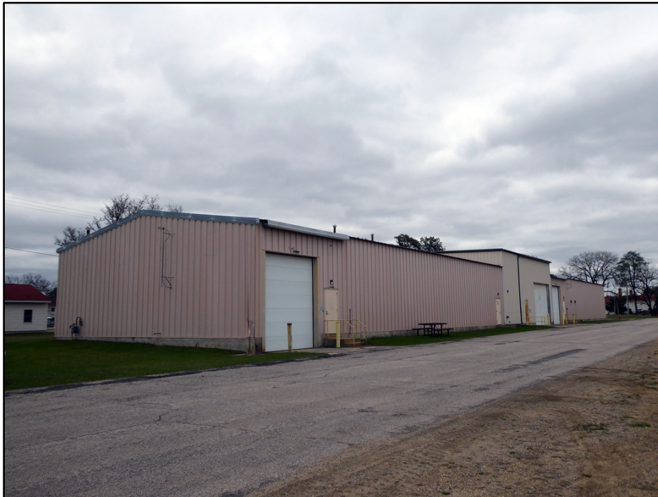
Figure 45. Southwest oblique of Building 1268 (with the original Building 1267 in the foreground, the hyphen addition in the middle, and Building 1268 in the background) (ERDC-CERL 2021).
