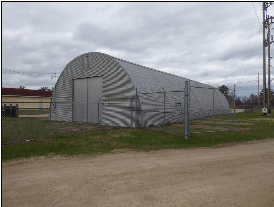
Figure 51. Southeast oblique of Building 2186 (ERDC-CERL 2021).
