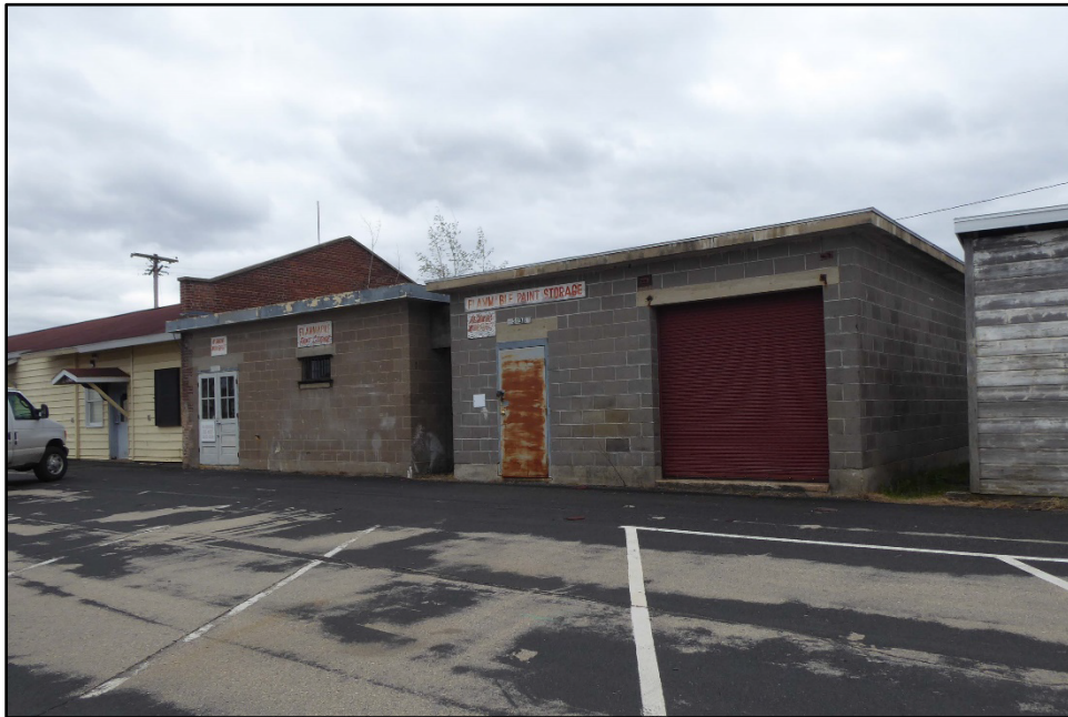
Figure 53. Northwest oblique of Building 2198 ( right ) and Building 2199 ( left ) (ERDC-CERL 2021).
