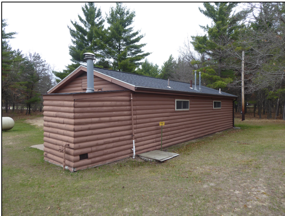
Figure 63. Southeast oblique of Building 8038 (ERDC-CERL 2021).
