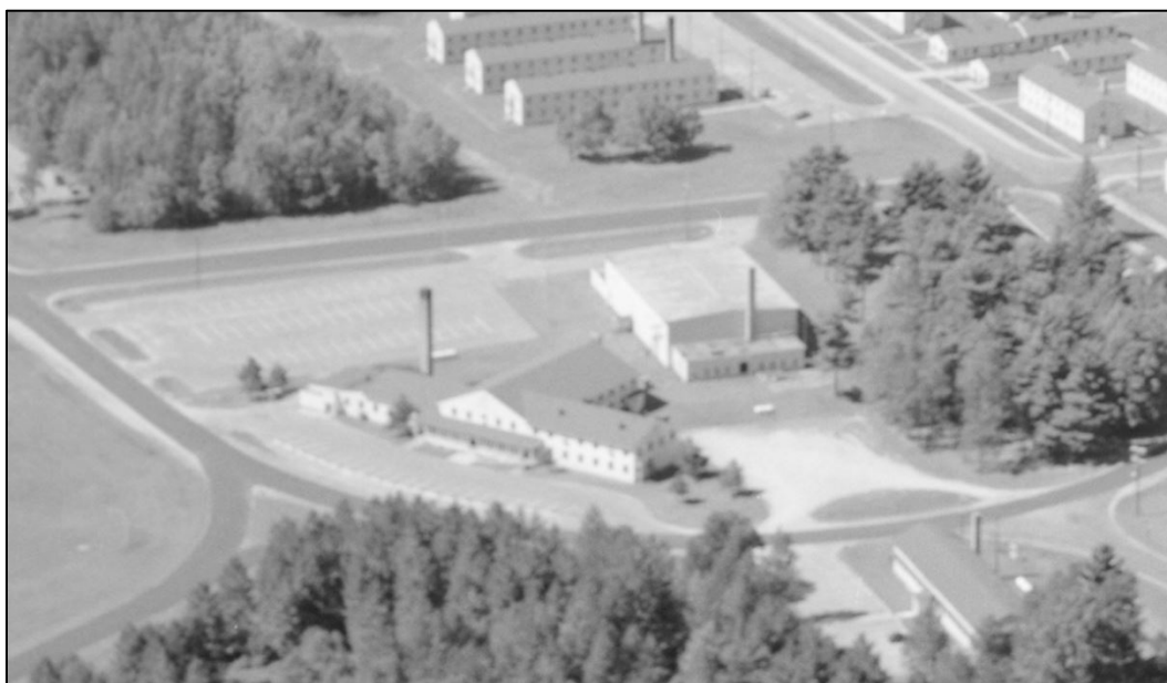
Figure 12. Building 905, Service Club No. 3, after being rebuilt, 1988 (HABS No. WI-308. Public Domain).
