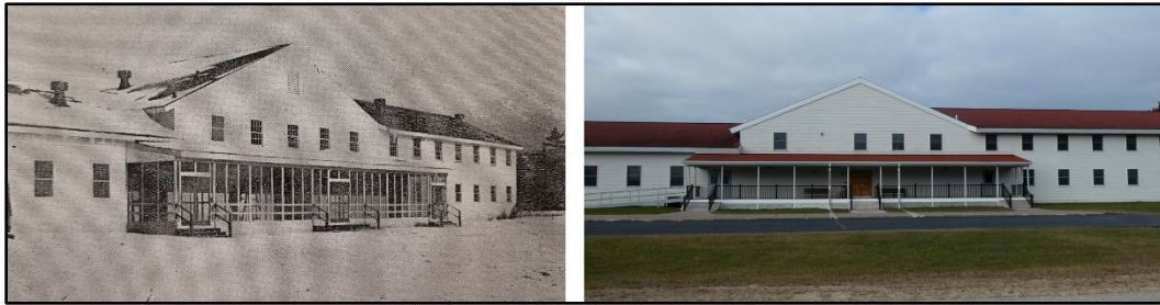
Figure 72. Comparison image of the southeast side of Building 905, Service Club No. 3. Left image from 1953 after the reconstruction of the building due to fire damage, and right image from 2021 ( Left is from La Cross Sunday Tribune , January 11, 1953, and right is from ERDC-CERL. Public Domain).
