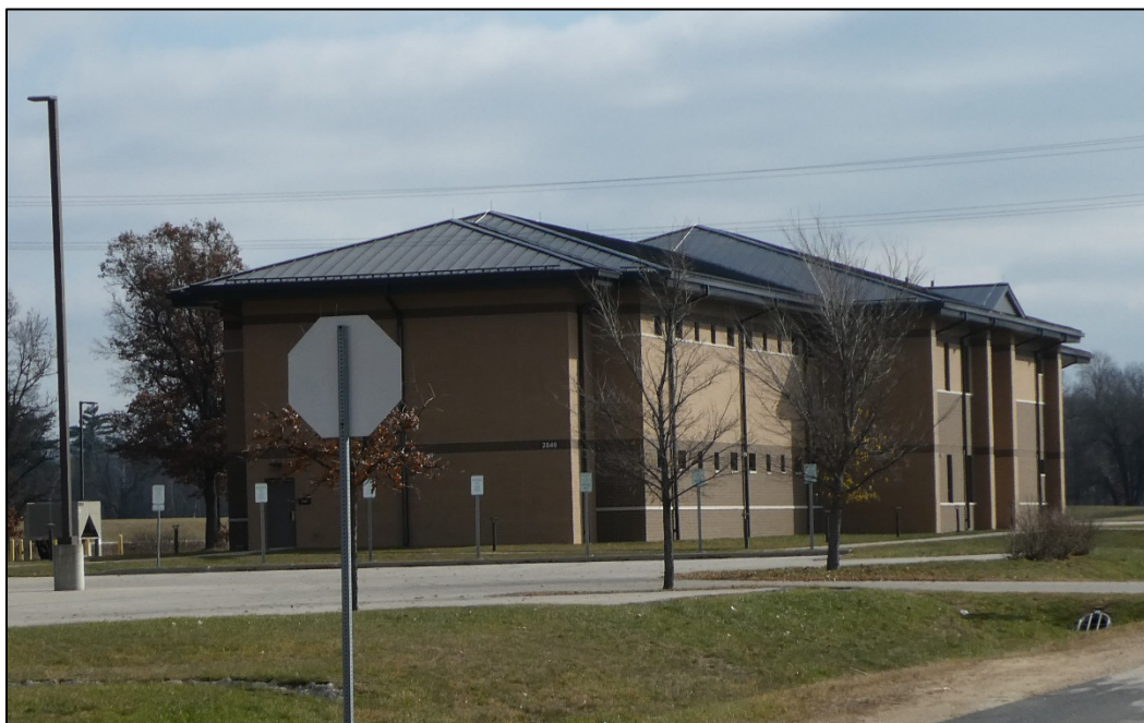
Figure 29. Looking east at Building 2840, a new administration building, 2020 (ERDC-CERL 2020).
