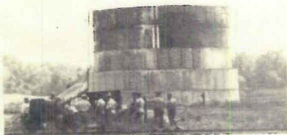
D. Tank after foam had been applied for 8 min.
