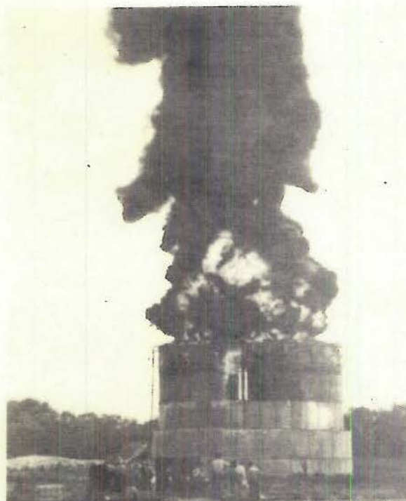
D. About 10 min. after ignition. Flame line visible at bottom of top ring.
