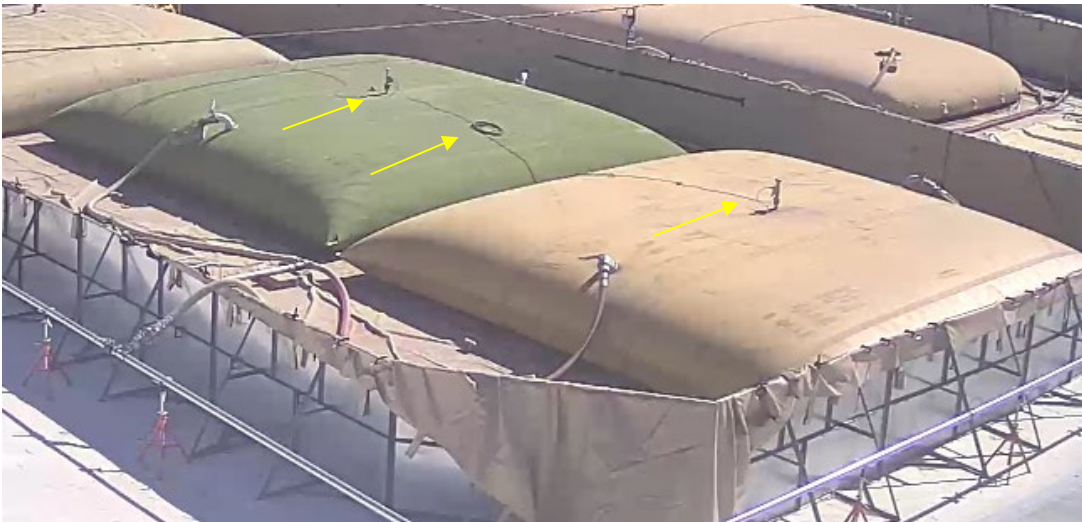
Figure A-14. Top Row (Left to Right)—Varec Cables and Control Boxes, Positive Displacement Flow Meter Used for Varec Virtual Strapping Chart Setup, Single Varec Cable/Probe Assembly Bottom Left—Varec Cables to Probes Installation Through CFT Vent Pipes (Yellow Arrows)
