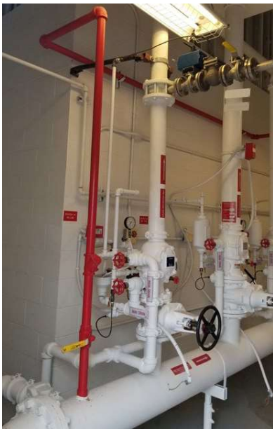
Figure 1. Foam/Water Deluge Riser (left) and Bladder Tank (right)
