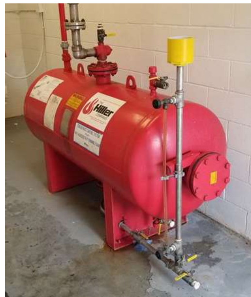
Figure 1. Foam/Water Deluge Riser (left) and Bladder Tank (right)
