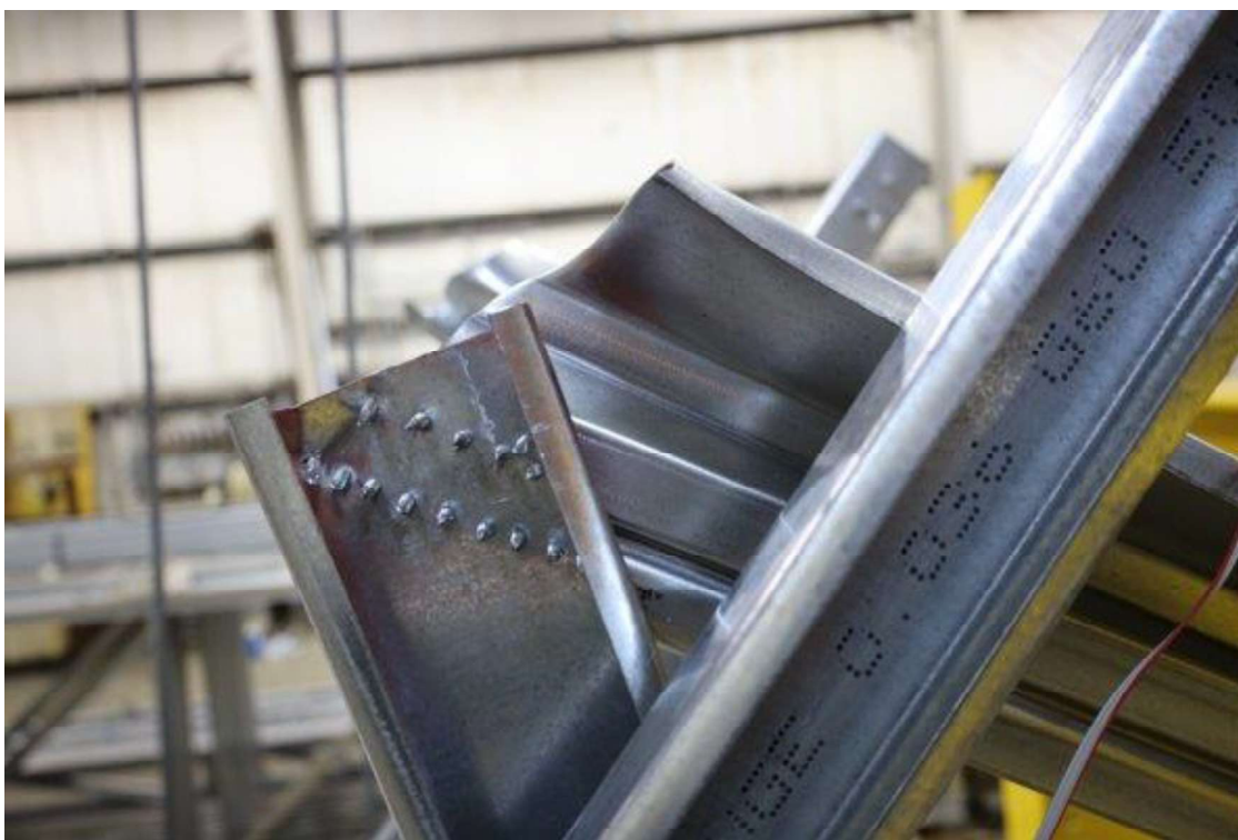
Figure 42: Cutting of Tension Chord Section (AG48-D57)
