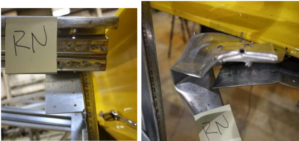
Figure 27: Bearing Connection Failure at RN (AG36-D35)
