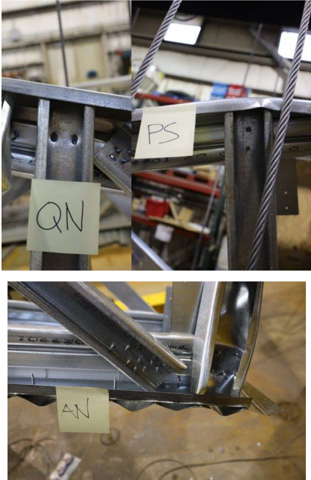
Figure 26: Partial Failures in Web Element Connections (AG36-D35)
