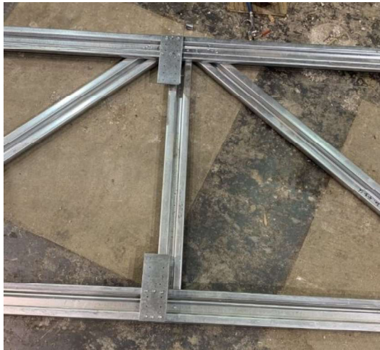
Figure 15: Swiftclip Bracing Angles
