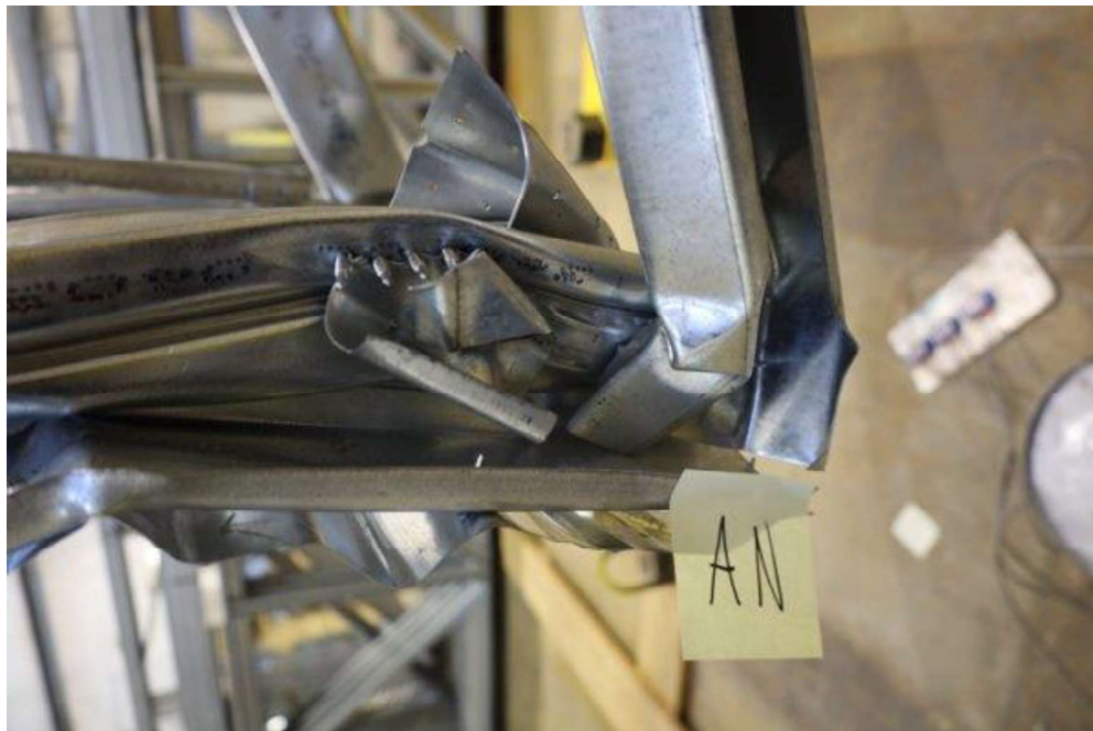
Figure 31: Rupture of Diagonal at Joint AN (AG48-D35)
