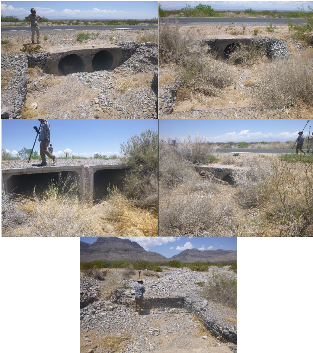
Figure 5. Culverts 2–5 ( top left, clockwise ). Typical gabion basket drop structure ( bottom ).
