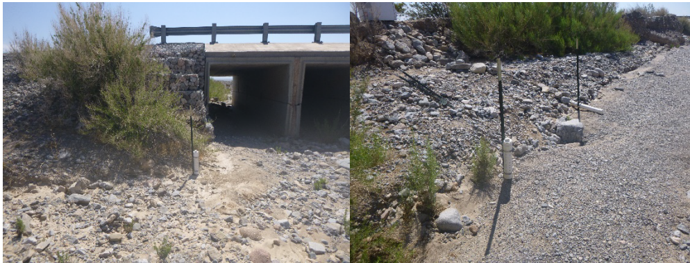
Figure 14. Typical HOBO installations.
