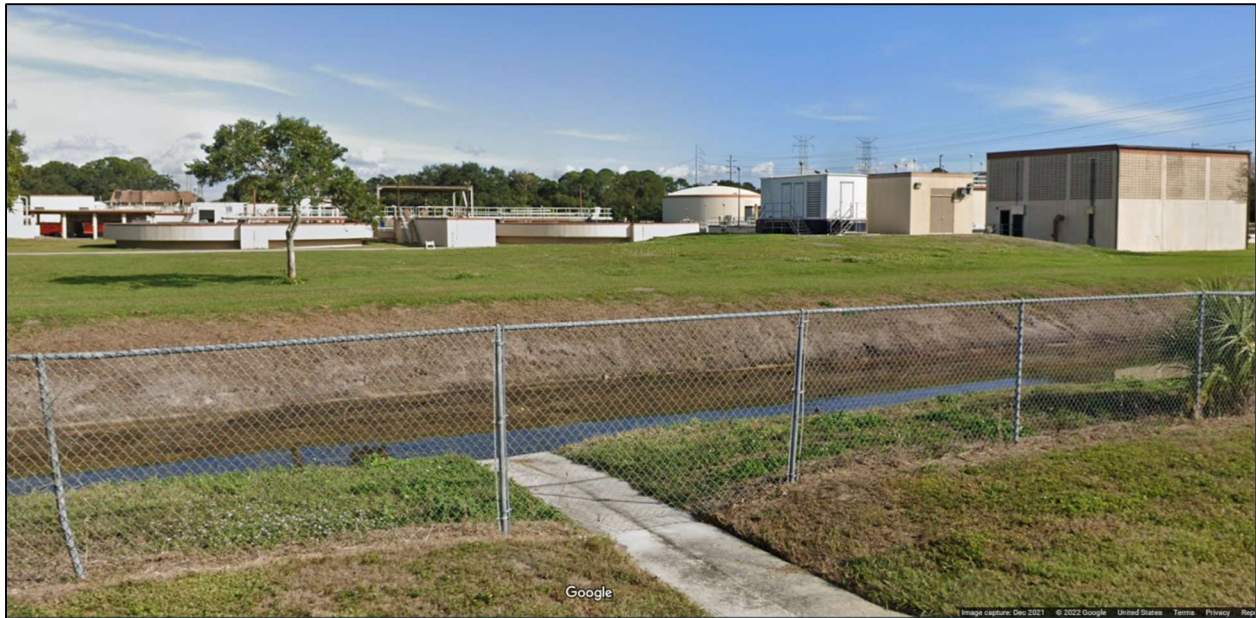
Figure 1: Street view of the Oldsmar Water Treatment Plant, Google Maps
