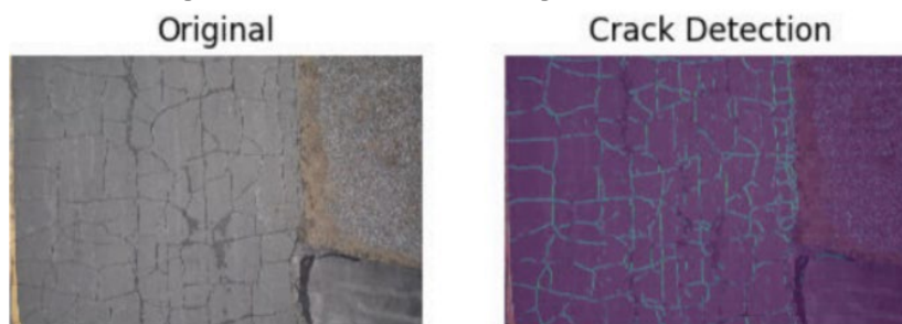
Figure 14. Example of full image crack detection.
