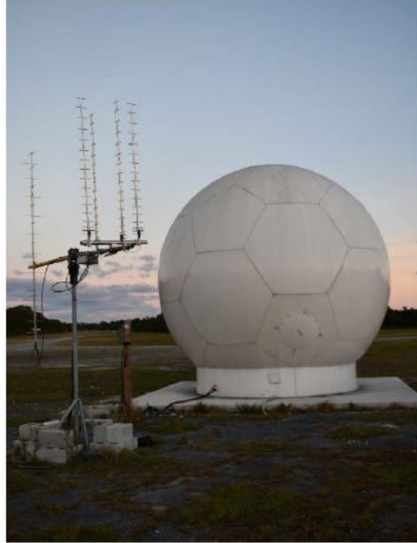
Figure 11. MLB ground station, UHF Yagi and S-band dish/radome. Source: [4].
