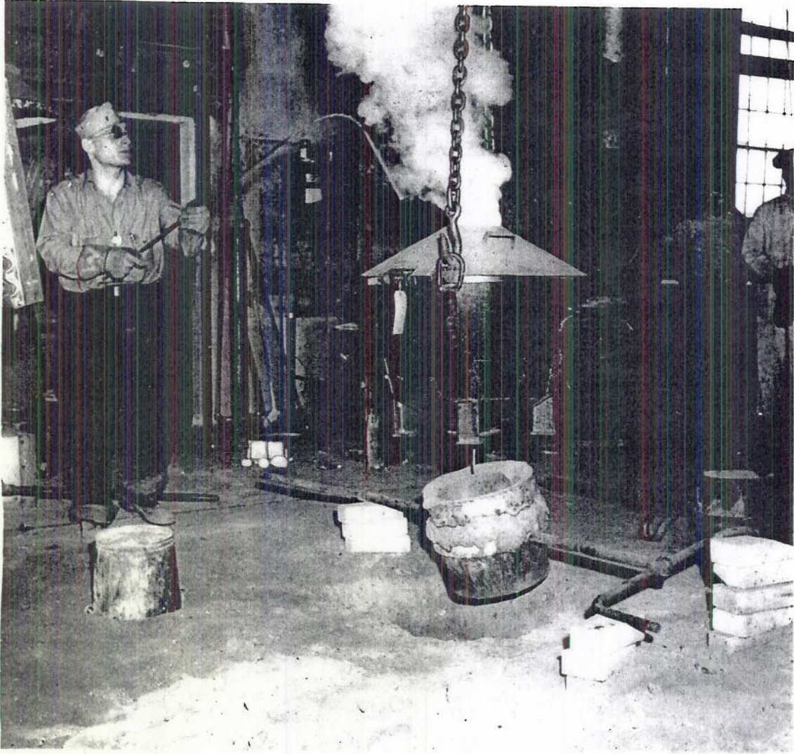
BEGINNING OF THERMIT REACTION
