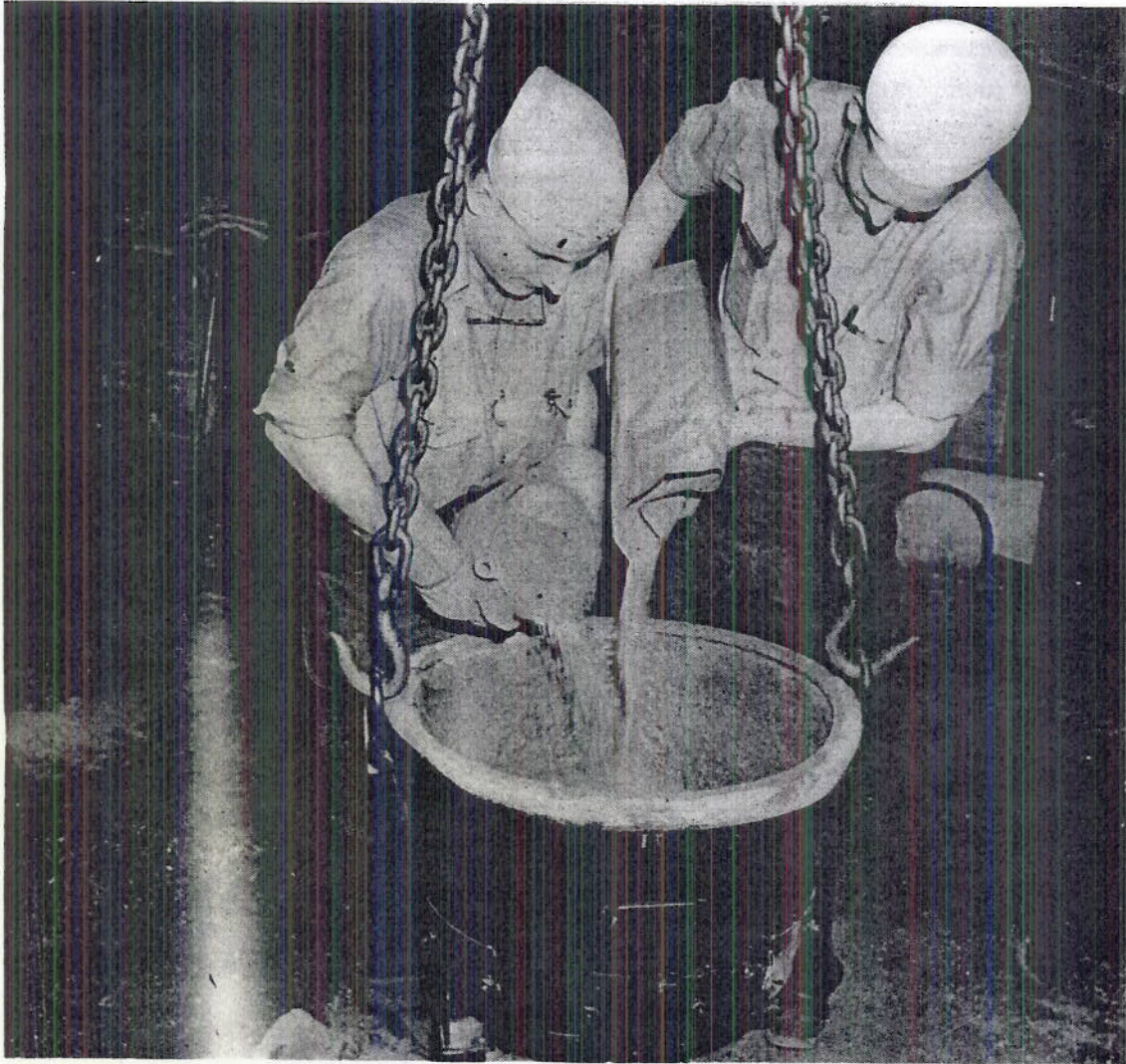
CHARGING STEEL PUNCHINGS AND THERMIT TO #8N (ROUND BOTTOM) CRUCIBLE
